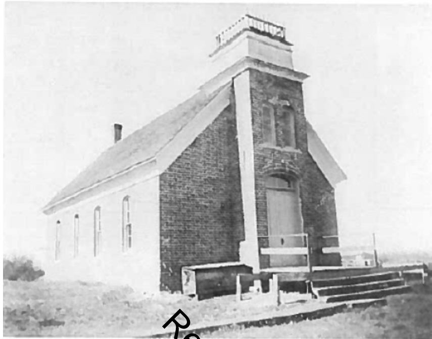
Figure 6: First Presbyterian Church. The Gibbon Baptist Church met here following its reorganization until their building was completed in 1890. ( Fair of the Generations , Gibbon Baptist Church, 2013: 14)
