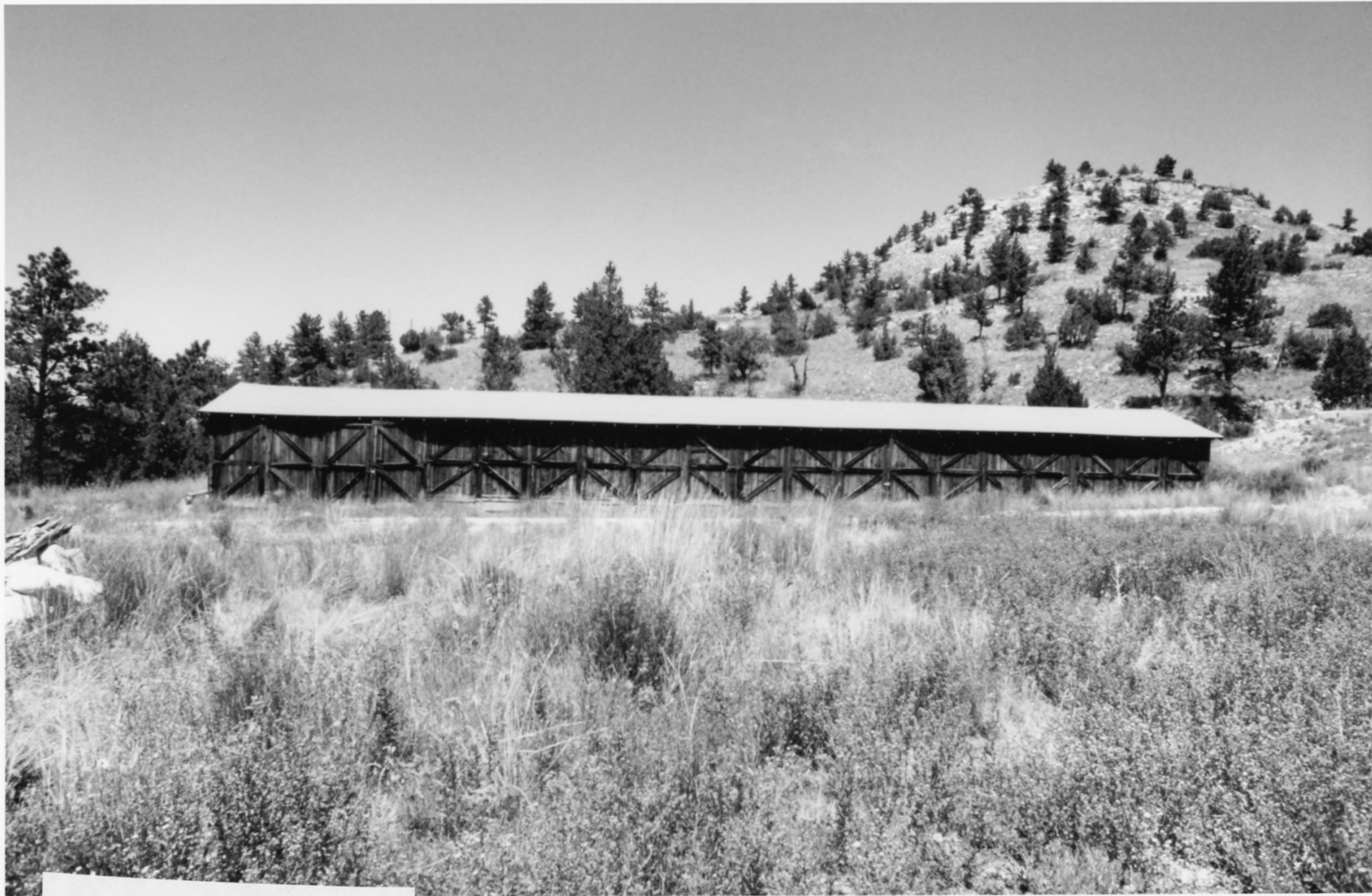
LAKE GUERNSEY STATE PARK Guernsey vicinity, Platte County, Wyoming Site of CCC Camp Photo: Ethan Carr, 1994
