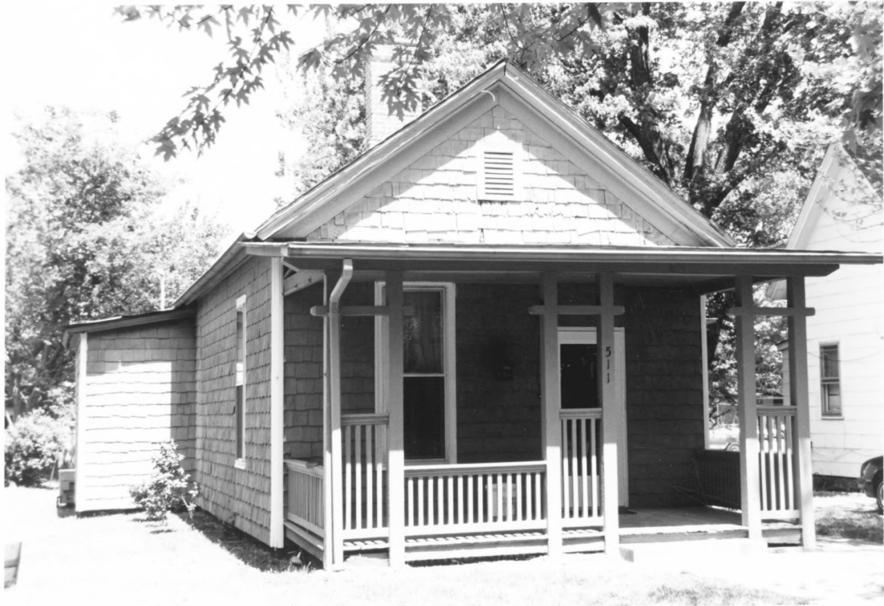
A) Green House, Alves Historic District, Henderson, KY
