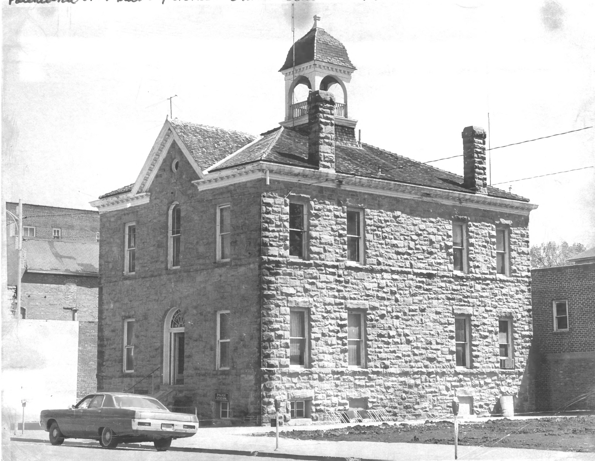
Parkersburg City Hall - Former OS&A course house
