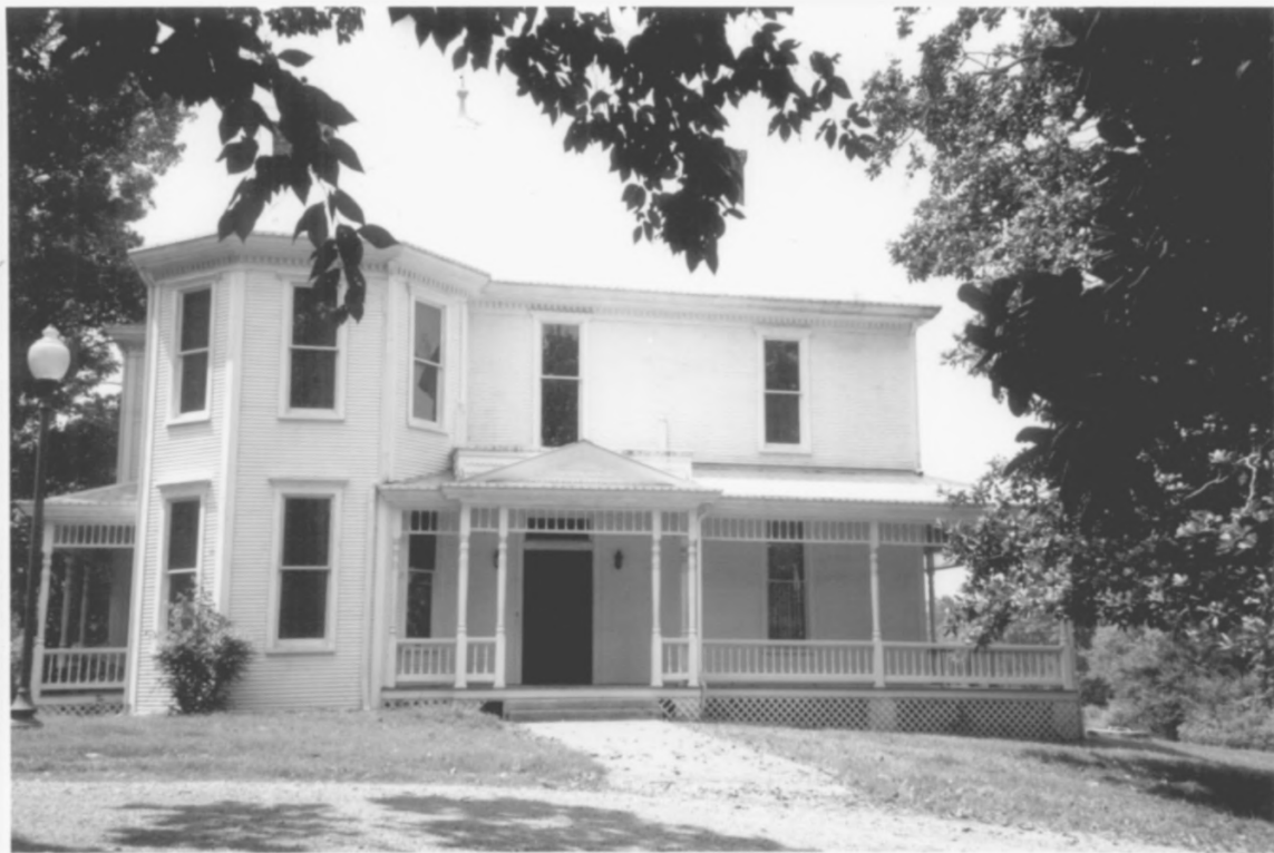
Riverside. Farm house Bedford County TN
