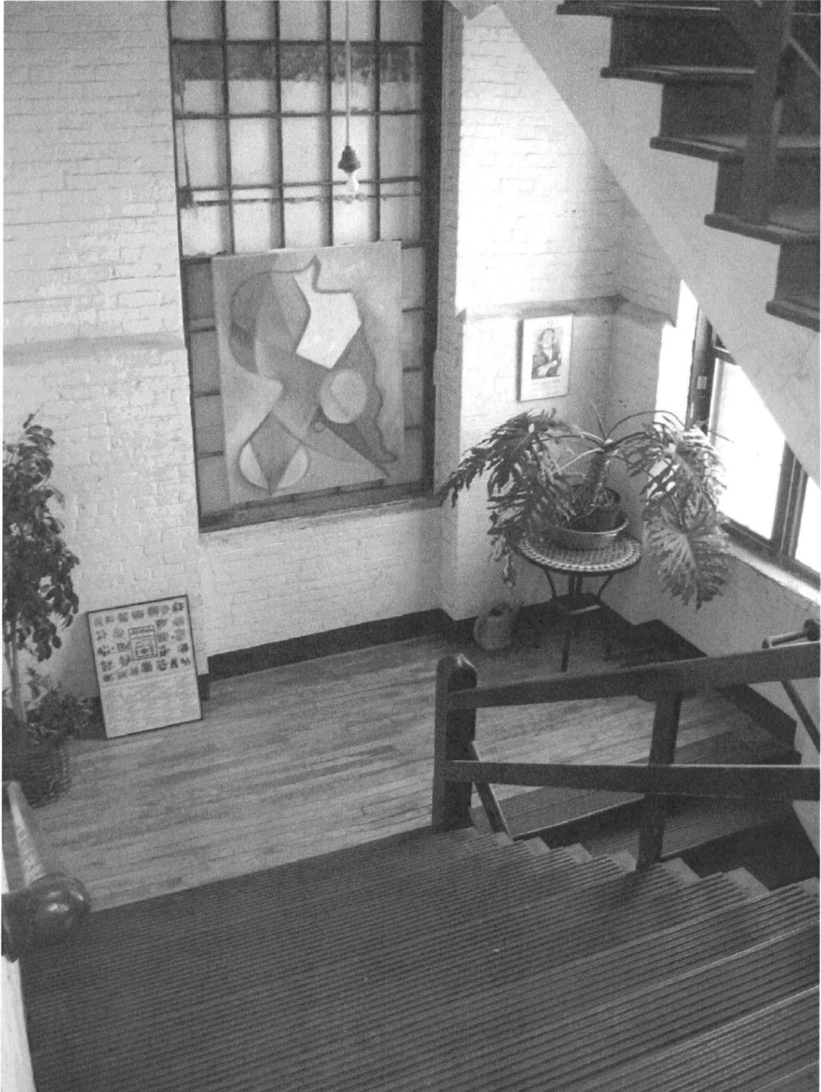
Interior of south stairwell, showing detail of landing between the first and second floors.
