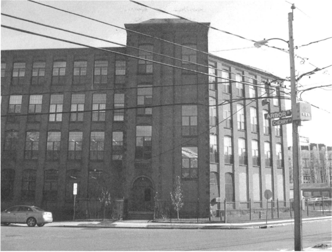
West and southwest elevations from Arbor Street, showing south stair tower and the ell attached to the south elevation.
