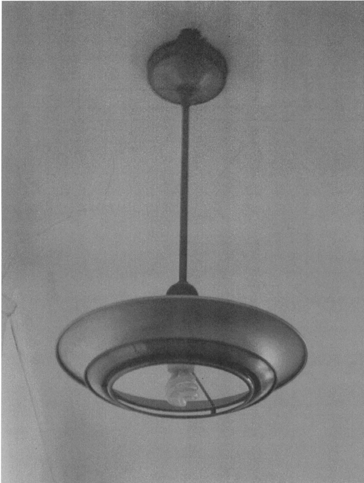
Interior of fourth floor hallway, showing detail of light fixture. Camera facing east. Photograph 21 of 21
