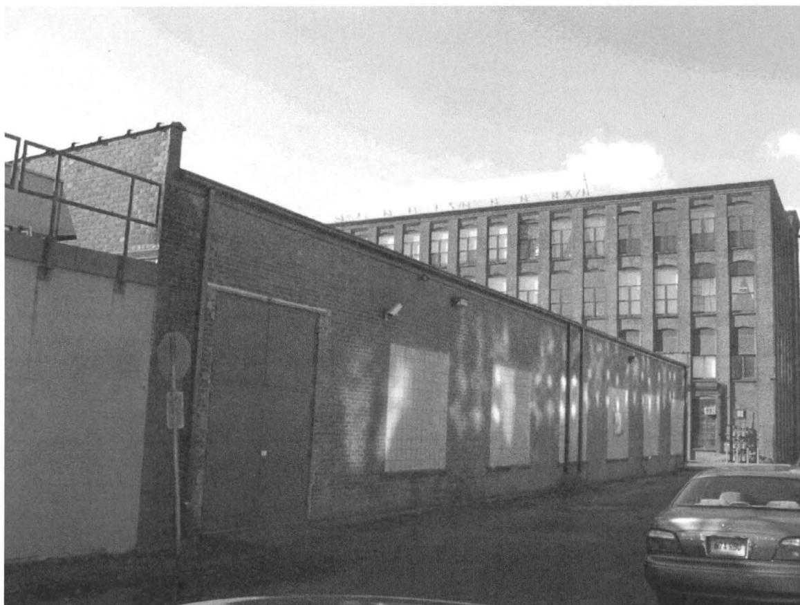
North elevation facing the Gray Pay Telephone Station Company, showing rear of main factory building and c. 1923 addition for cafeteria. Camera facing southwest. Photograph 11 of 21
