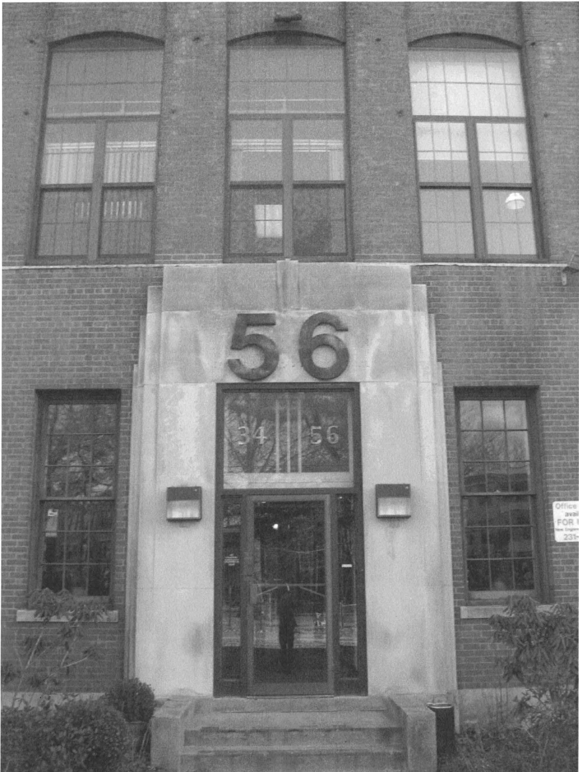
Detail of central entryway, showing molded concrete details and glass doors. Camera facing east. Photograph 5 of 21
