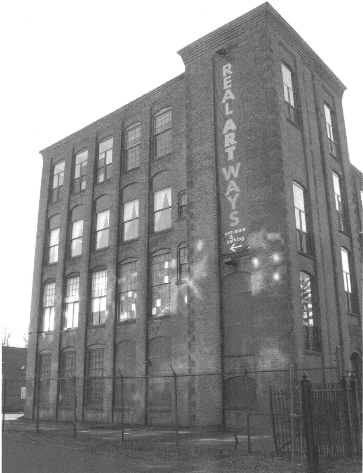
North elevation, facing Gray Pay Telephone Station Company, showing end of main factory, north stair tower, and window details.
