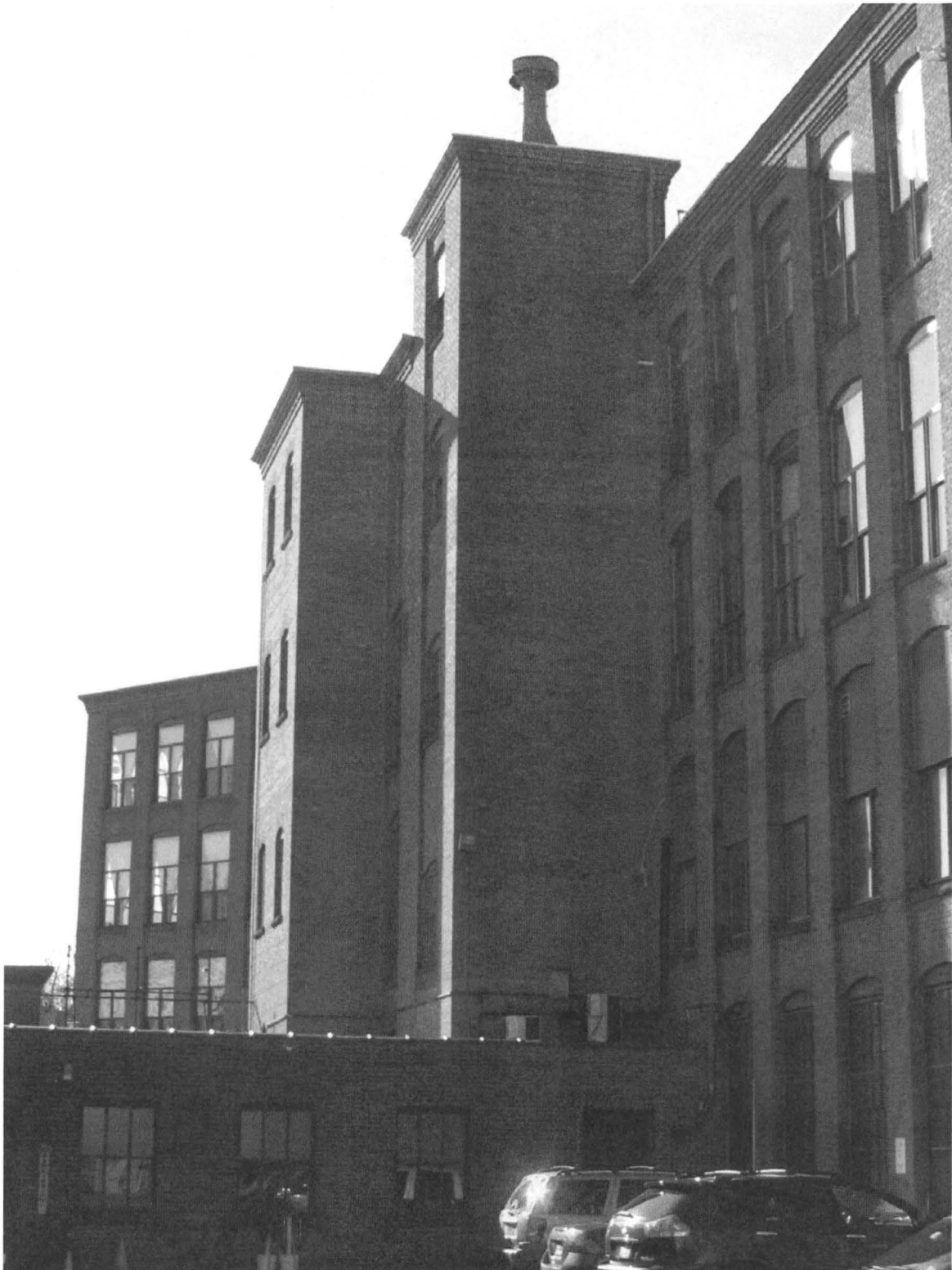
East elevation facing the New York, New Haven, and Hartford Railroad; showing main factory building, elevator, and restroom shafts as well as the receiving room, and northeast elevation of the ell.
