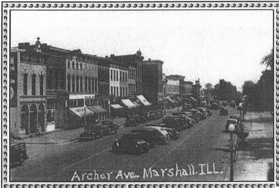
Image 6: Historic photo circa 1940 showing the north side of Archer Ave and the 500- 600 blocks; photo is facing NE.
