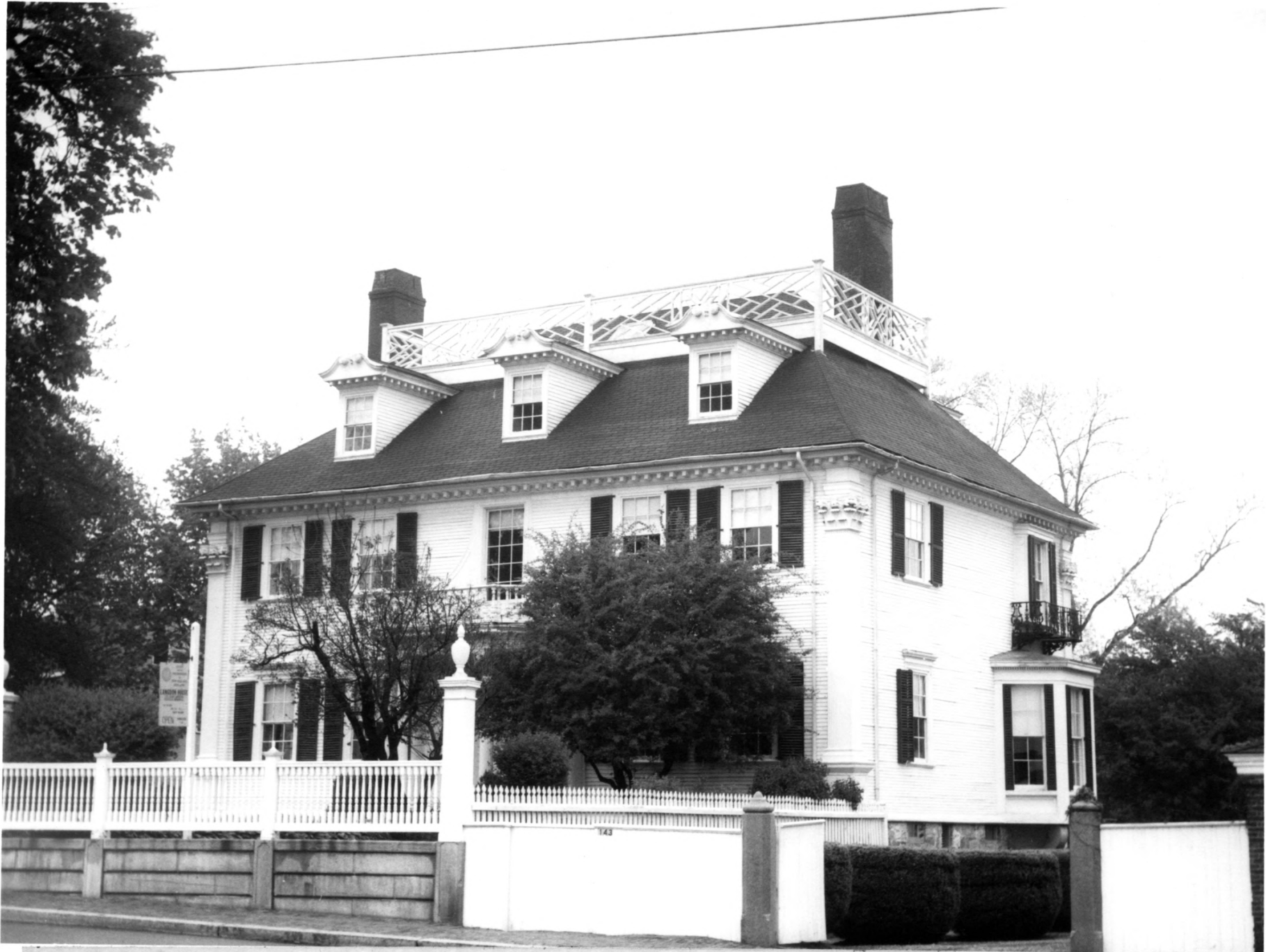
Governor John Langdon Mansion, Portsmouth, New Hampshire
