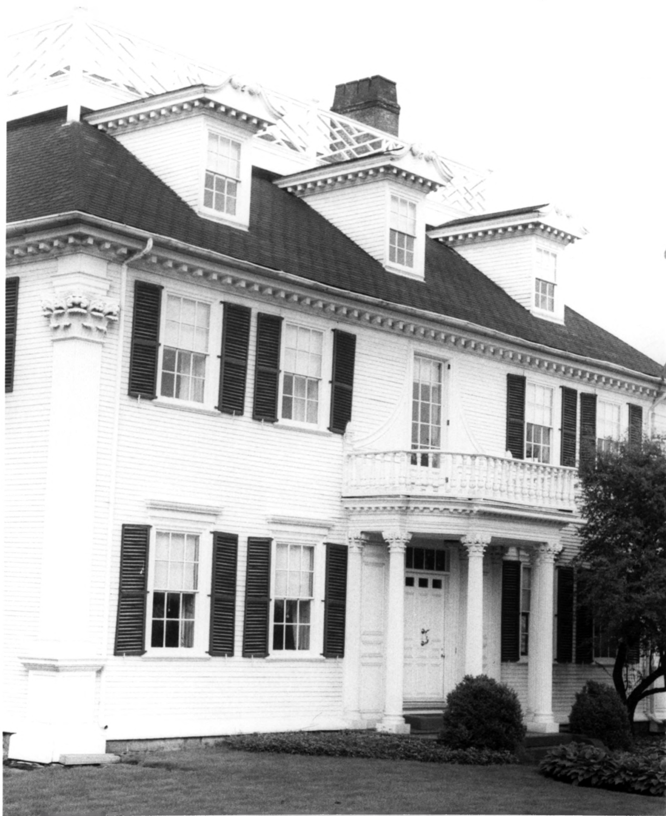
Governor John Langdon Mansion, Portsmouth, New Hampshire
