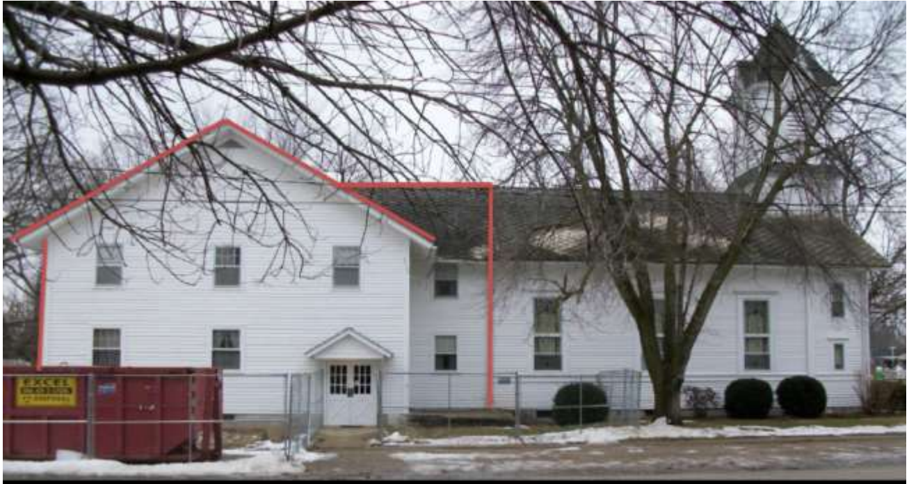
West elevation of the Bristol Congregational Church, showing the 1953 extension and addition (outlined in orange).
