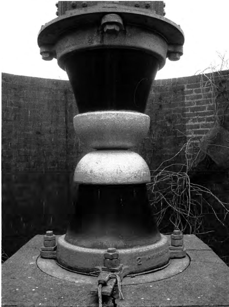
Figure 9. The two Lapp insulators on which the entire tower antenna rests.
