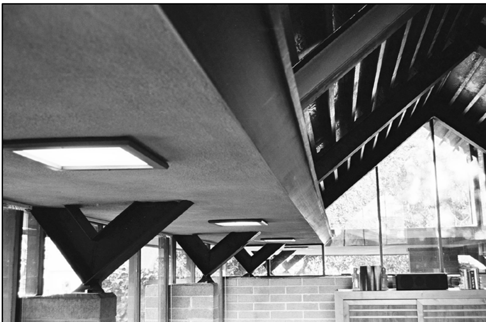
Figure F. W-shaped rigid steel bents resting atop concrete masonry piers support peaked gable roof, roof overhang, and soffit, camera facing northwest, 2000. Graeme Whifler, Photographer.
