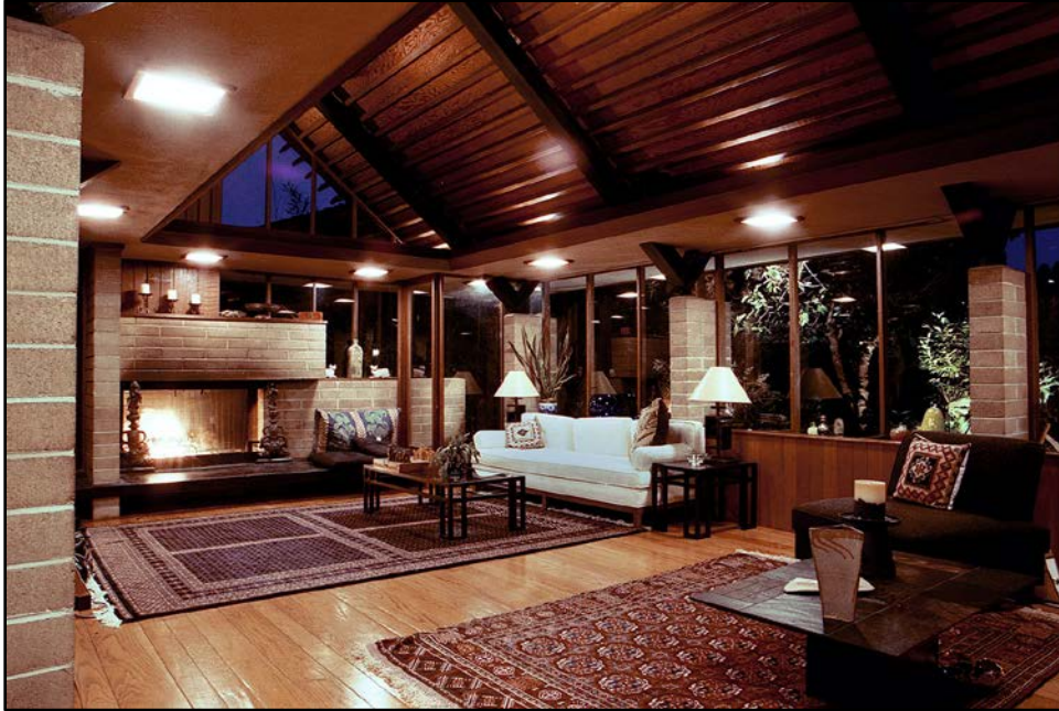
Figure F. W-shaped rigid steel bents resting atop concrete masonry piers support peaked gable roof, roof overhang, and soffit, camera facing northwest, 2000. Graeme Whifler, Photographer.
