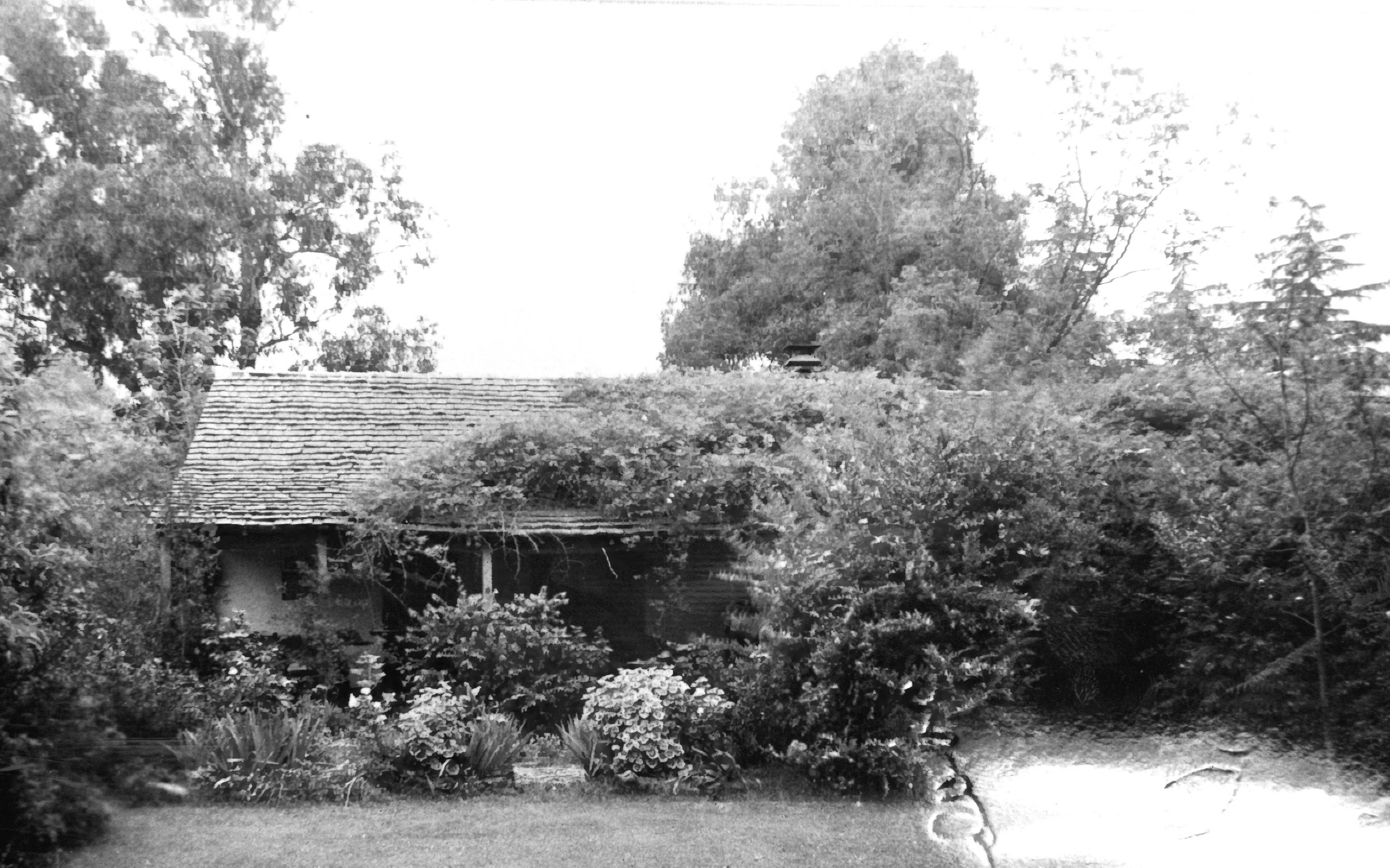
Catalina Verdugo Adobe Glendale's oldest home 50.
