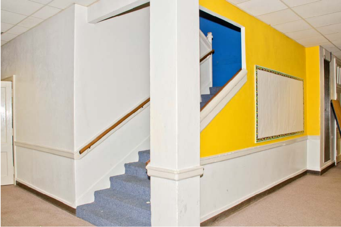
17 of 25: First floor interior, view southeast
