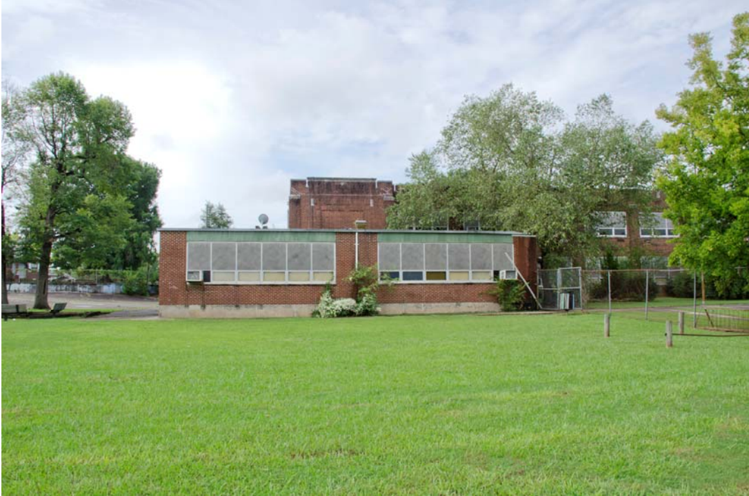
5 of 25: North (Primary) Elevation, view south
