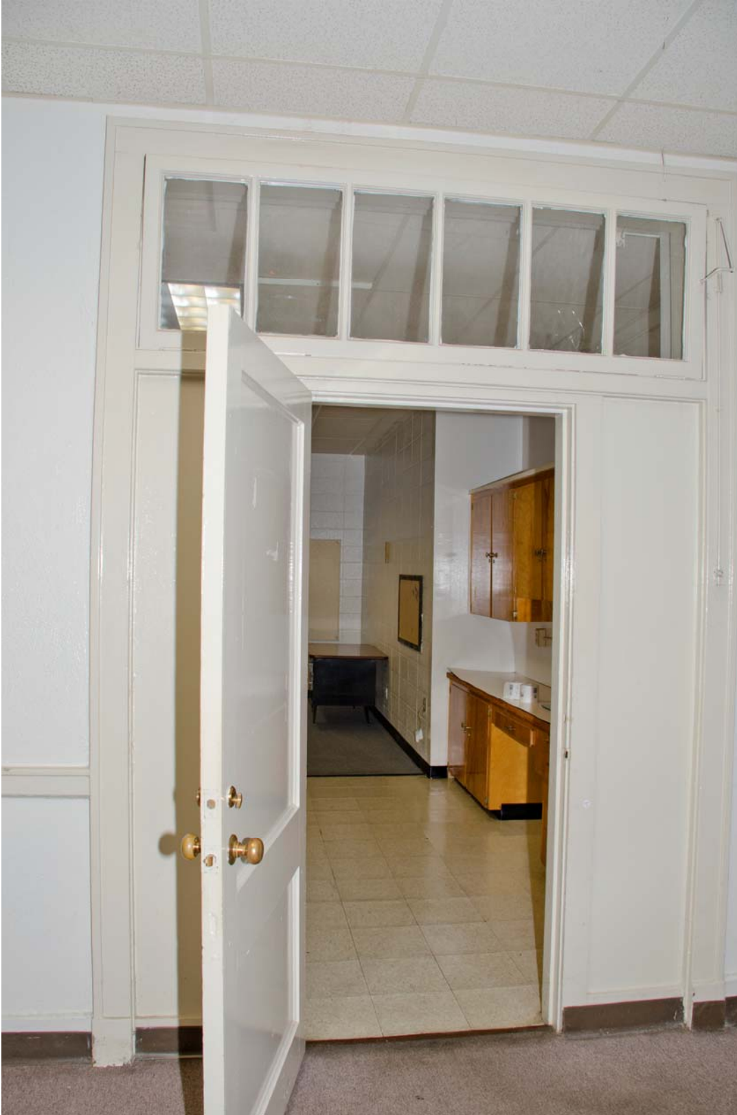
16 of 25: First floor interior, view south
