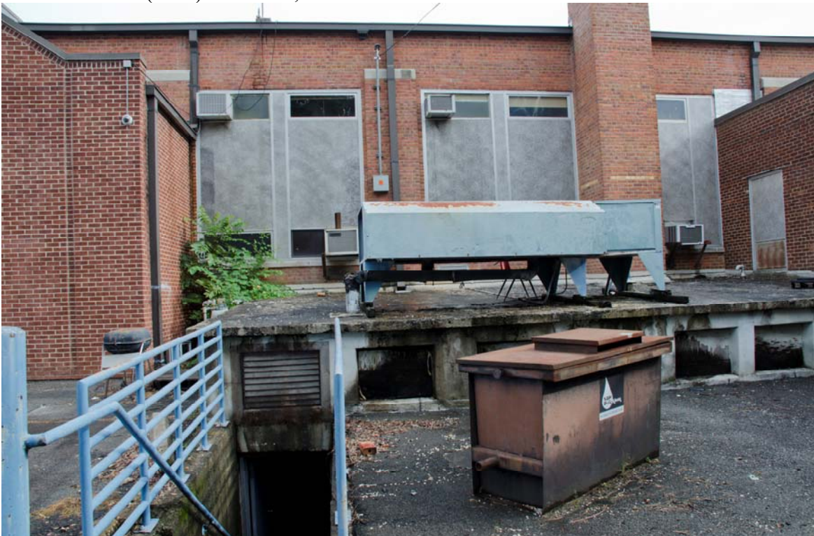
12 of 25: South (Rear) Elevation, view north
