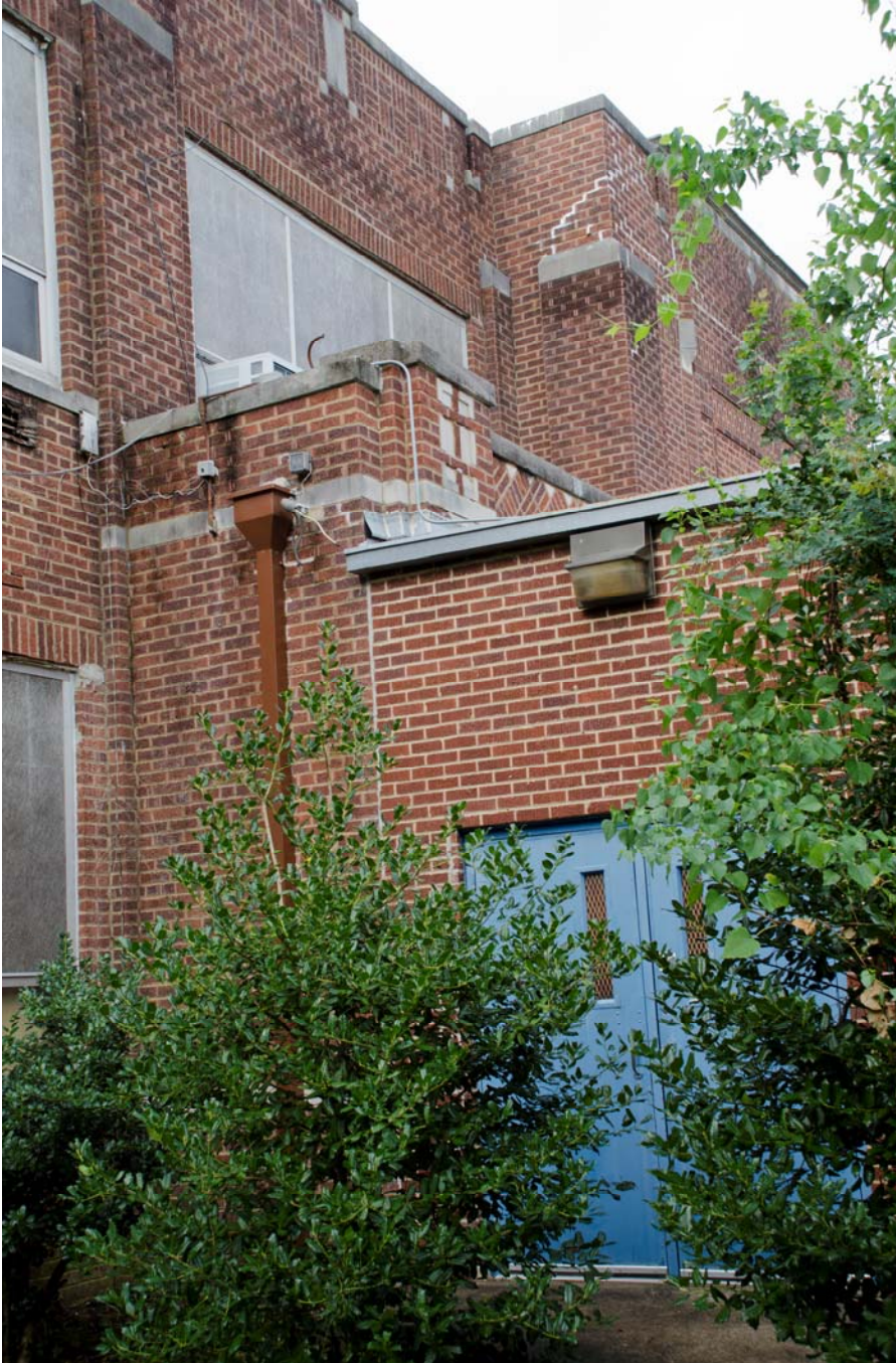
6 of 25: North (Primary) Elevation detail, view southwest
