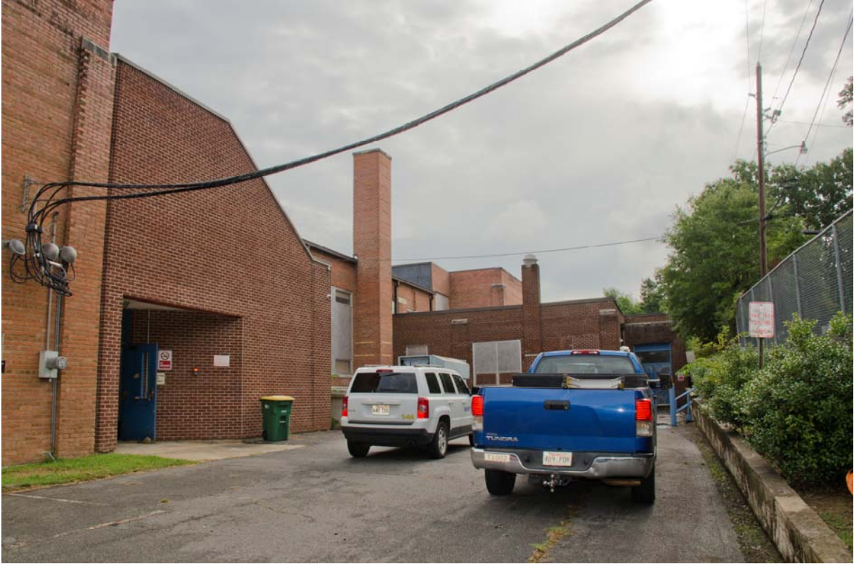
11 of 25: South (Rear) Elevation, view northeast
