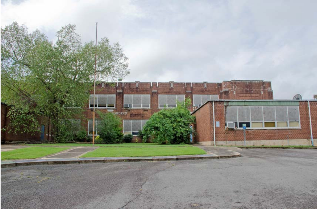
1 of 25: North (Primary) Elevation, view south
