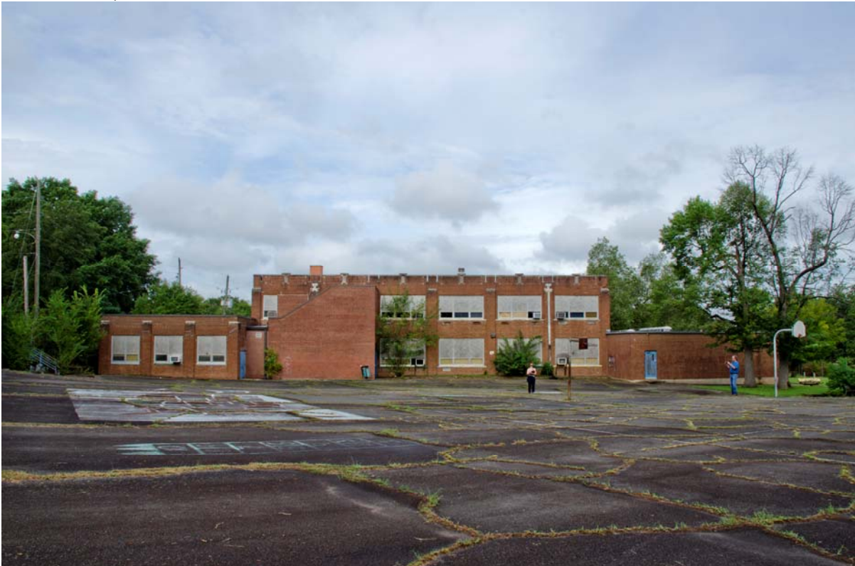
10 of 25: East elevation, view west
