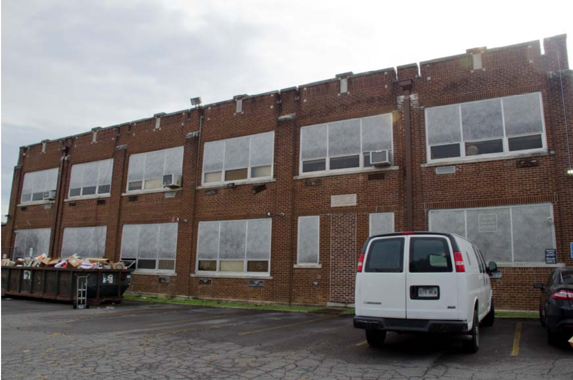
7 of 25: West Elevation, view east
