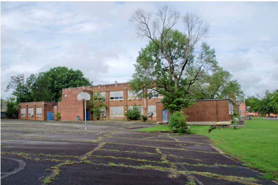
8 of 25: East Elevation, view west
