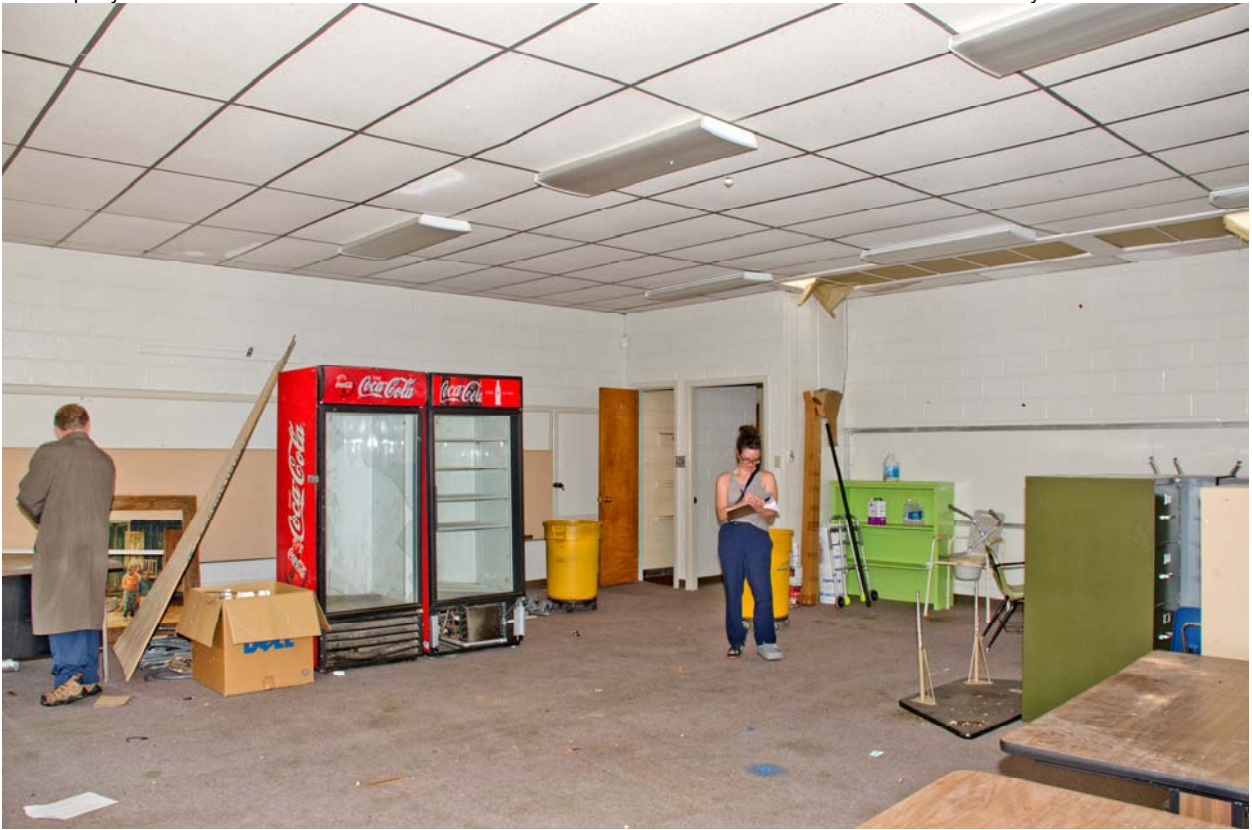
19 of 25: First floor interior, view south
