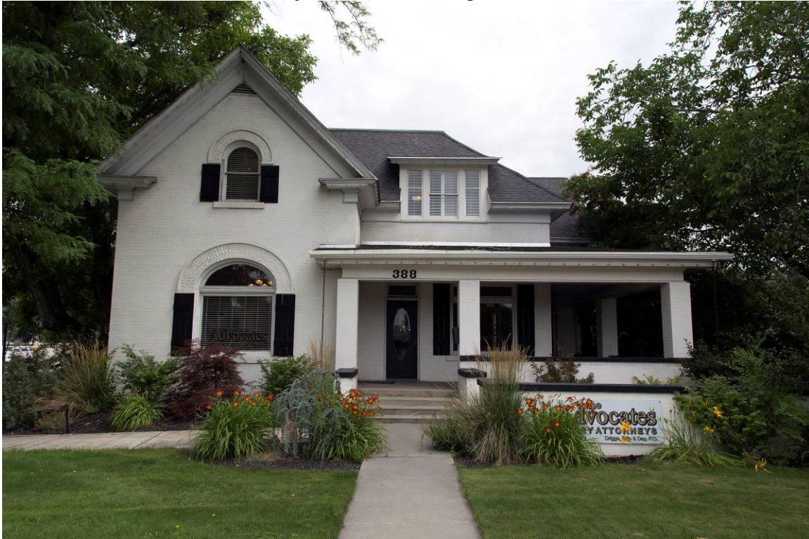
1 of 16. View of south (front) façade. Camera facing north
