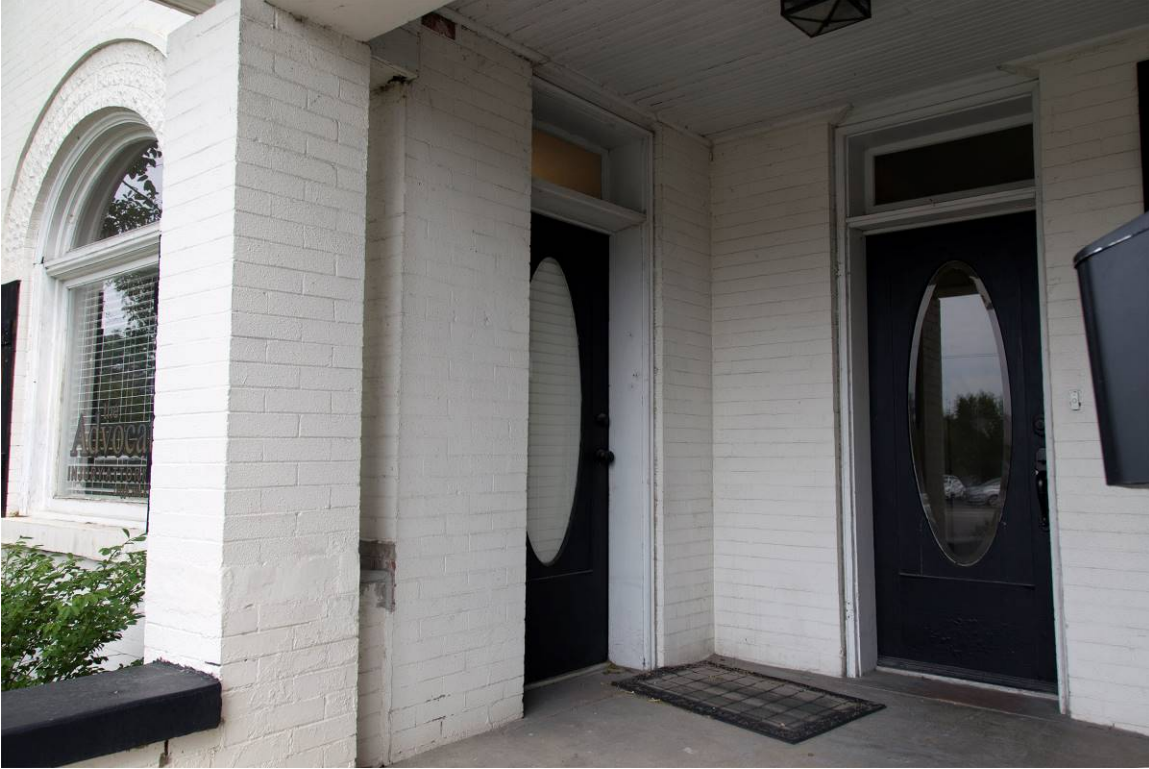
9 of 16. Projecting gable window and door detail. Camera facing northwest.
