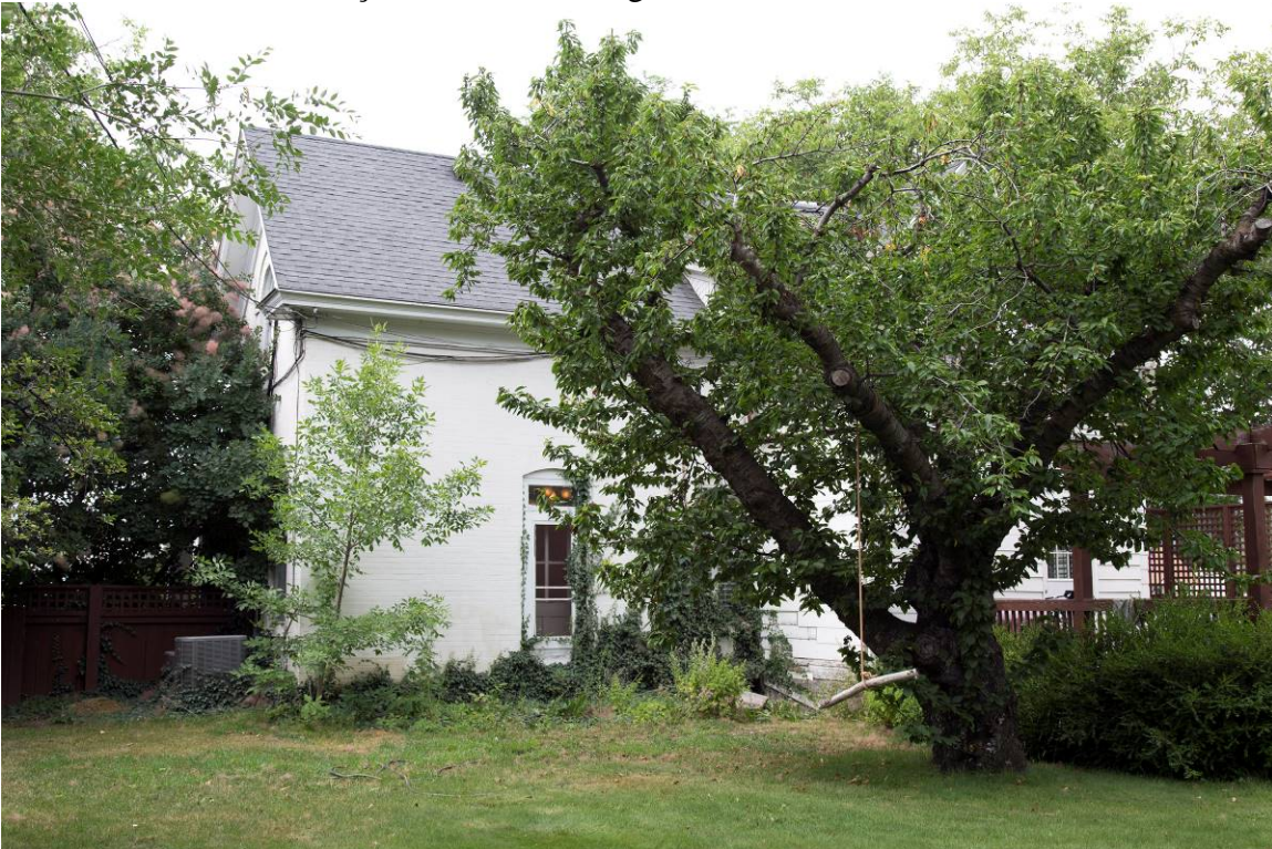
4 of 16. View of north façade. Camera facing south.
