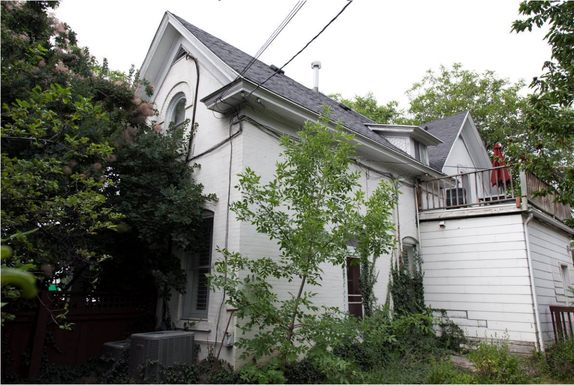
3 of 16. View of north and east façades. Camera facing southwest.
