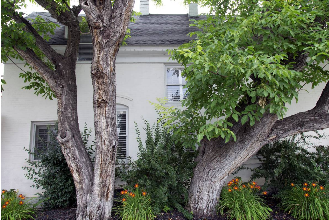
7 of 16. View of west façade. Camera facing east.
