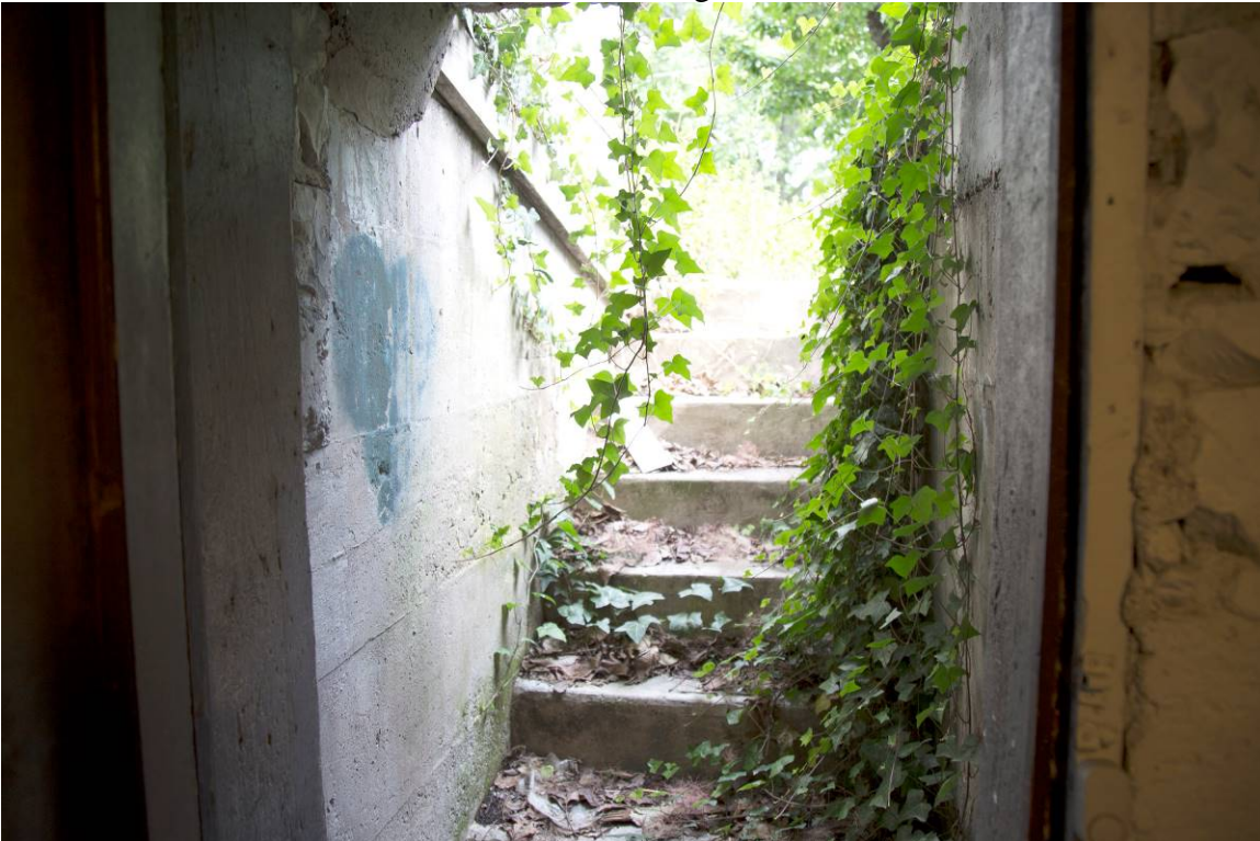
12 of 16. Back stair addition detail. Camera facing north.
