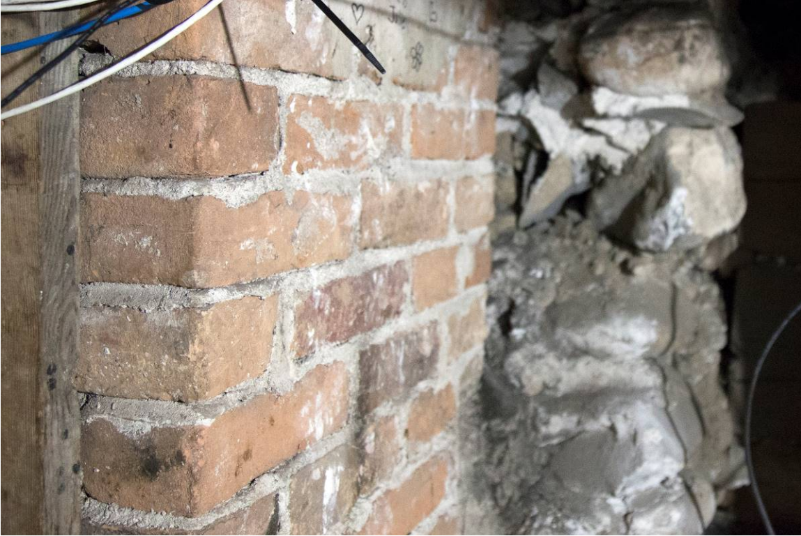
11 of 16. Original brick and foundation stone detail (basement). Camera facing east.
