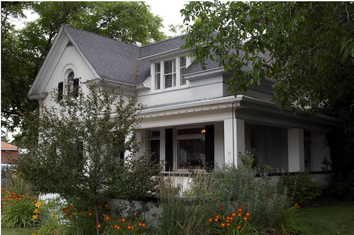
2 of 16. View of south and east facades. Camera facing northwest.
