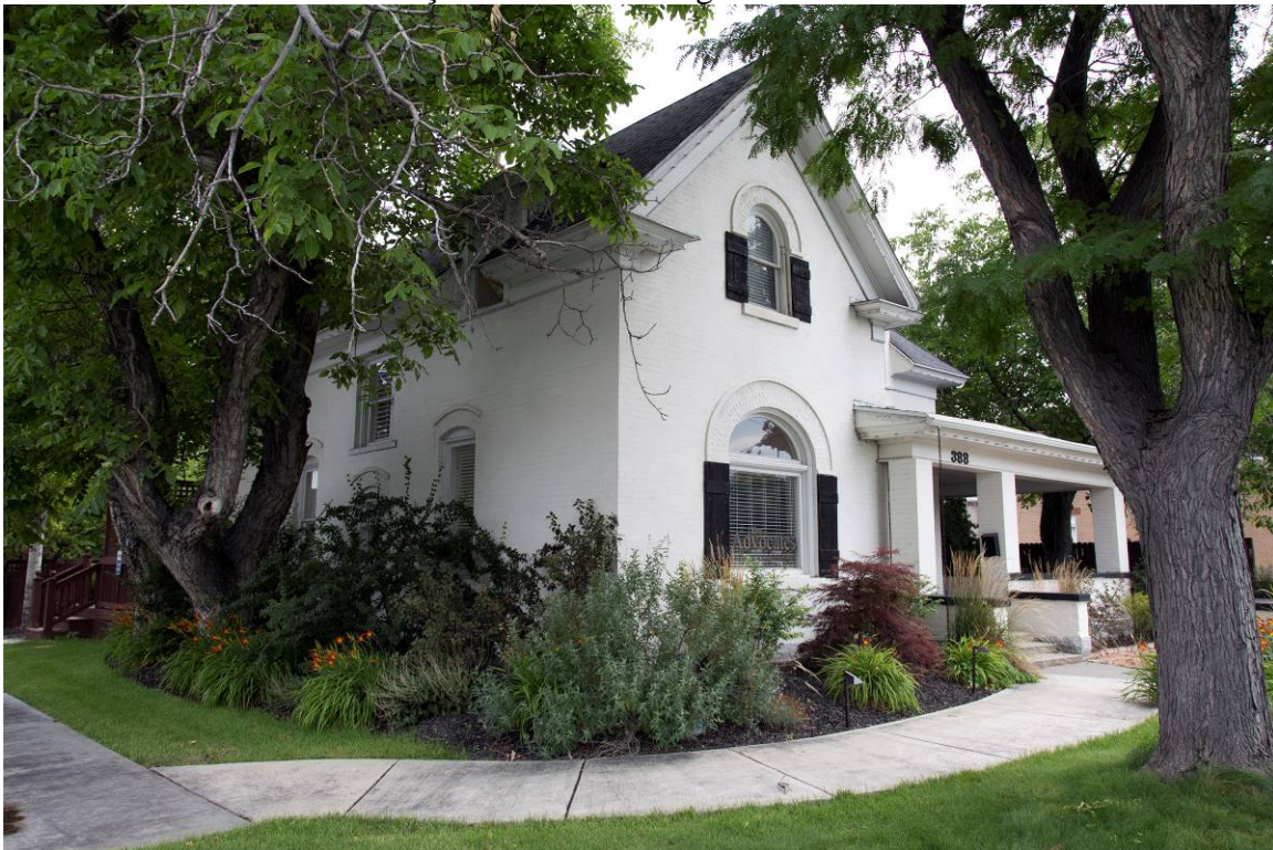
8 of 16. View of southwest façade. Camera facing northeast.
