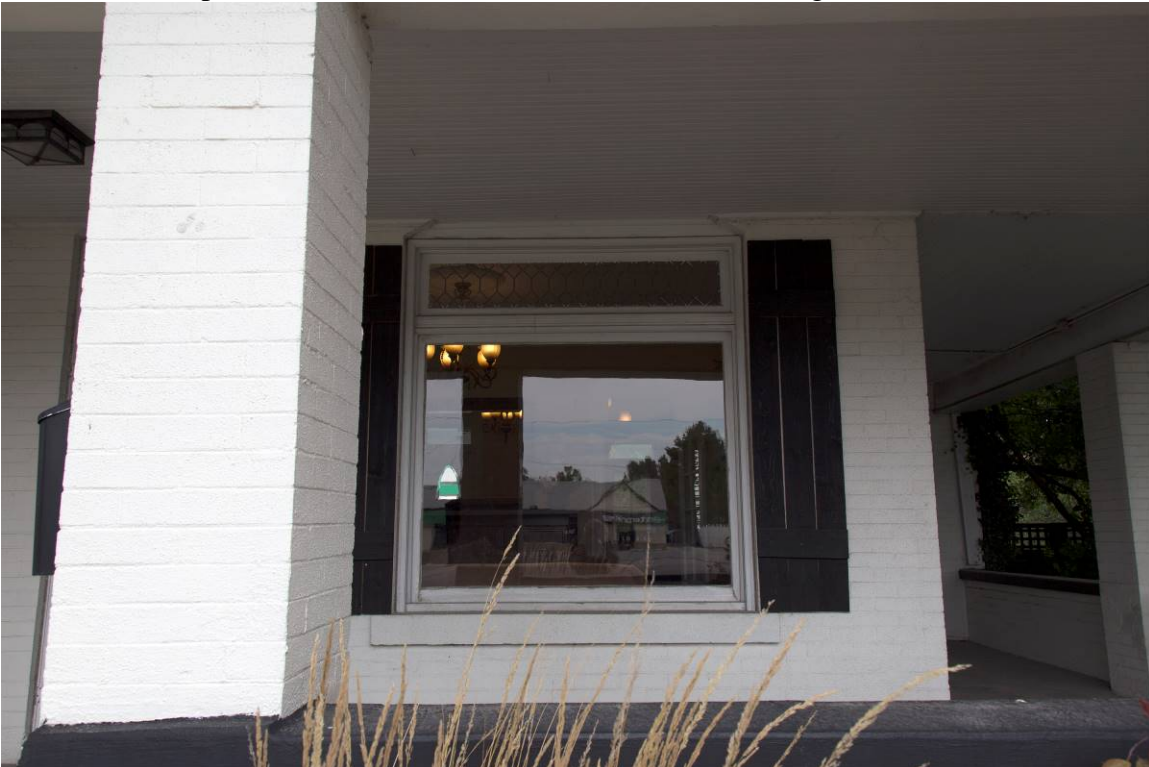
10 of 16. Front porch column and window detail. Camera facing north.
