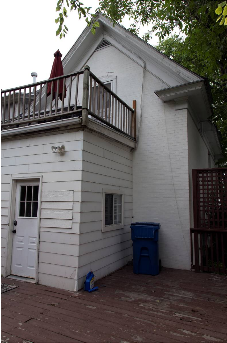
6 of 16. View of northwest façade. Camera facing southeast.
