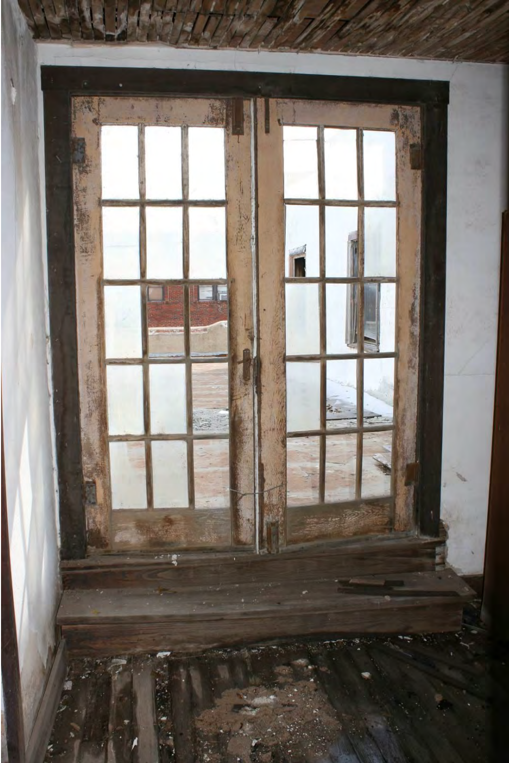
Photo 13: Second floor; double doors opening onto the east bay. Camera facing south.
