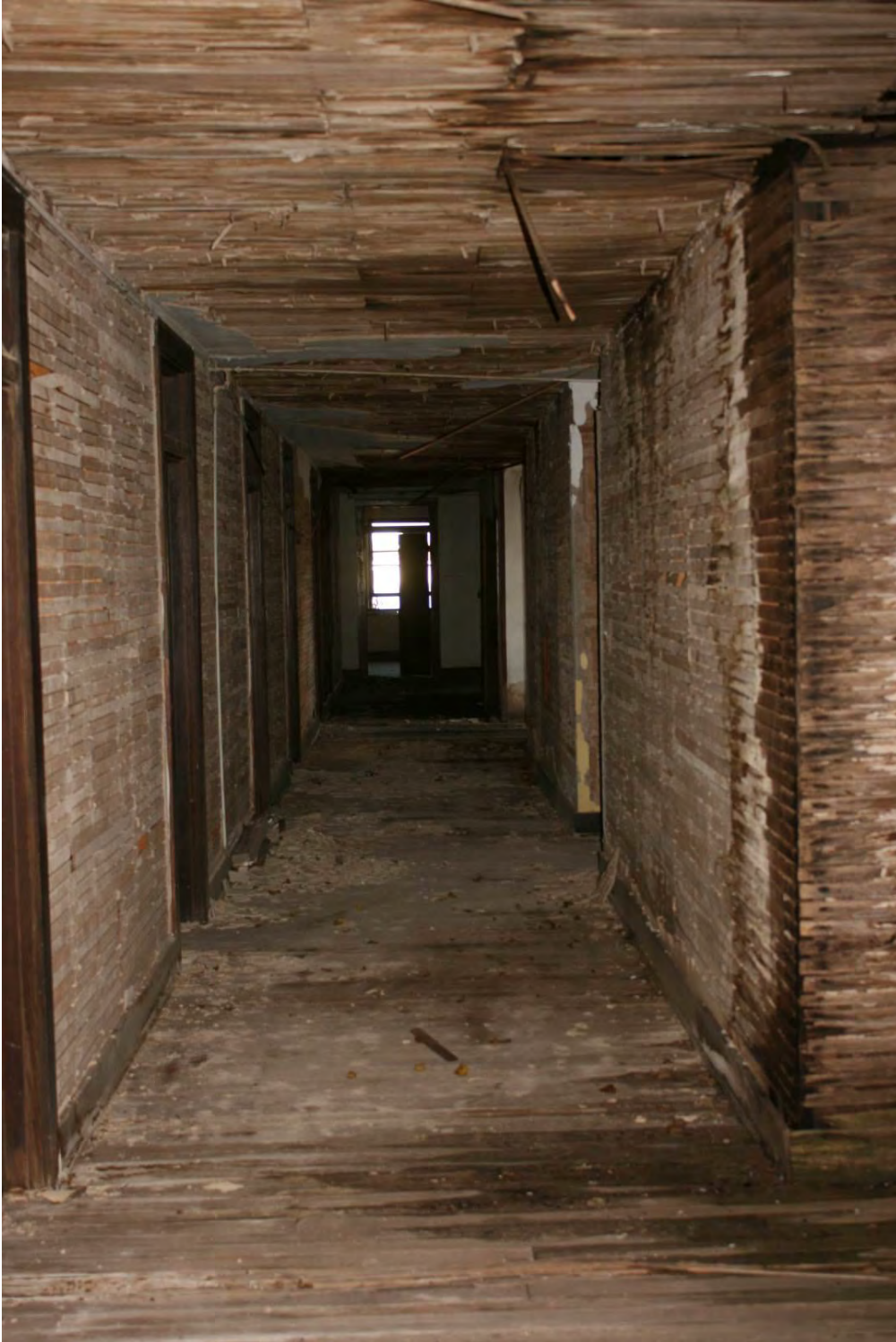
Photo 11: Second floor; East-west corridor. Camera facing east.
