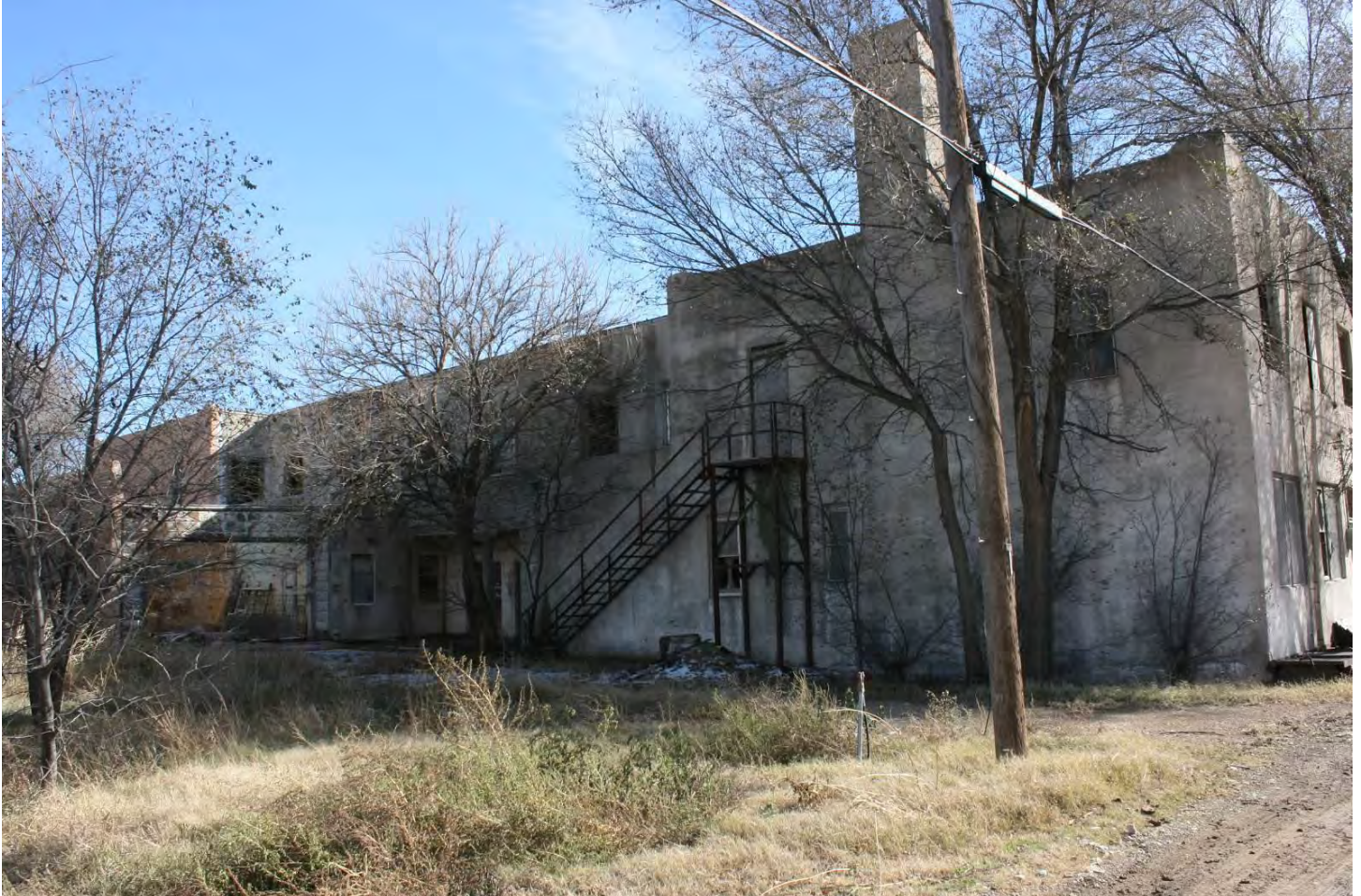
Photo 4: North elevation. Camera facing south.
