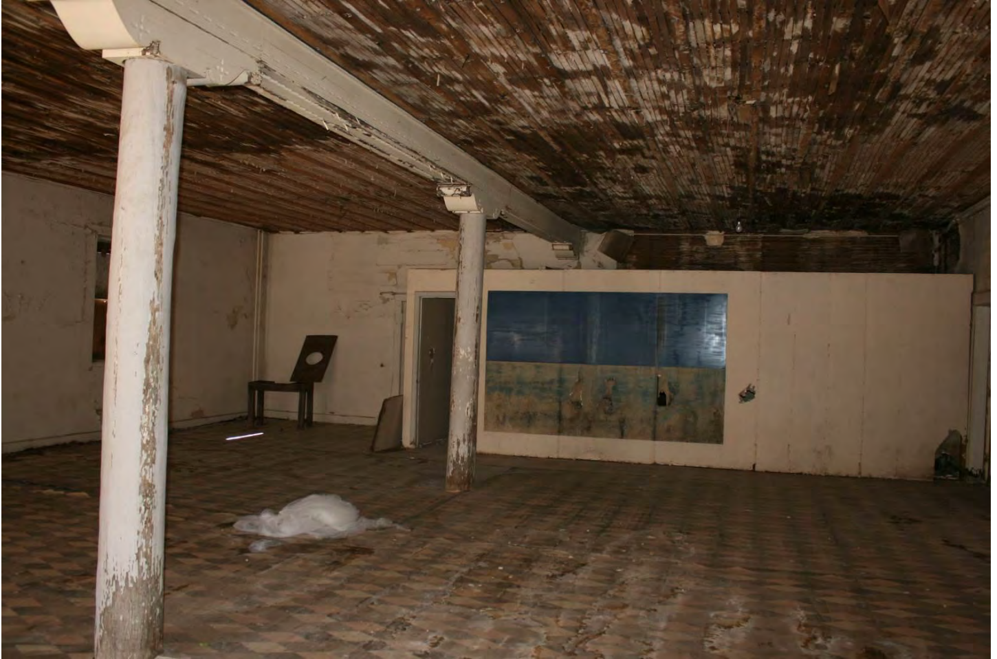
Photo 7: Ballroom. Camera facing north.
