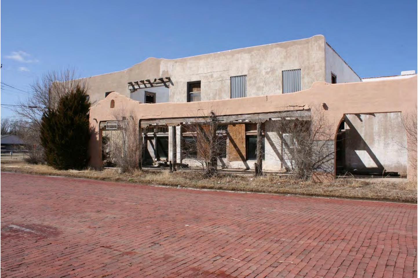
Photo 2: South elevation. Camera facing north.
