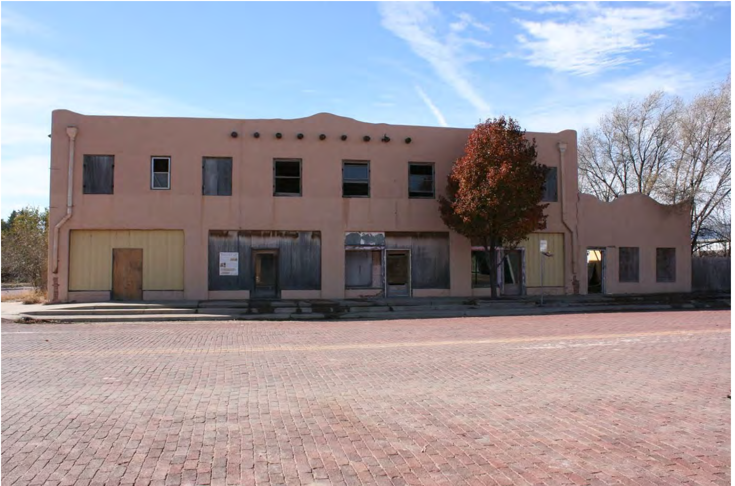
Photo 1: East elevation. Camera facing west.
