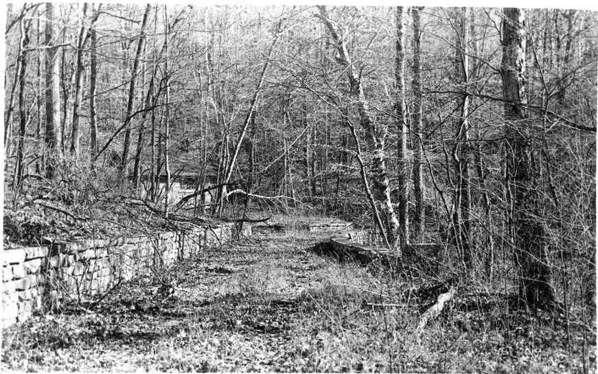
3. Three Springs Retaining walls (004A) Mammoth Cave National Park, Kentucky
