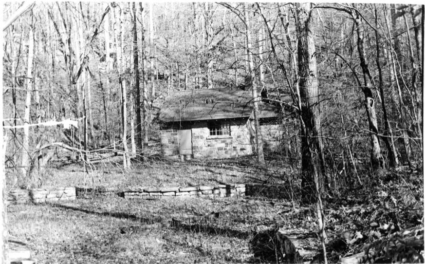
1. Three Springs Pumphouse (024) Mammoth Cave National Park, Kentucky
