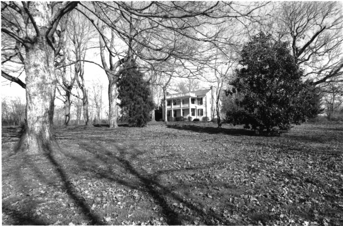
Smith, Alexander, House Williamson Co. TN
