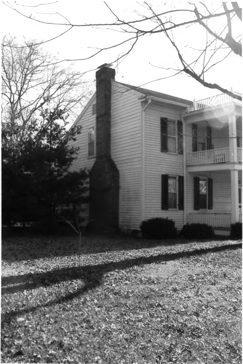
Smith, Alexander, House Williamson Co. TN
