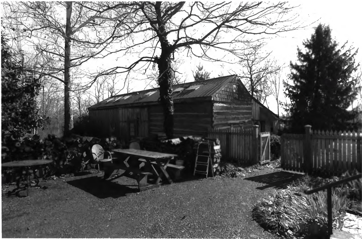
Smith, Alexander, House Williamson Co. TN
