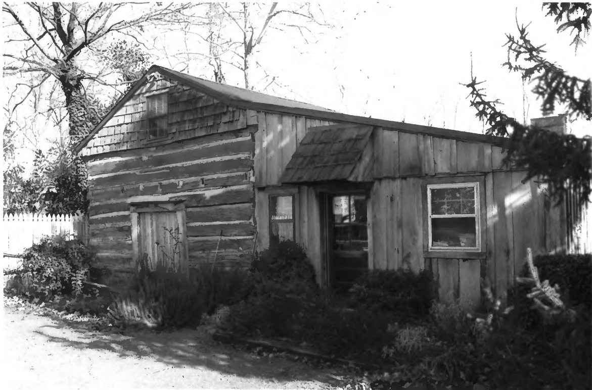
Smith, Alexander, House Williamson Co. TN
