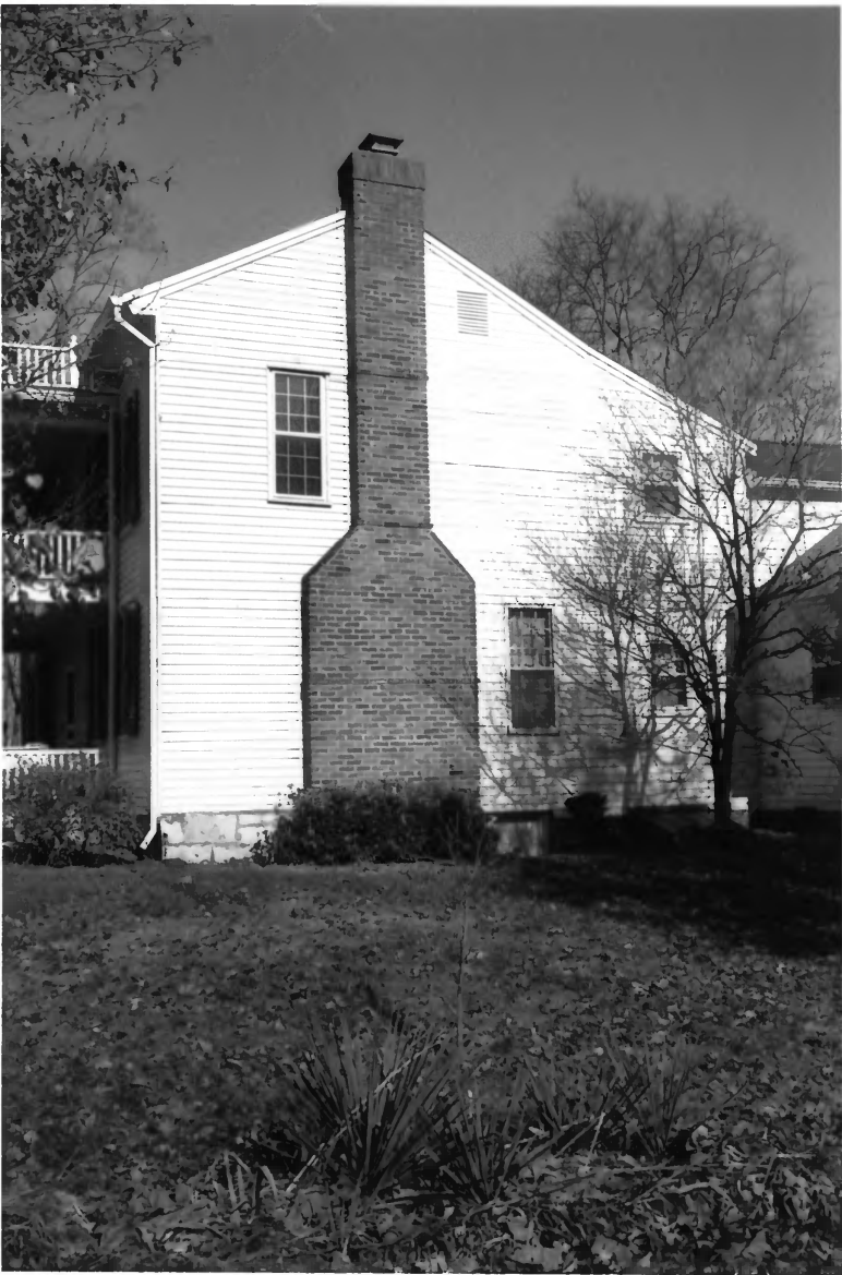
Smith, Alexander, House Williamson Co. TN
