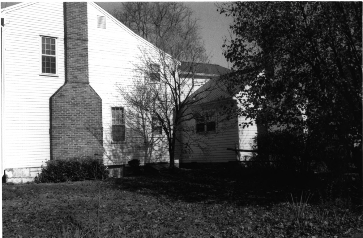
Smith, Alexander, House Williamson Co. TN
