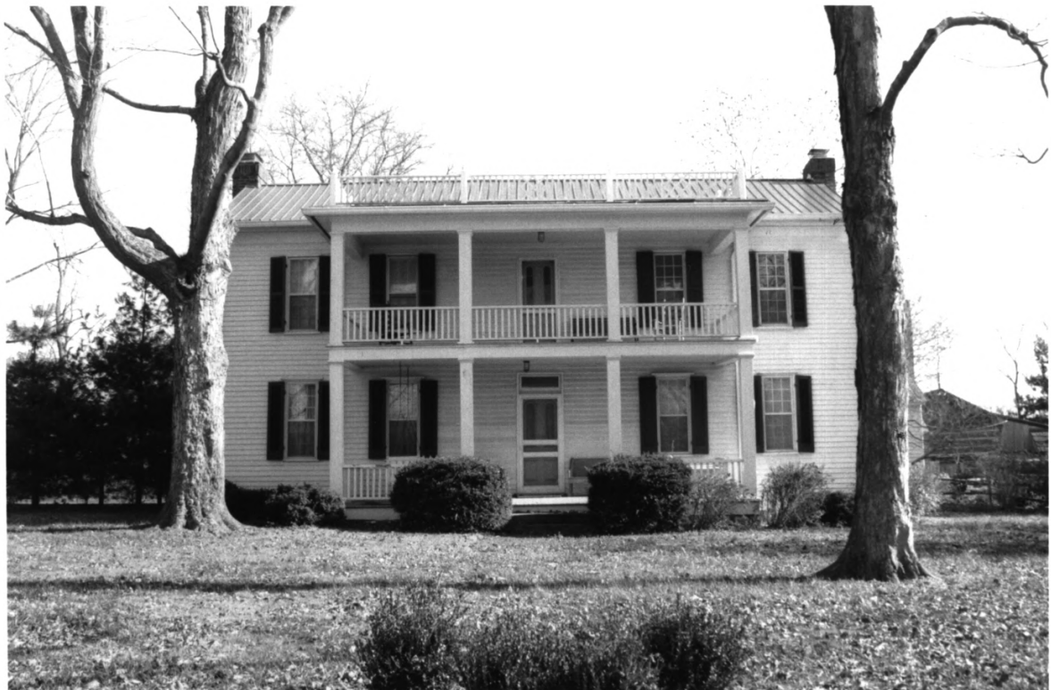
Smith, Alexander, House Williamson Co. TN
