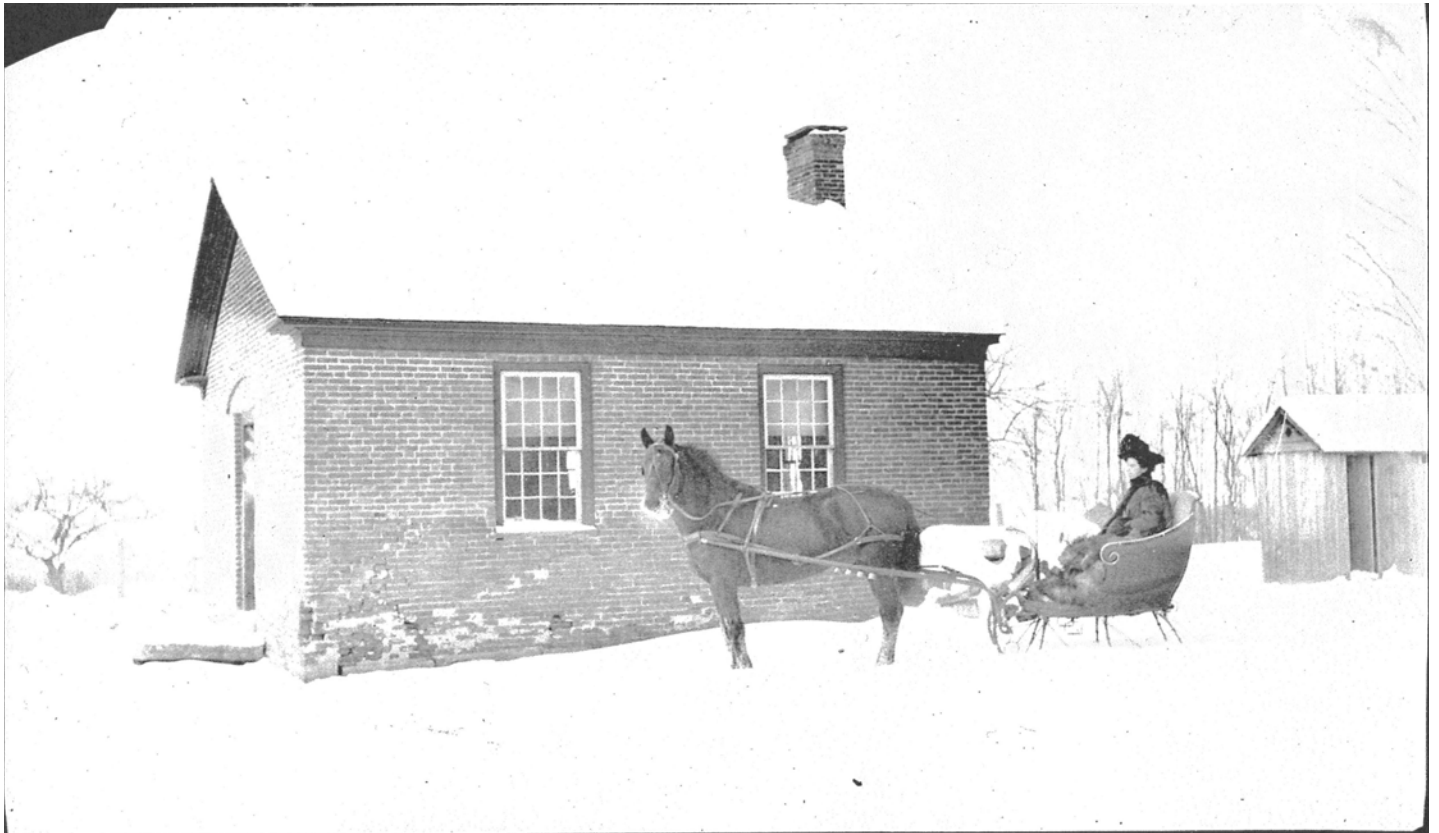
Figure 4: Glenville District No. 5 Schoolhouse - Photograph taken by Clarence Van der Veer in 1910
