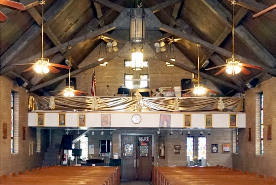
NJ_CAMDEN_ST. BARTHOLOMEW ROMAN CATHOLIC CHURCH_0016 Detail of the windows at the south end of the east and west nave walls, facing south.
