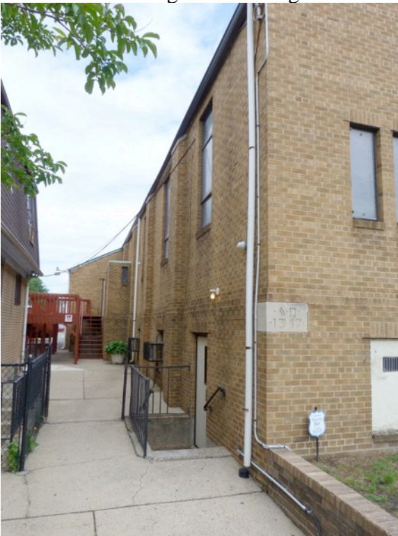
NJ_CAMDEN_ST. BARTHOLOMEW ROMAN CATHOLIC CHURCH_0005 Overall view facing north showing an oblique view of the west elevation of the church.
