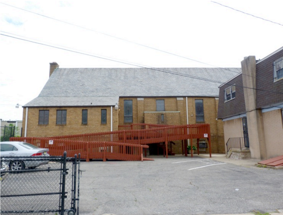
NJ_CAMDEN_ST. BARTHOLOMEW ROMAN CATHOLIC CHURCH_0004 Overall view facing east showing the northern portion of the west elevation of the church.
