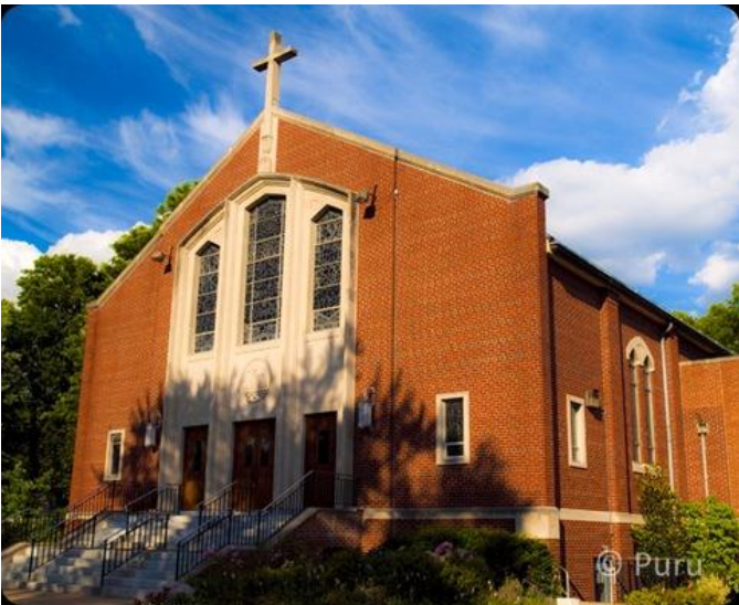
36 of 43 St. Andrew R.C. Church, Avel, NJ, 1957. http://www.twp.woodbridge.nj.us/Facilities/Facility/Details/St-Andrews-Roman-Catholic-Church-39
