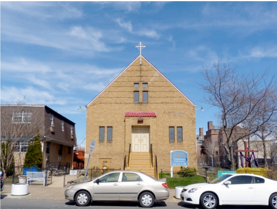
NJ_CAMDEN_ST. BARTHOLOMEW ROMAN CATHOLIC CHURCH_0007 View of the south elevation, facing north.
