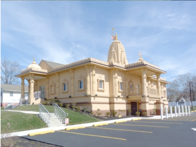
27 of 43 Holy Rosary as Swaminarayan Mandir Vasna Sanstha temple, façade after alterations, 2018. Photograph by Margaret Westfield
