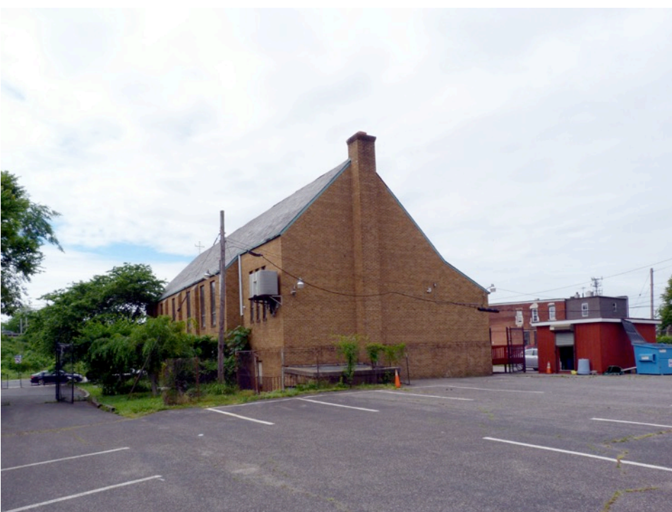
NJ_CAMDEN_ST. BARTHOLOMEW ROMAN CATHOLIC CHURCH_0003 Overall view facing southwest showing the east and north elevations of the church.
