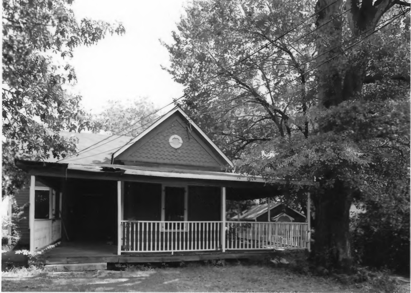
Atlanta - Frasier Street Historic District Cobb Co. , Georgia 3 of 12
