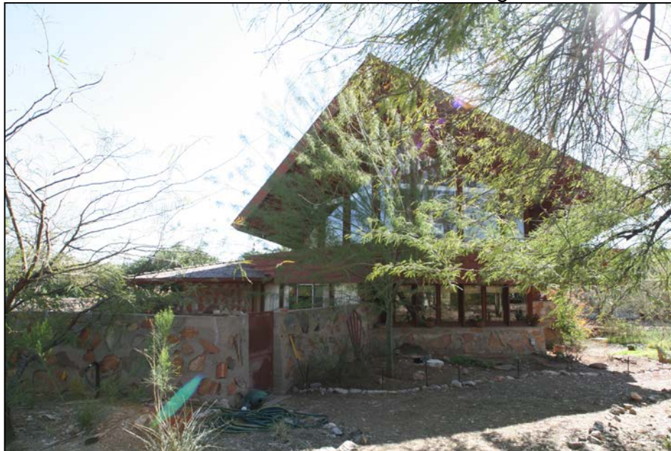
AZ_Maricopa County_Jorgine Boomer House_0006 Exterior View, N Elevation, Looking S
