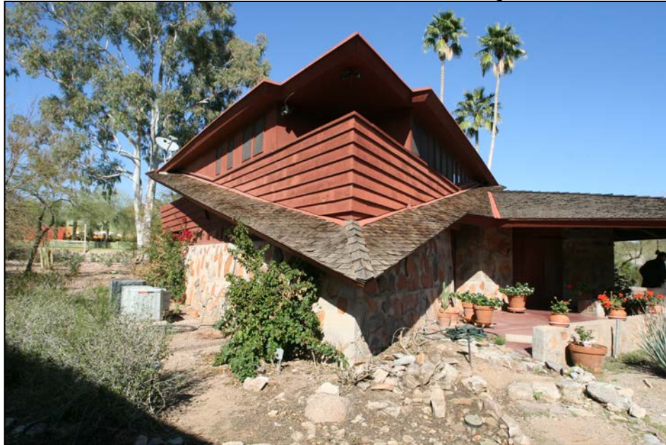
AZ_Maricopa County_Jorgine Boomer House_0003 Exterior View, SW Elevation, Looking NE
