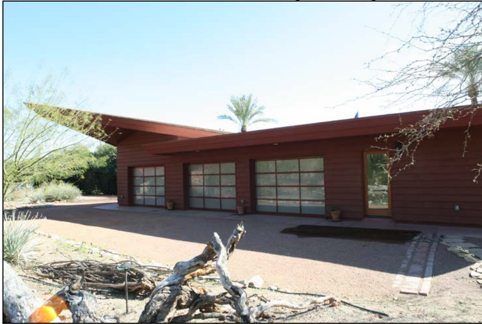
AZ_Maricopa County_Jorgine Boomer House_0017 Exterior View, 2013 Garage, Looking SE
