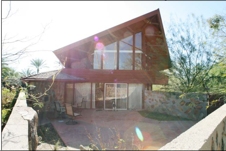
AZ_Maricopa County_Jorgine Boomer House_0007 Exterior View, NE Elevation, Looking SW
