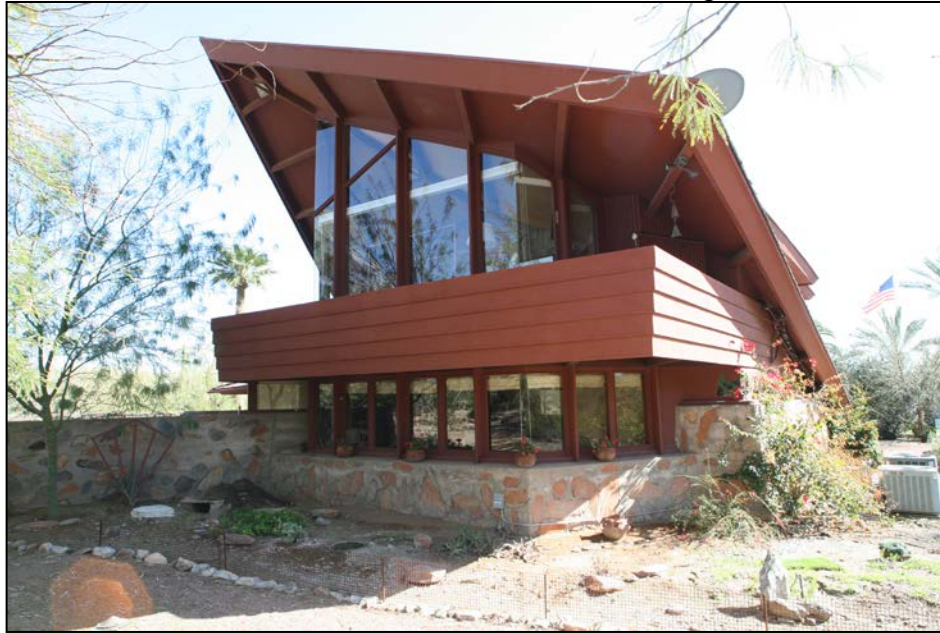
AZ_Maricopa County_Jorgine Boomer House_0005 Exterior View, NW Elevation, Looking SE
