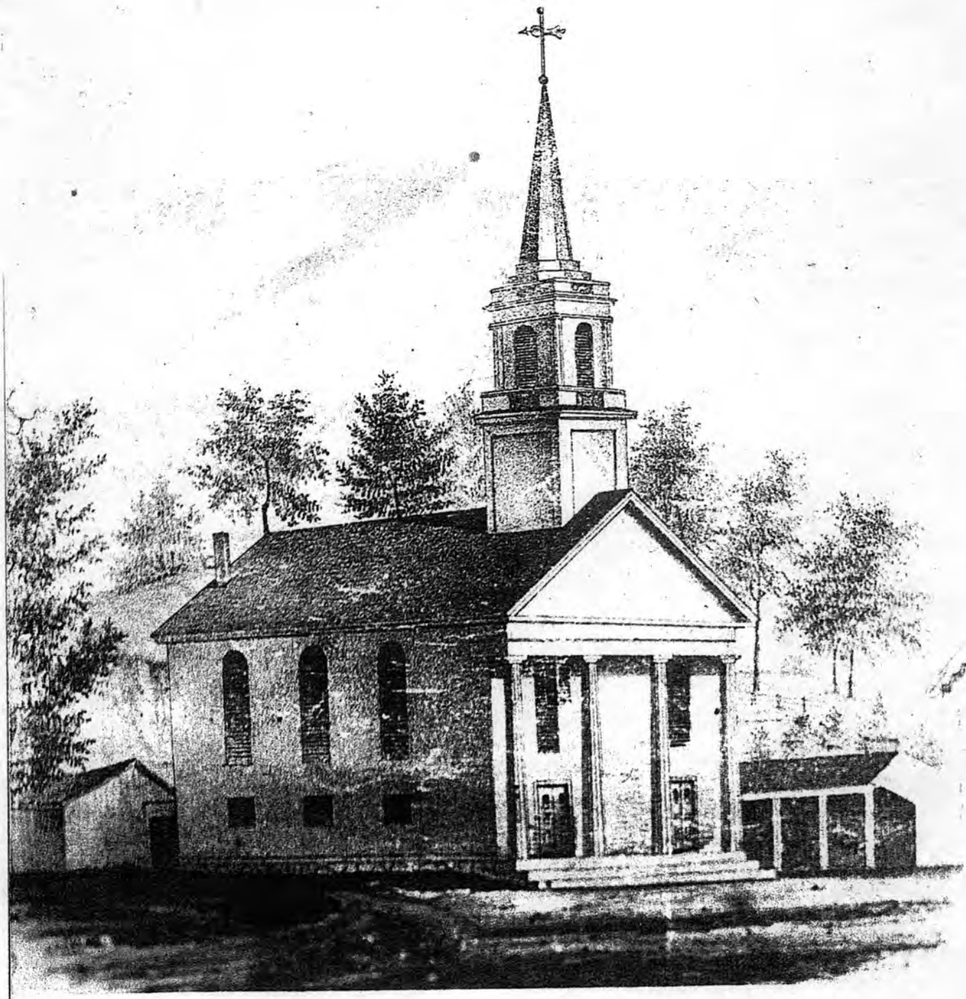
ILLUSTRATION # 3 The 1797 meeting house after its 1837 move off of the Common and remodeling By 1838 the old meeting house had taken the form of a Greek Revival style church, with a temple front and an integral steeple rising from its roof.
