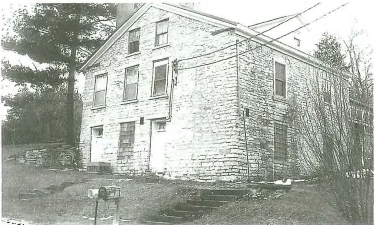
Figure 24. East and north elevations of the Boyle House in 2004 (HCHPC 2004: 34).
