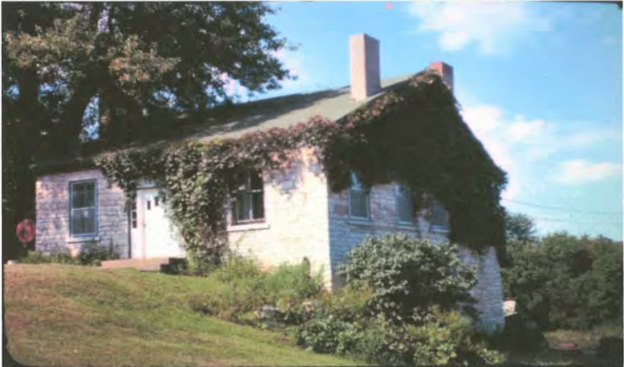
Figure 23. South and east elevations of the Boyle House in September 1975 (Young collection)
