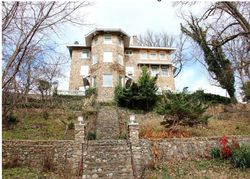
9. South wall of the house. Camera facing north.
