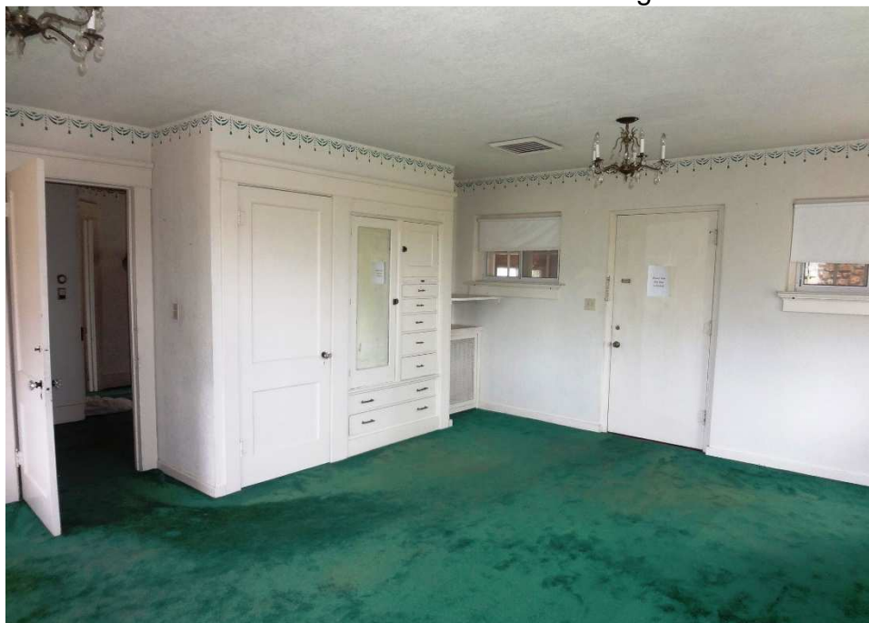
22. East bedroom in the third level. Camera facing northwest.
