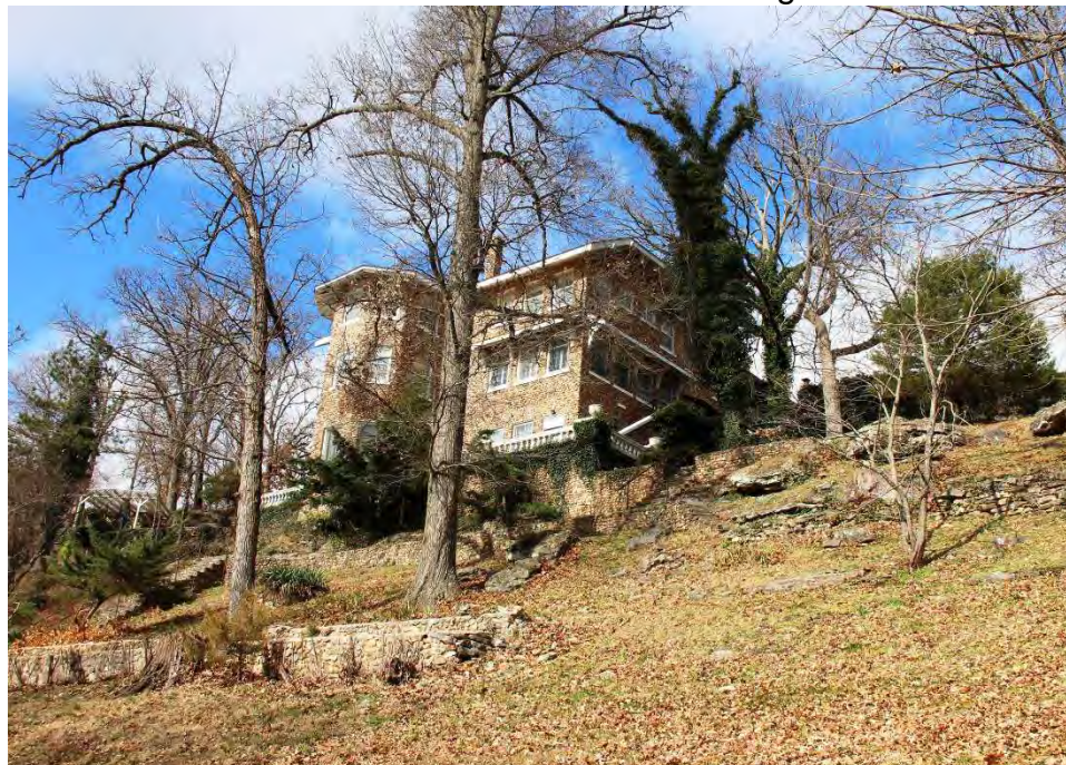
10. Southeast corner of the house. Camera facing northwest.
