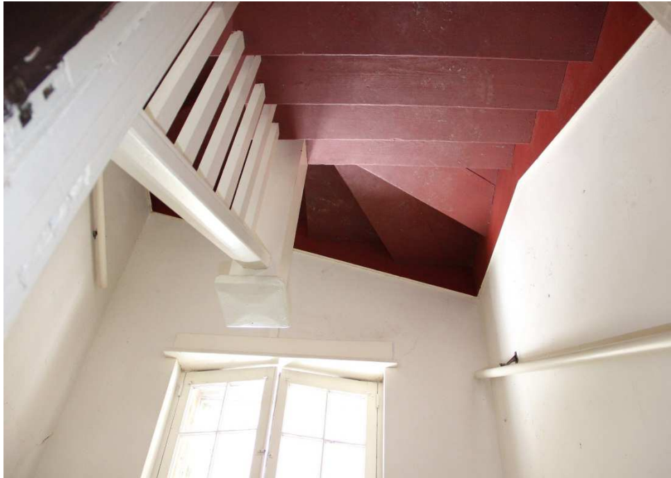
25. Guest house, stairway to garage. Camera facing east
