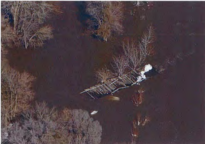
A portion of the missing Green Mill Bridge in Janesville that floated away in floodwaters is shown downstream Mor PHOTO COURTESY OF KIP LADAGE, BREMER COUNTY EMERGENCY MANAGEMENT
