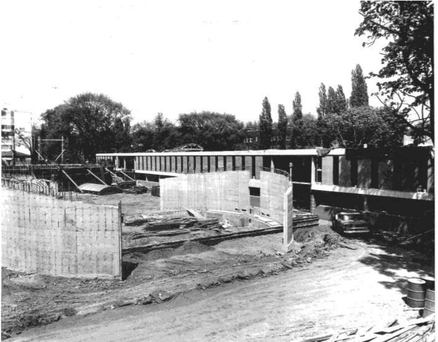
Figure 35: Temple Beth Zion – Building Construction; Sisterhood Chapel (May 25, 1965)
