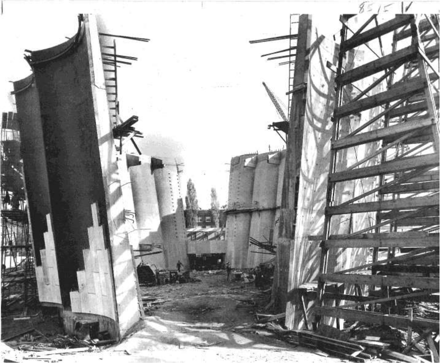
Figure 33: Temple Beth Zion – Building Construction; Sanctuary (November 4, 1965)
