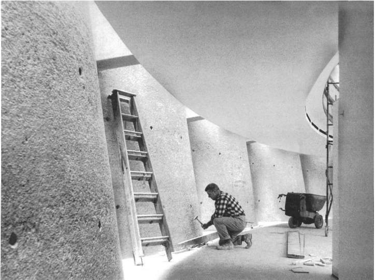
Figure 34: Temple Beth Zion – Building Construction; workman finishing interior concrete walls (November 4, 1966)
