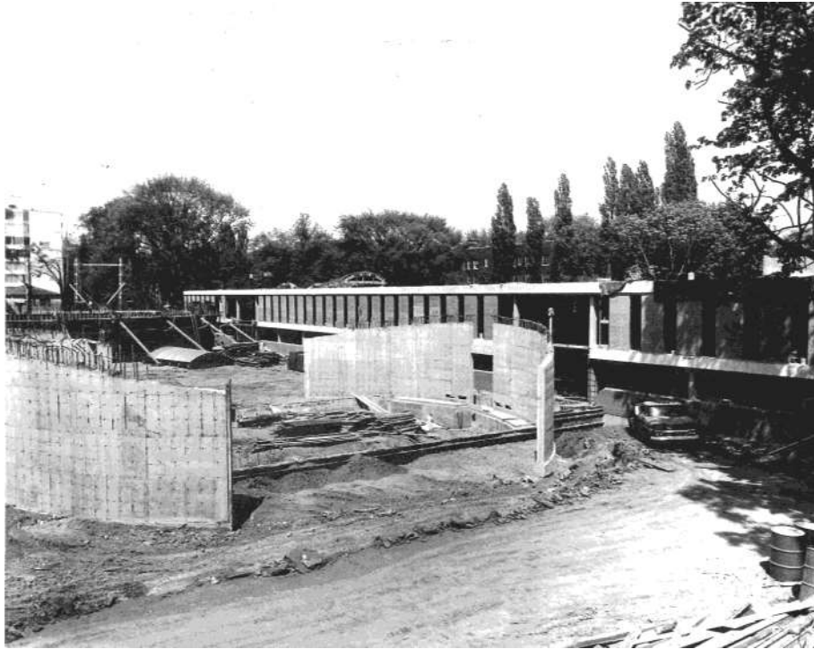
Building Construction; Sisterhood Chapel (May 25, 1965)
