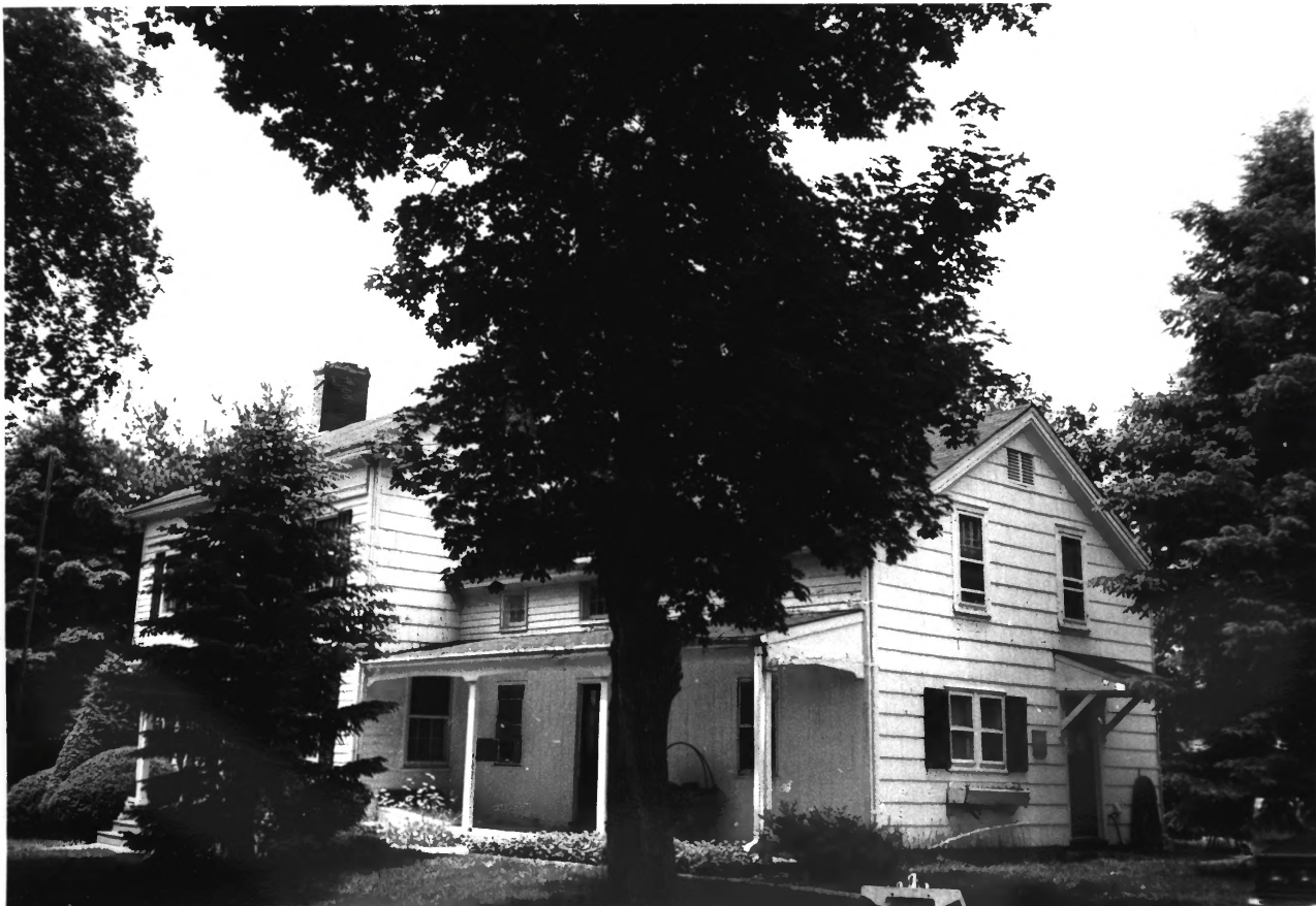
NJ 023 RICHARD FIELD JR HOUSE, WING ON NE END
