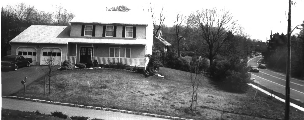
NJ 0283 VIEW FROM HILLSIDE SETTING OF FIELD HOUSE - EAST
