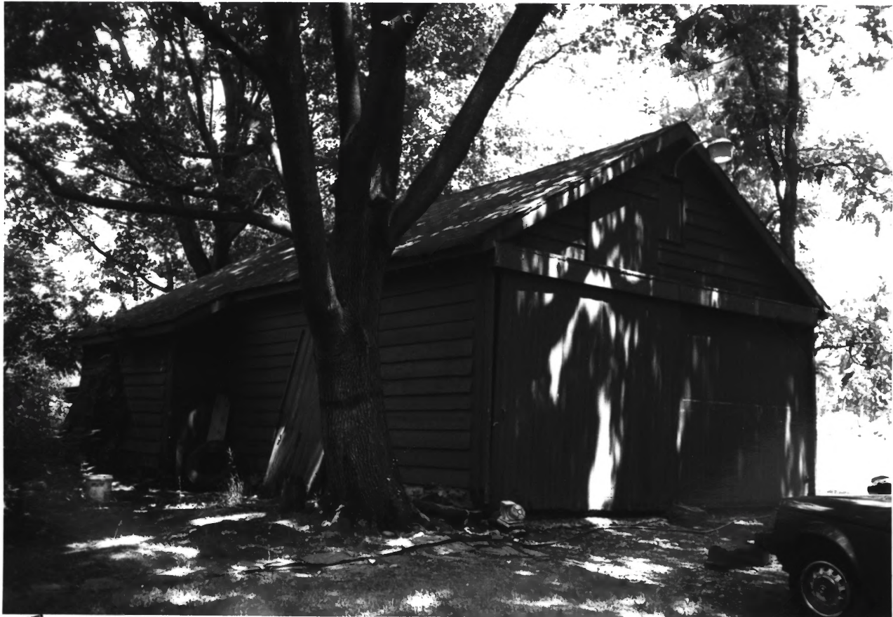
NJ 023 BARN AT JONATHAN SMOCK'S HOUSE
