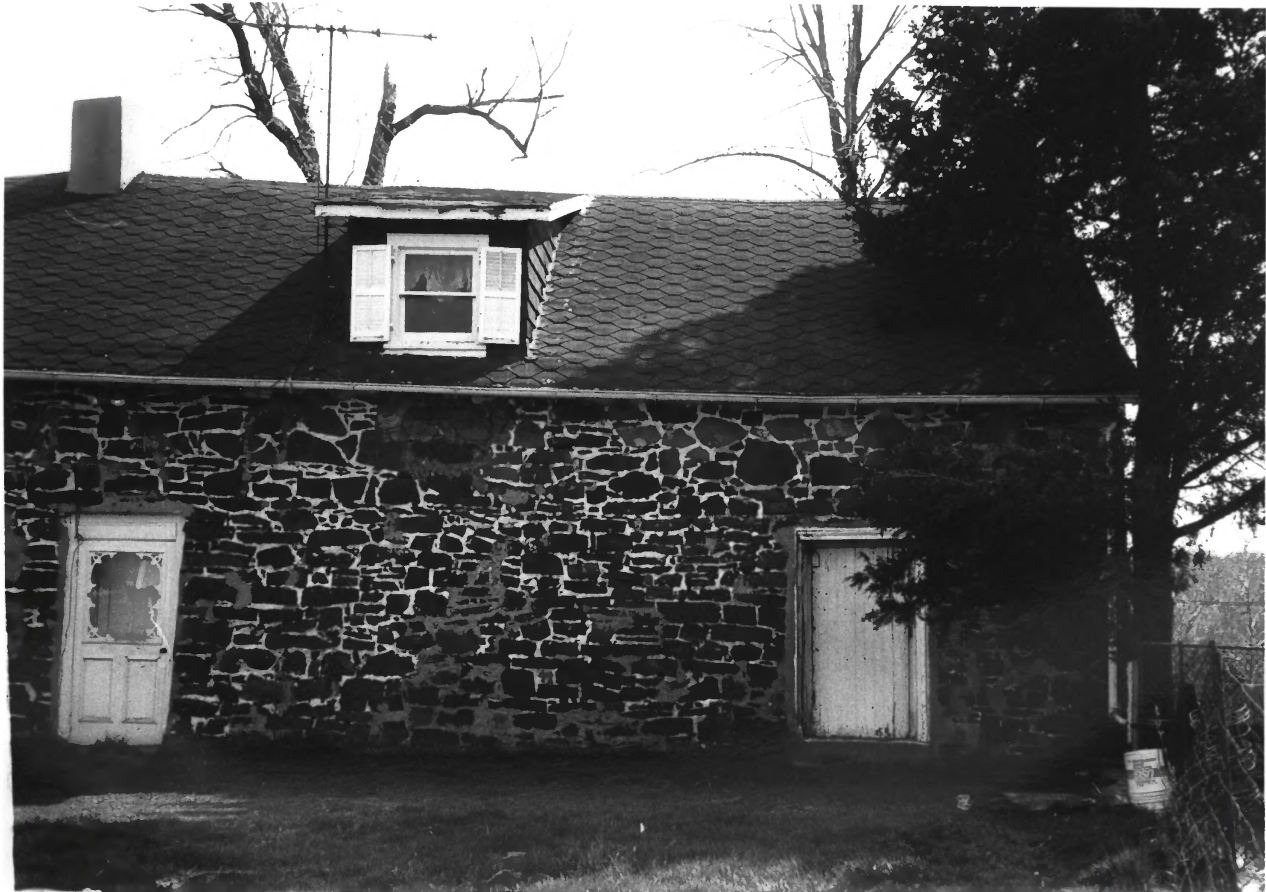
NJ 023 REAR FACADE - JOHN FIELD HOUSE
