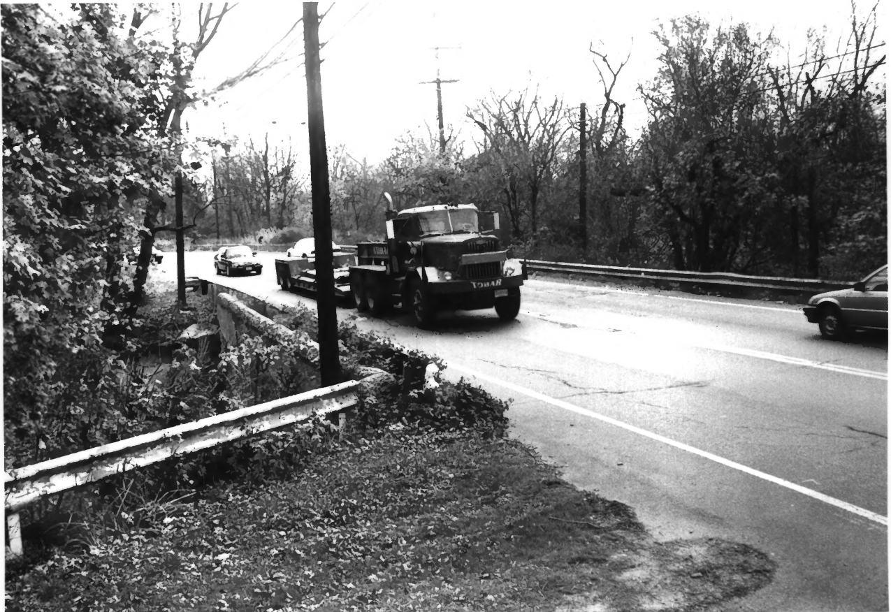
NJ 023 RIVER RD - looking SE by McETP's Brook (by J. Smock), 44/49
