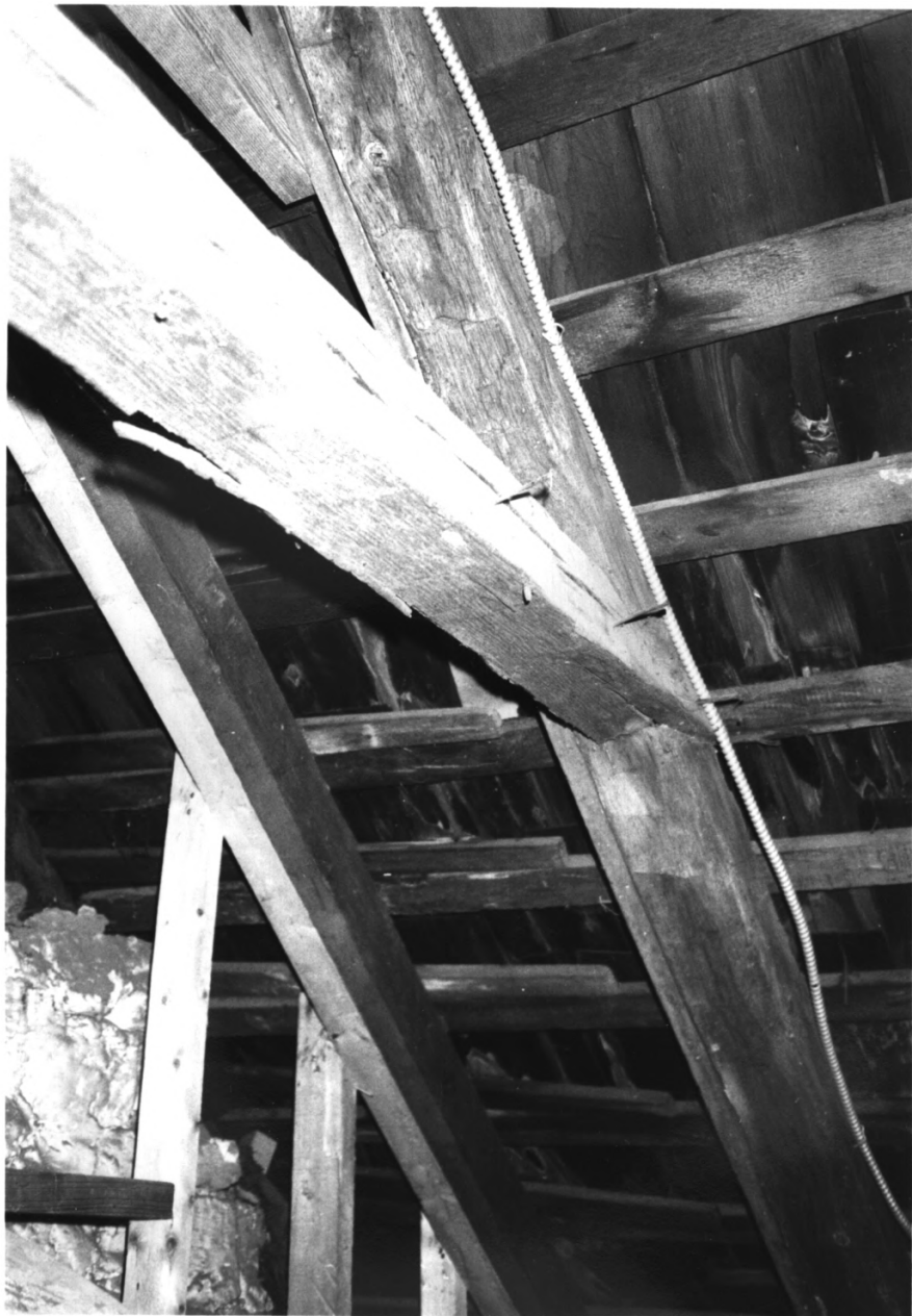
NJ023 Attic details, J. FIELD HOUSE
