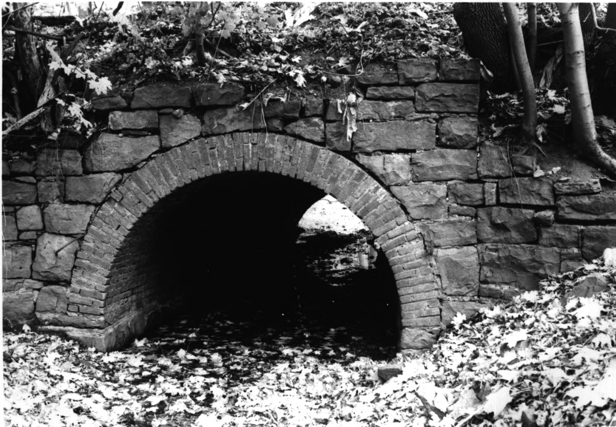
NJ 023 Early arched bridge over McEtie Brook
