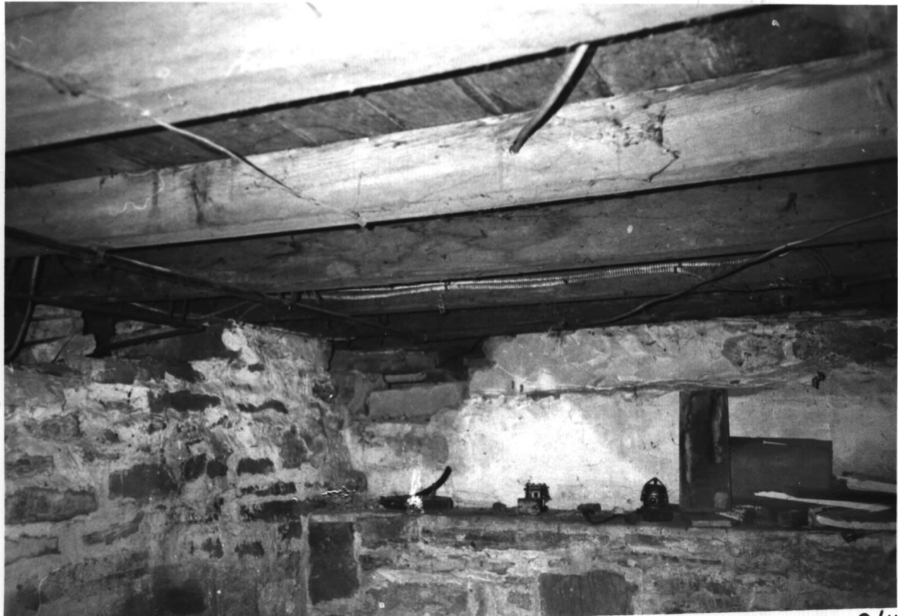
NJ 023 ONLY FOUNDATION OF OUDE DONK-BOUKAM HOUSE
