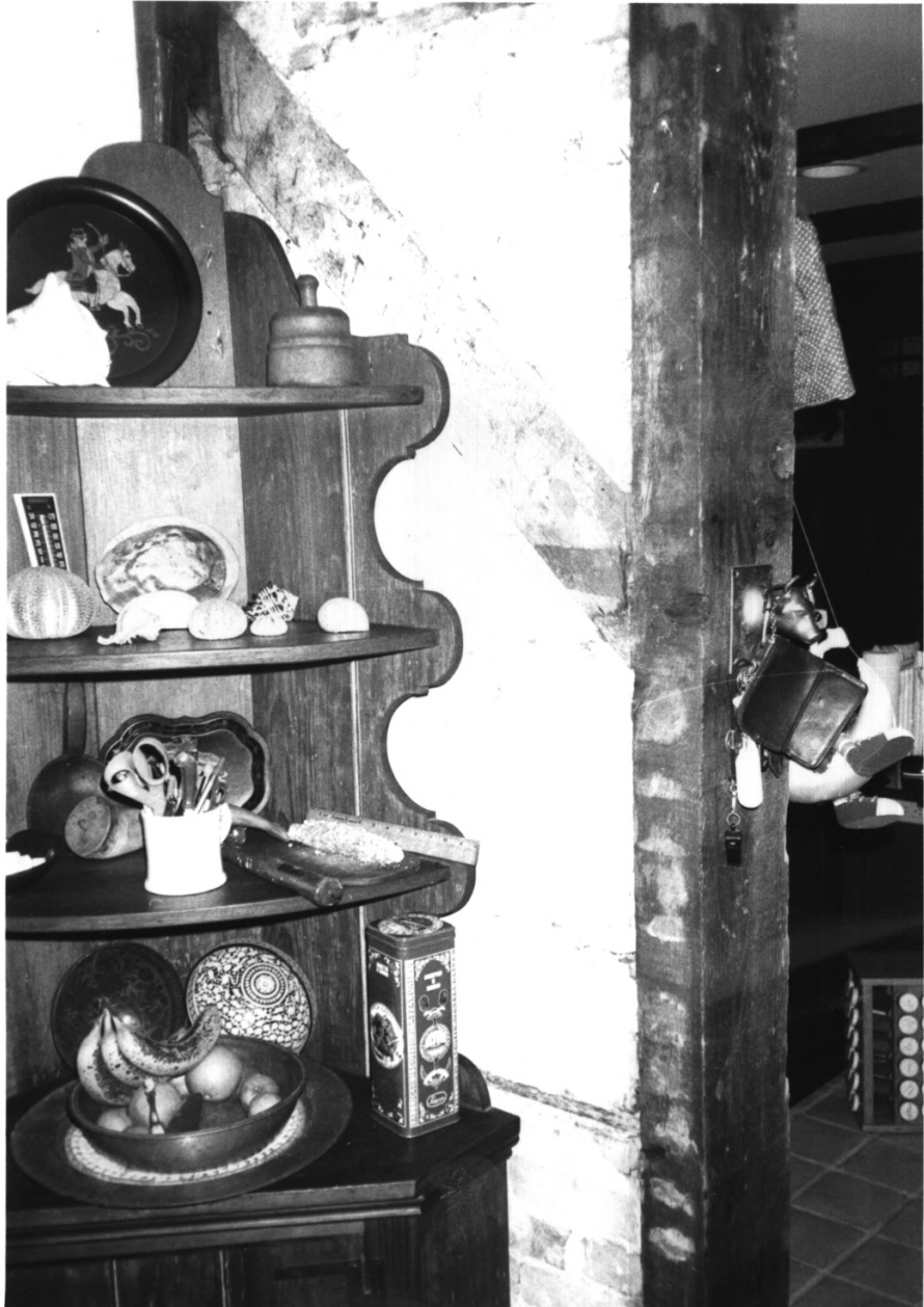
105203 033 EXPOSED EARLY FRAMING, I. OUDERDONK'S 20/49
