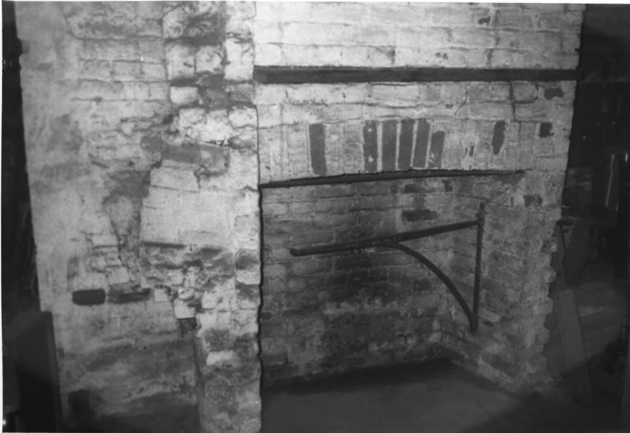
NJ 023 LEWIS ONDERDONK HOUSE, CELLAR
