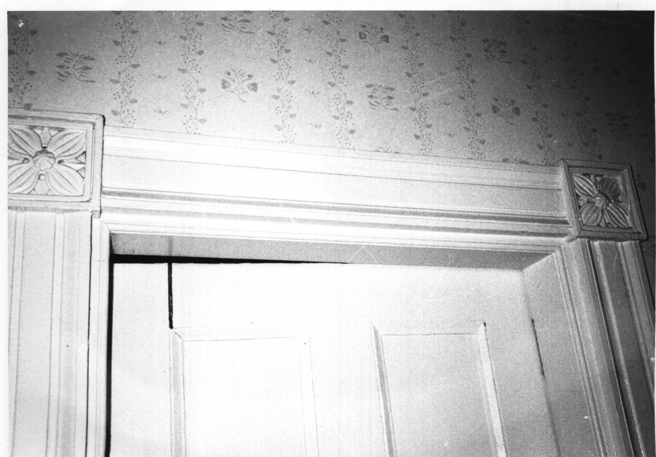
NS 023 LINTEL ORNAMENTATION, FRAMING, FIELD/DUNHAM HOOSE 13/49
