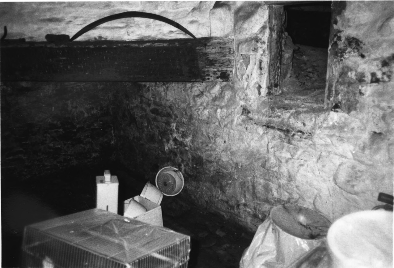
NJ 023 Support in cellar for corner fireplace, I. ONDERDONK house
