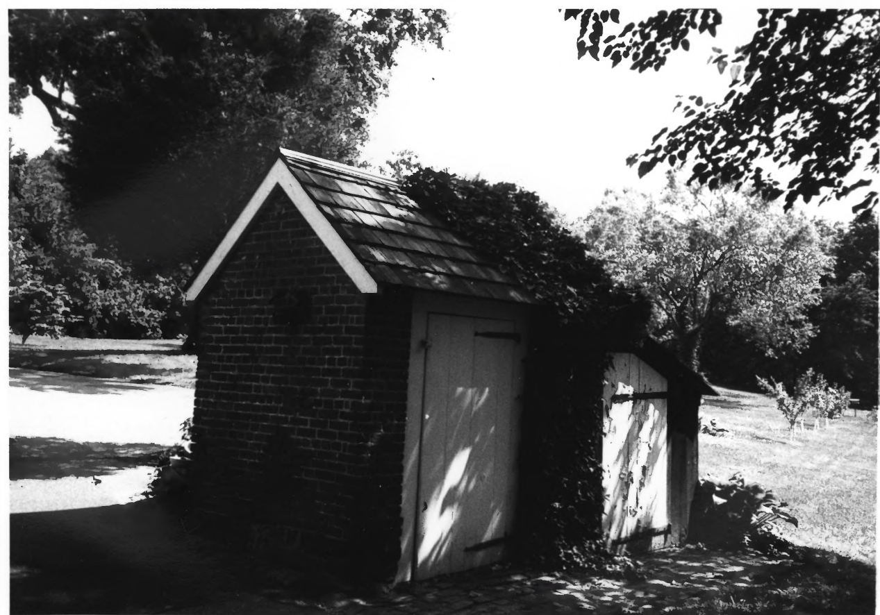
NJ 623 SPRING HOUSE, ISAAC ONDERDONK HOUSE
