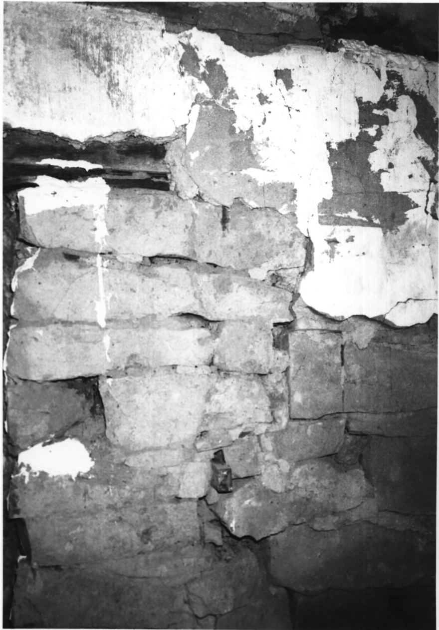
NJ023 CELLAR WALL - J. FIELD HOUSE
