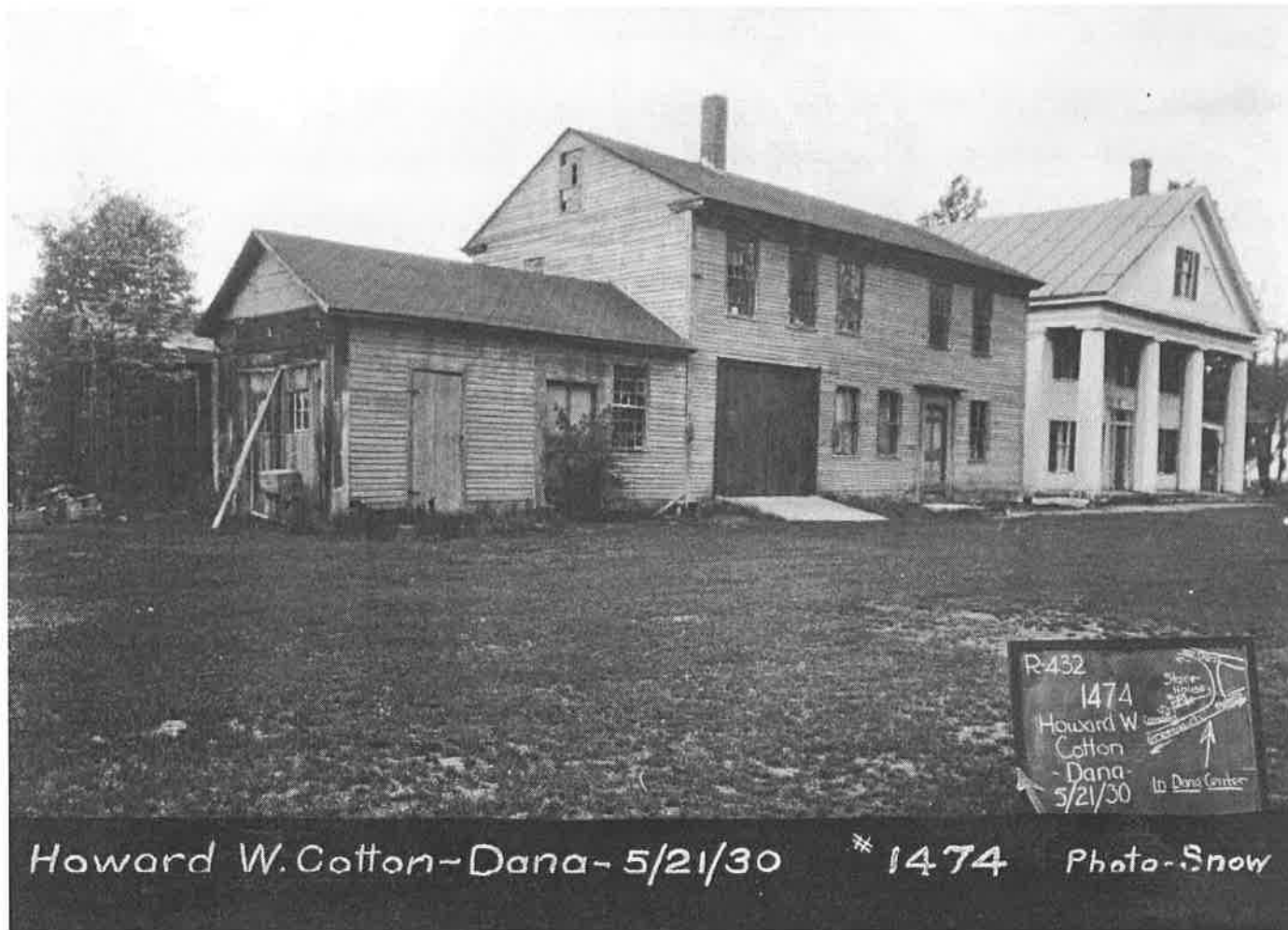
Historic Photo 18. Howard W. Cotton [storehouse] (Map #16). MDWSC Real Estate Photo 1474, May 1930.
