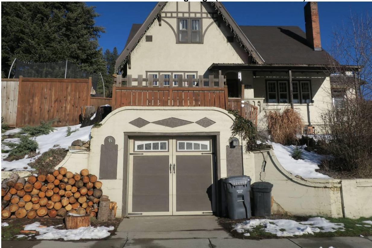
Photo 6: View Northeast of garage (southwest elevation)
