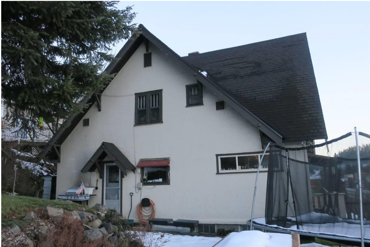
Photo 5: View Southeast of Northwest elevation
