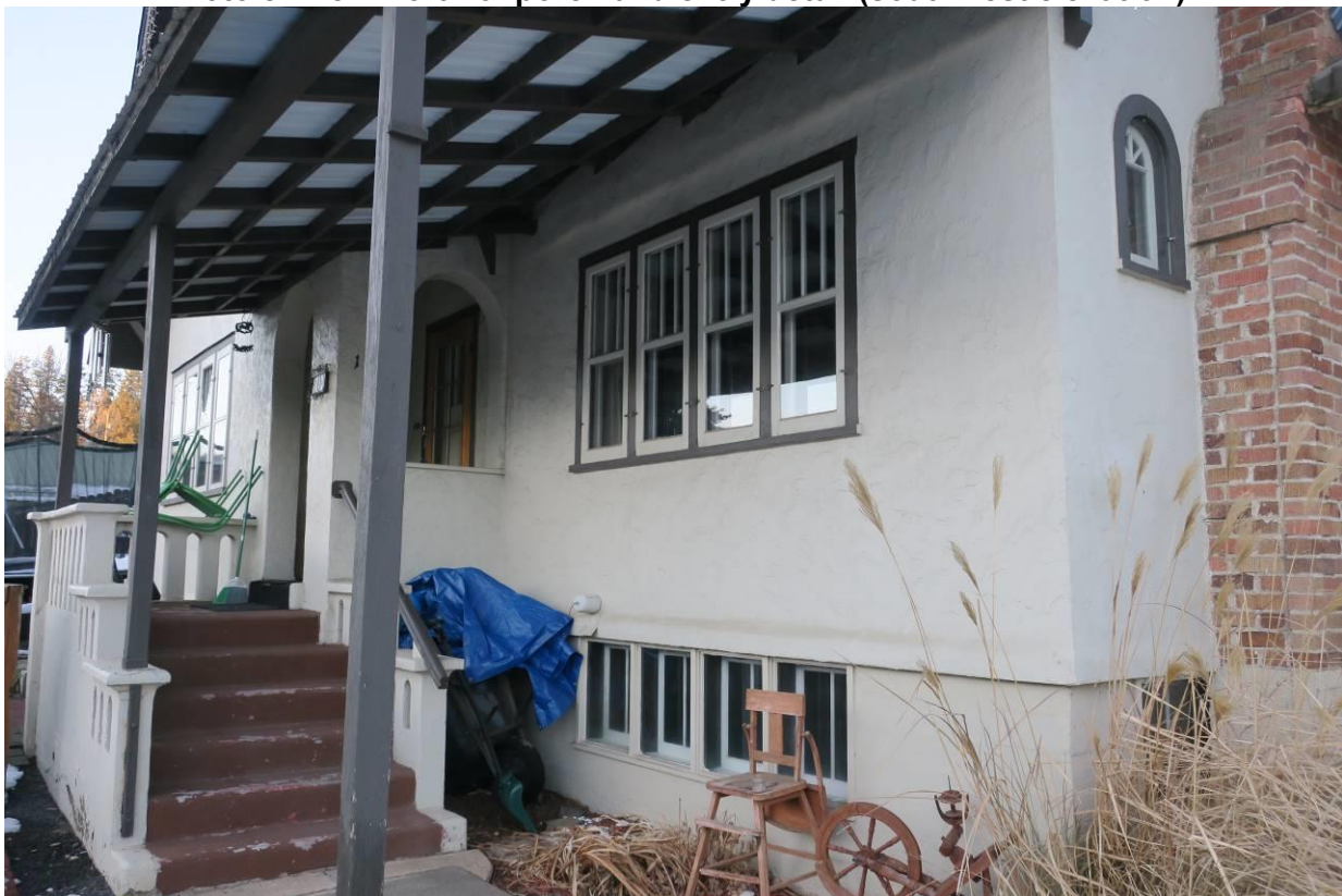
Photo 8: View North of porch and entry detail (southwest elevation)
