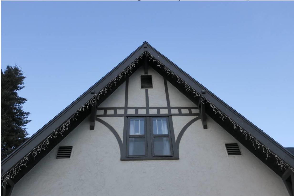
Photo 7: View Northeast of gable detail (southwest elevation)
