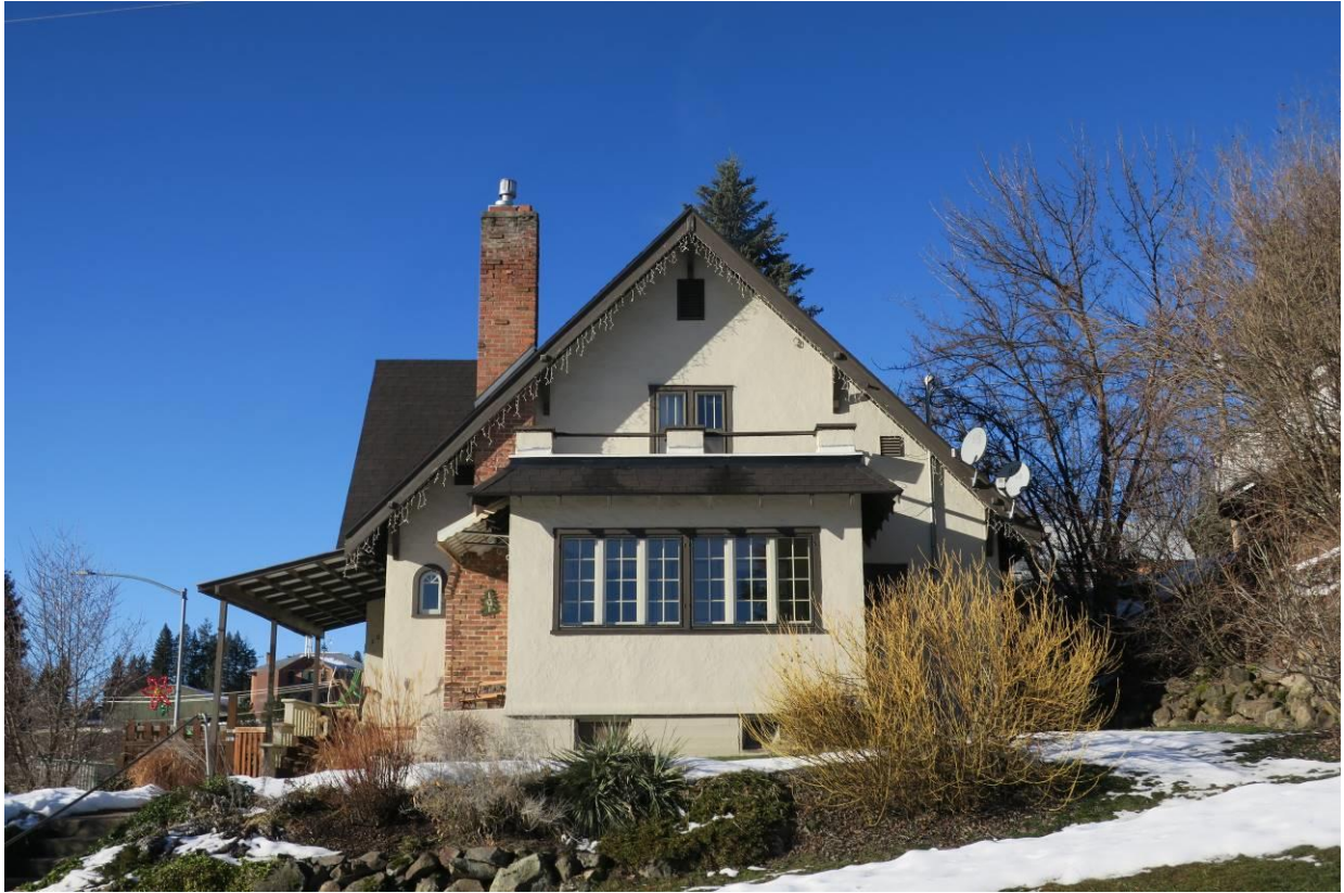
Photo 3: View Northwest of Southeast elevation
