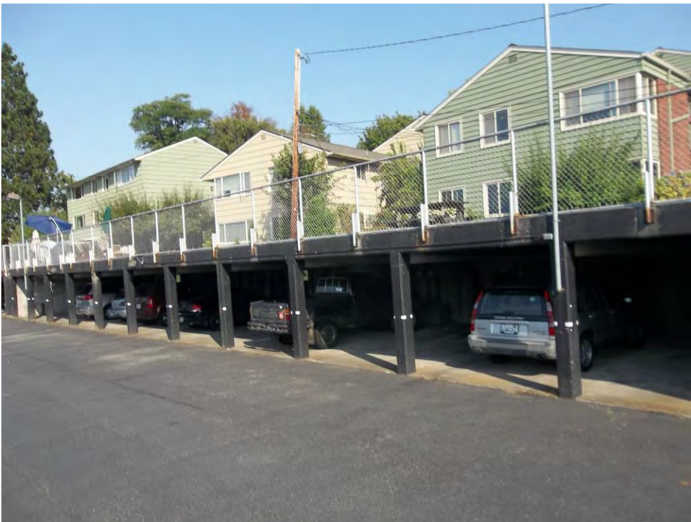
9 of 20 Northeast boundary, showing Carport and Building No. 2, 3 and 4.
