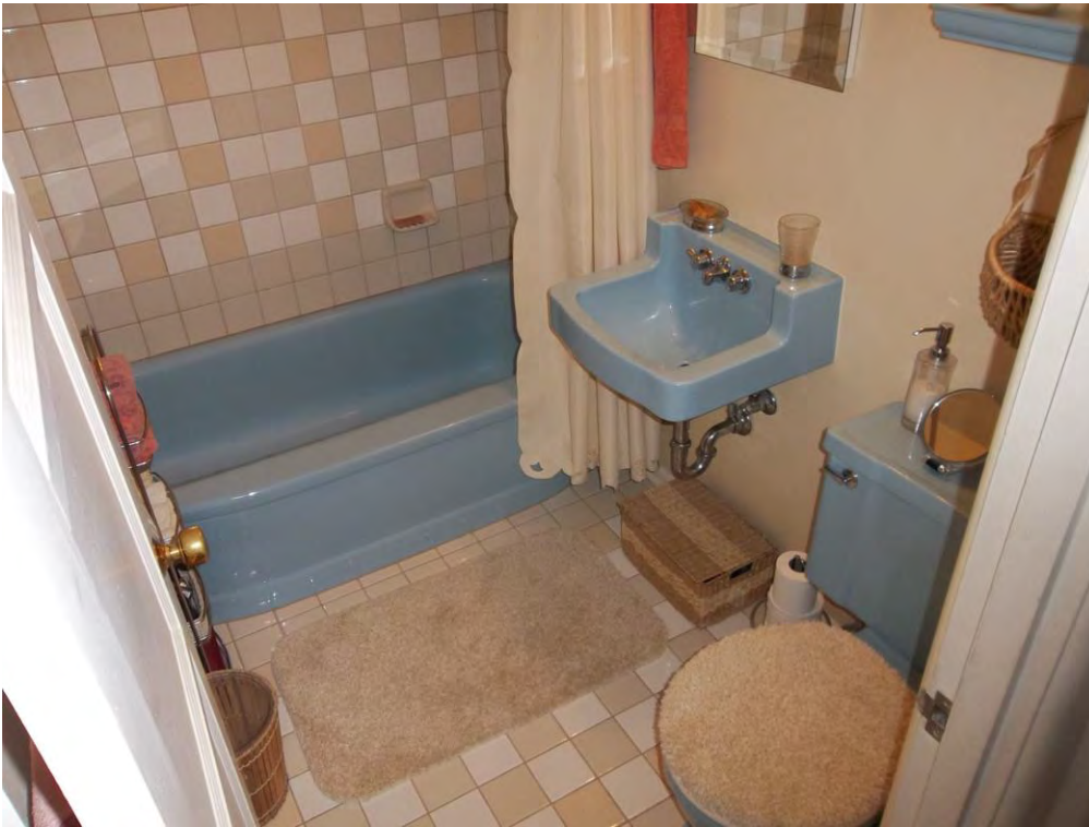
16 of 20 Unit showing original blue bathroom fixtures.
