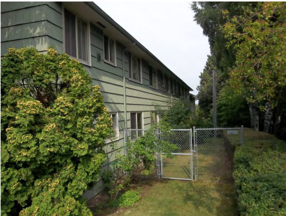
5 of 20 Northwest boundary line from North Forest Street at Building No. 2.
