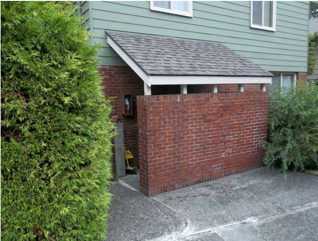
20 of 20 Waste storage pavilion attached to unit.
