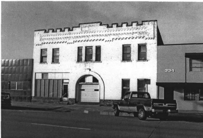
Armory Building Prior to Rehabilitation, 1992 Office of Archaeology and Historic Preservation, Colorado Historical Society
