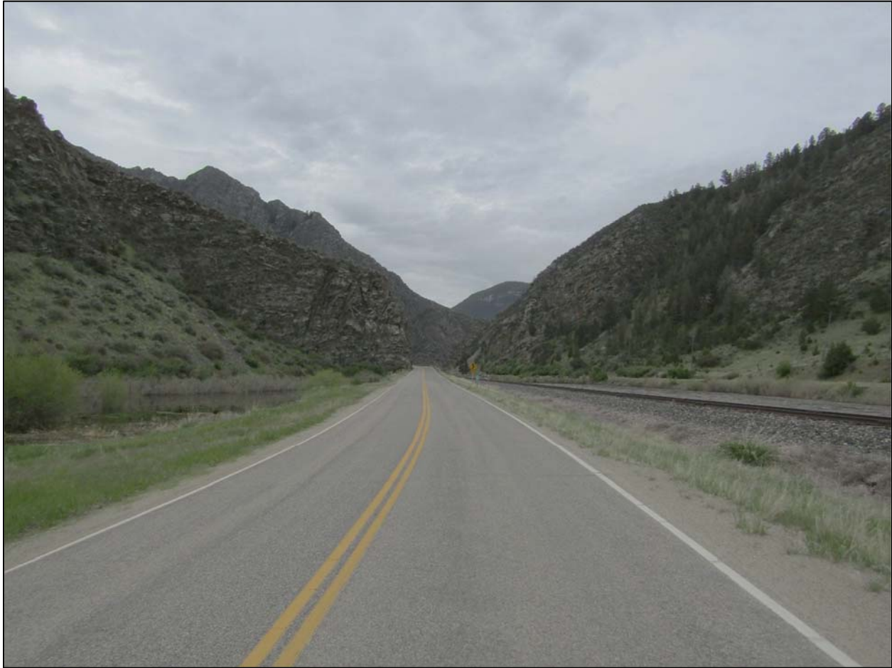
Photo # MT_JeffersonCounty_JeffersonCanyonHighwayHD_0008: The Jefferson Canyon Highway Historic District. Beginning of Segment 2 (Milepost 3.0). View to the southeast. Photo date: May 23, 2018.
