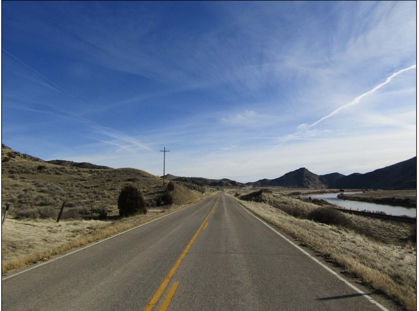
Photo # MT_JeffersonCounty_JeffersonCanyonHighwayHD_0024: The Jefferson Canyon Highway Historic District. Milepost 7.67. View to the east. Photo date: November 30, 2017.
