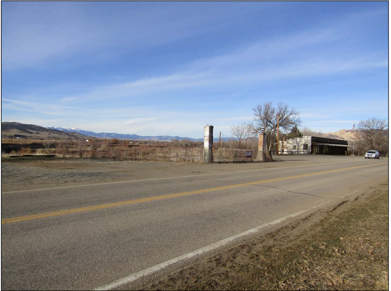
Photo # MT_JeffersonCounty_JeffersonCanyonHighwayHD_0005: The Jefferson Canyon Highway Historic District. Mountain View Inn site (Milepost 2.3). View to the northwest. Photo date: November 30, 2017.
