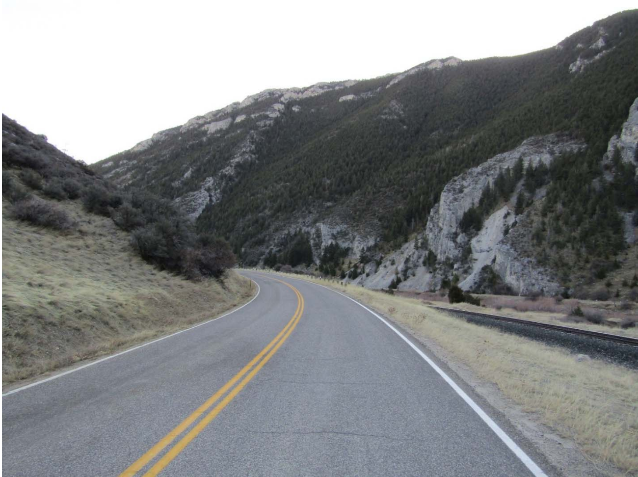
Photo # MT_JeffersonCounty_JeffersonCanyonHighwayHD_0015: The Jefferson Canyon Highway Historic District. Milepost 4.03. View to the south. Photo date: November 30, 2017.
