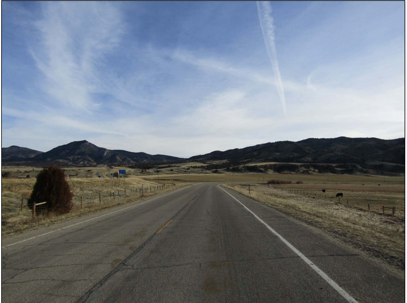
Photo # MT_JeffersonCounty_JeffersonCanyonHighwayHD_0001: The Jefferson Canyon Highway Historic District. Beginning of Segment 1 (Milepost 0.6). View to the east-northeast. Photo date: November 30, 2017.
