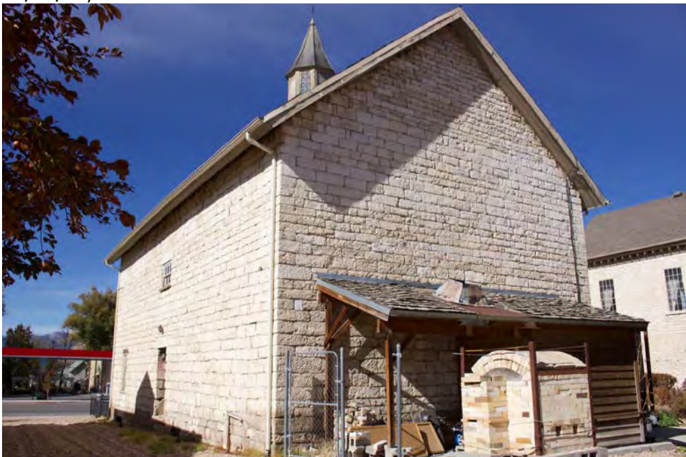
4 of 21: South-east corner of granary. Camera facing north-west. (Photo by Jamyn Maddox, 10/31/18)
