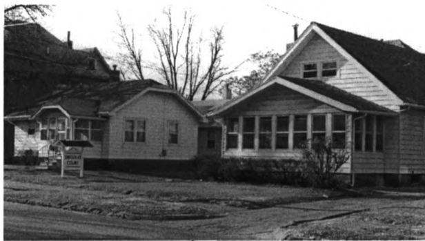
1228 (left) and 1232 (right) East 12 th Street, view to southeast, Court Entrance (photo by James Jacobsen, December 7, 1999)
