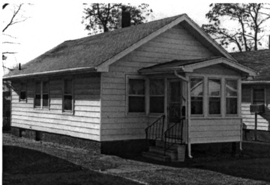
1107 Doukas Court, south bungalow row example, view southwest (photo by James Jacobsen, December 7, 1999)
