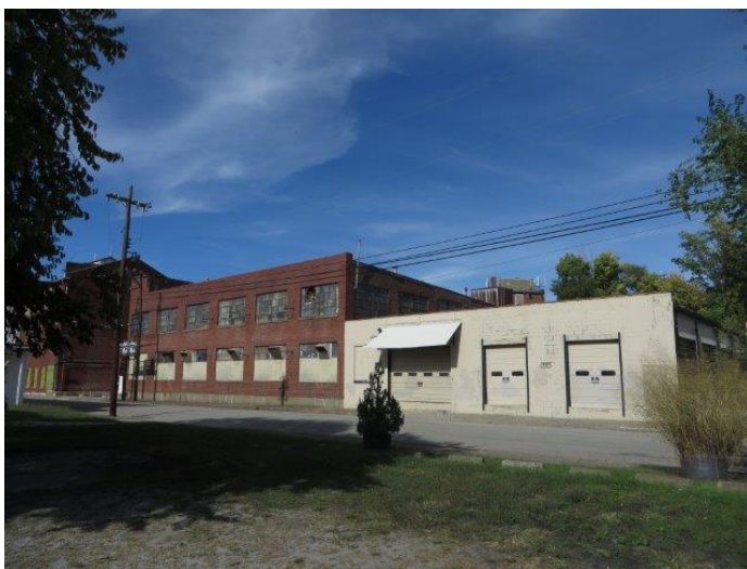
Primary (west) façade, along Brent Street
