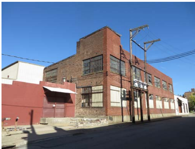
West façade, along Brent Street
