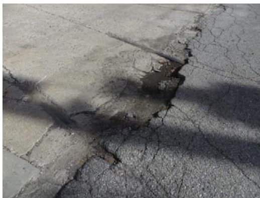
Pavement and Railroad tracks on North side
