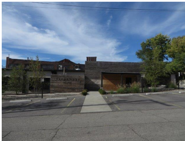
South façade, Louisville Stoneware entrance
