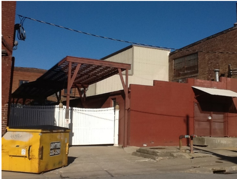
2015 photo showing railroad tracks adjacent to yellow "anytime" dumpster
