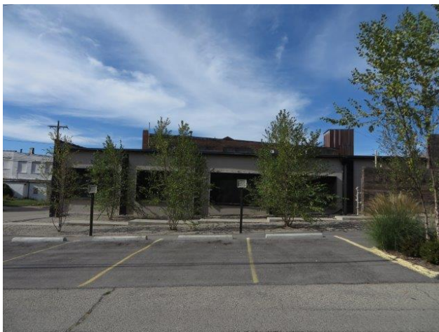
South façade, Louisville Stoneware Parking
