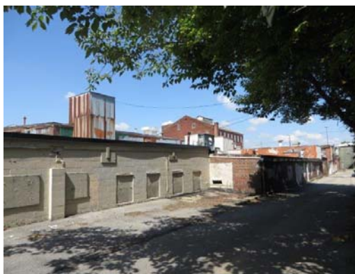
East Façade from northern part of alley
