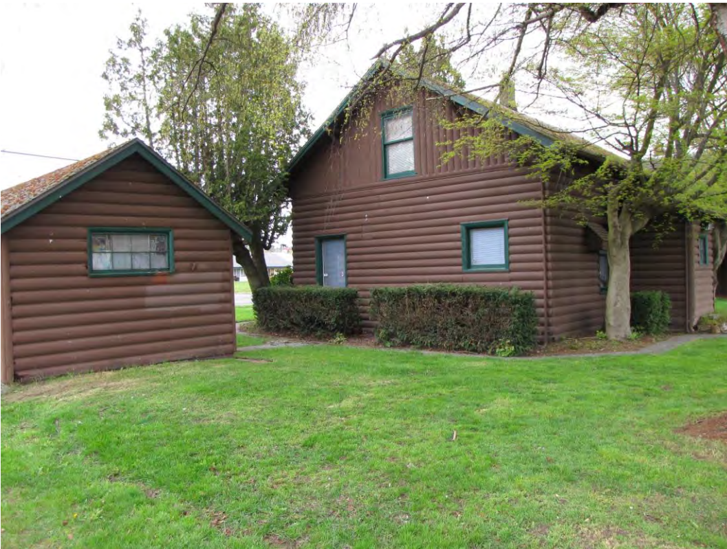
15 of 15 – Rear of caretaker garage & cottage taken from southwest corner, No. 0015
