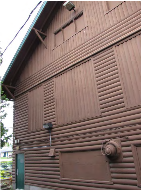
8 of 15 – West façade of fieldhouse, No. 0008
