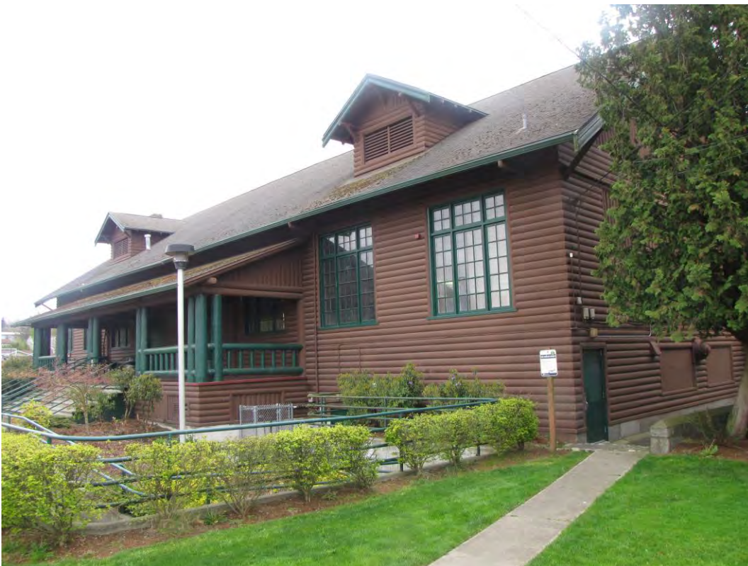
3 of 15 – Northwest corner of fieldhouse showing basement handicap access, No. 0003
