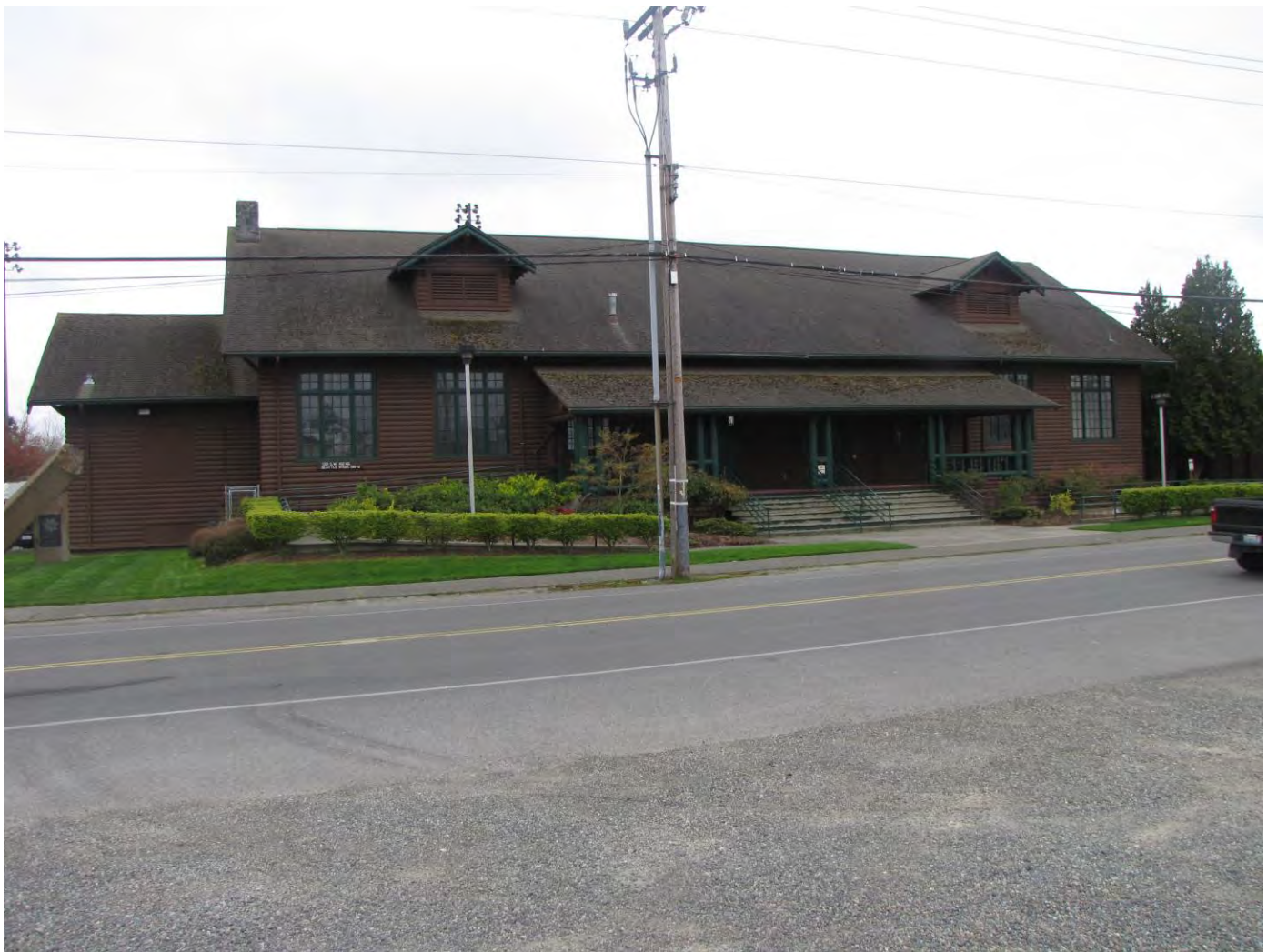
1 of 15 - Main façade/ north elevation of fieldhouse, No. 0001
