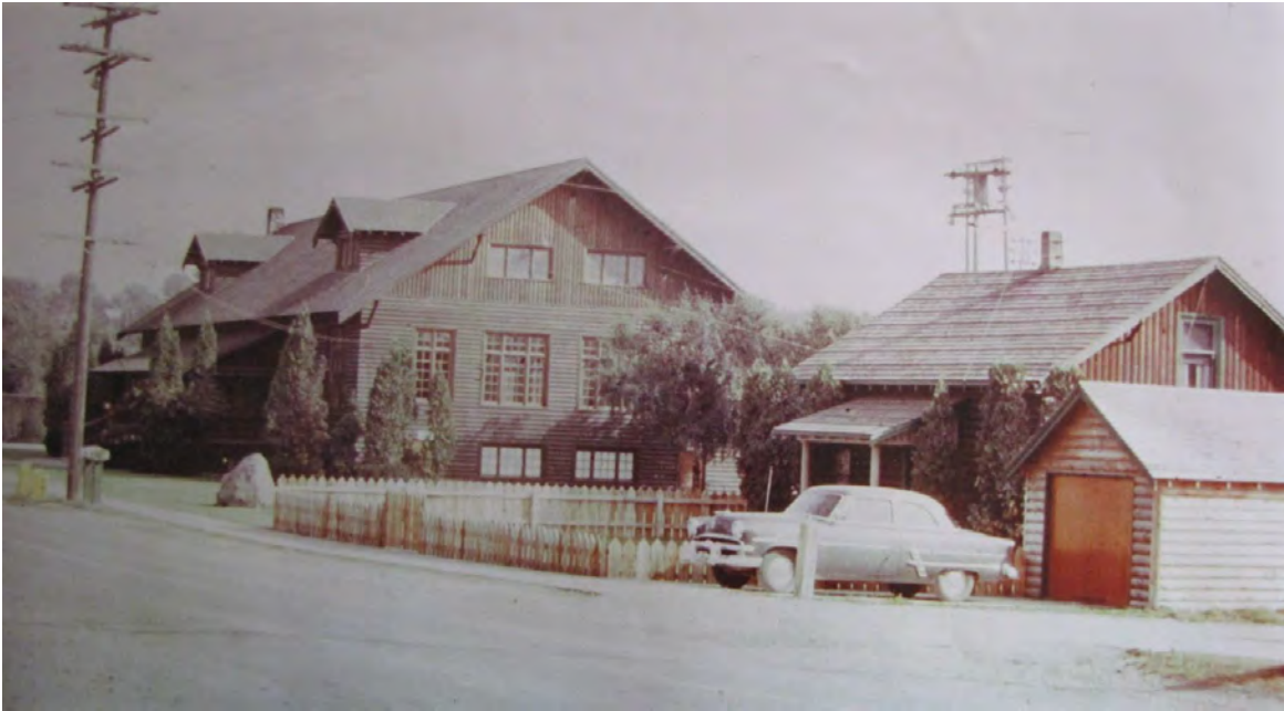
Right to Left: Garage, Caretakers Cottage and Fieldhouse – c. 1952
