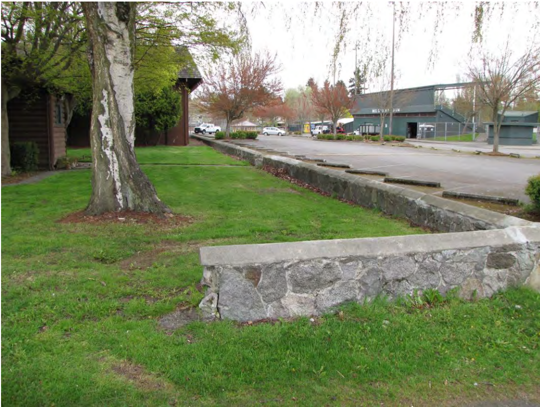
12 of 15 – Rock wall at rear of caretaker house, No. 0012
