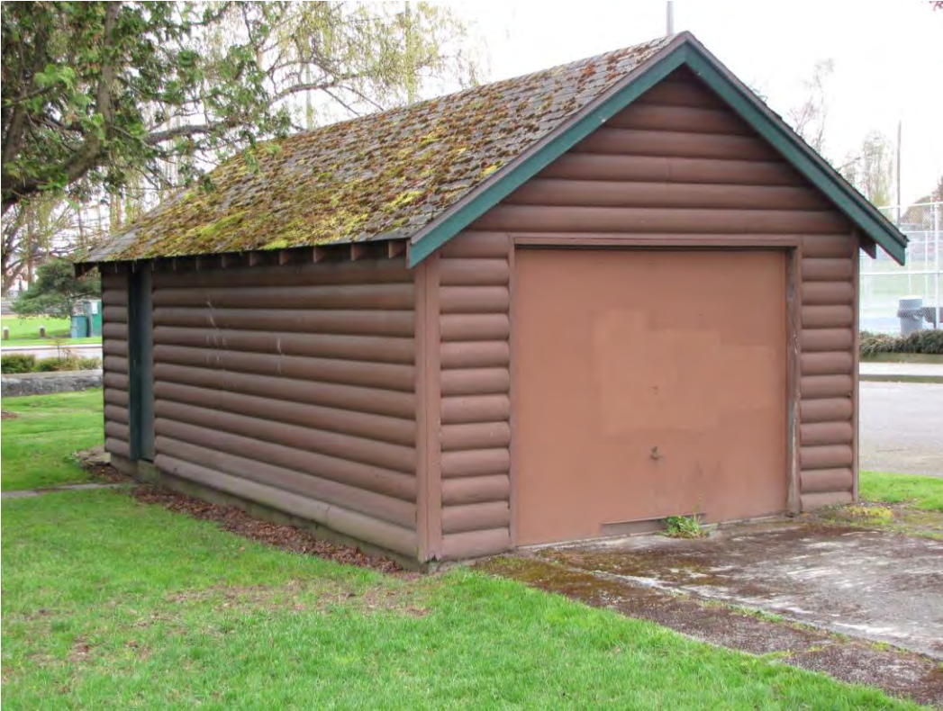
14 of 15 – Caretaker garage, No. 0014
