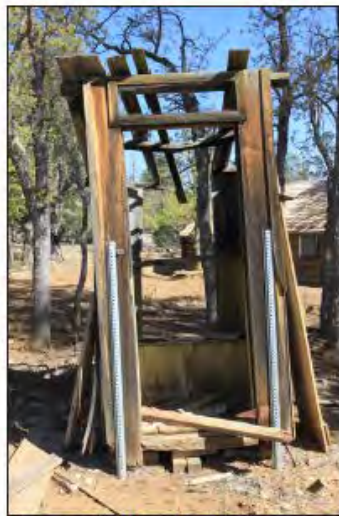
Figures 29-30. Above: East exterior before rehabilitation. Below: East exterior after.
