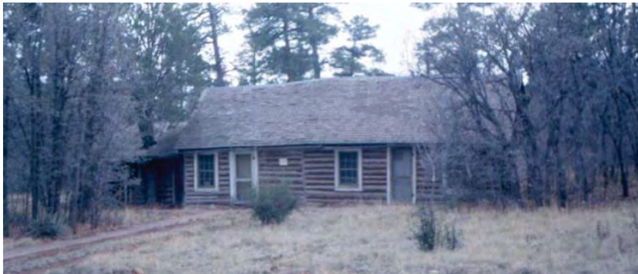
Cabin's New Roof during Mission 66, facing south. NPS photograph by N. Ritchie, 1966, WACA Archives.
