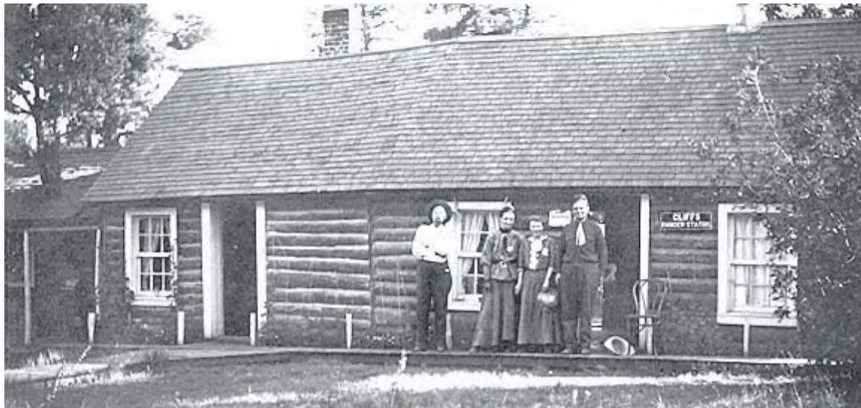
Cliffs Ranger Station, facing south-southwest. Note sign at right. Photograph c.1915, NAU Cline Library.
