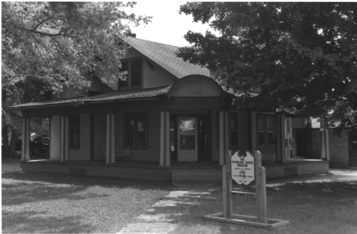
Water Street Historic District Clifton, Wayne Co., TN #9 of 10
