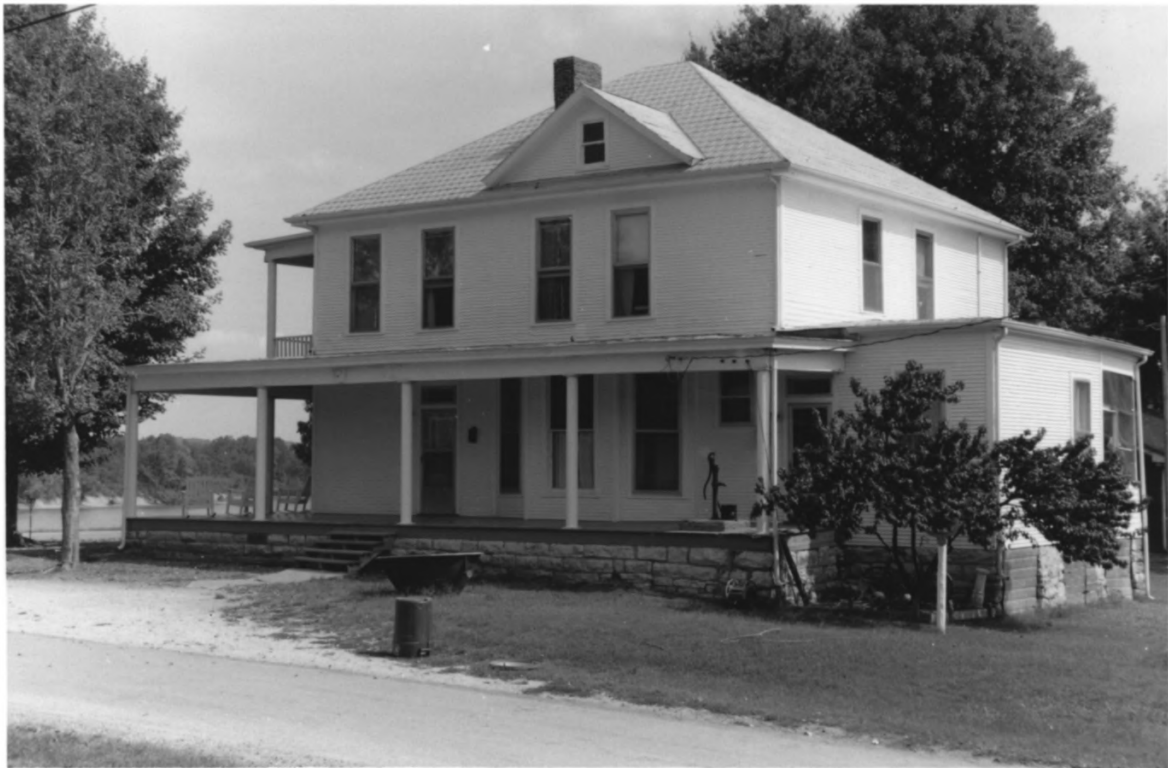
Water Street Historic District Clifton, Wayne Co., TN #2 of 10
