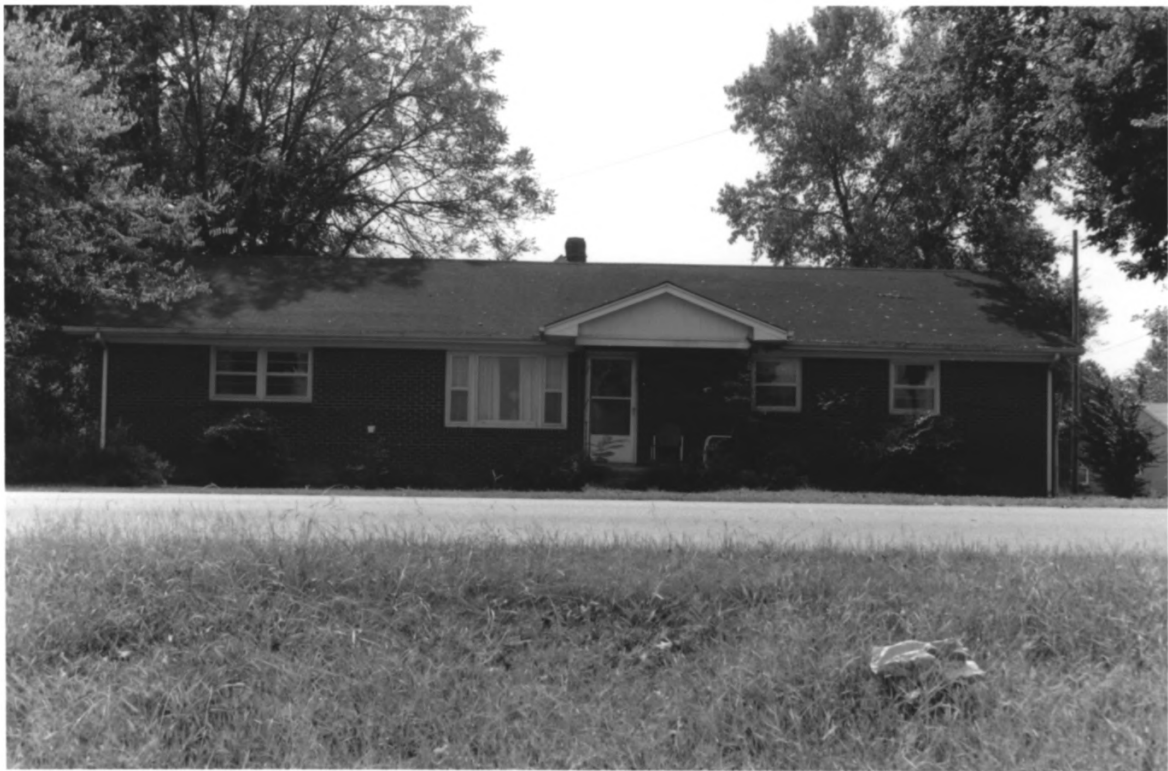
Water Street Historic District Clifton, Wayne Co., TN #4 of 10
