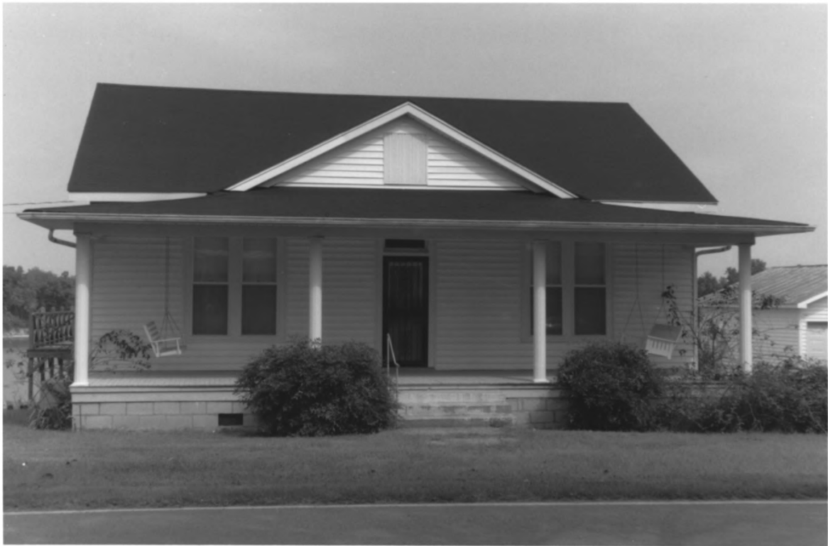
Water Street Historic District Clifton, Wayne Co., TN #6 of 10
