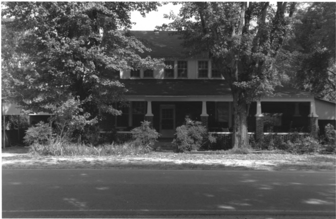
Water Street Historic District Clifton, Wayne Co., TN #10 of 10
