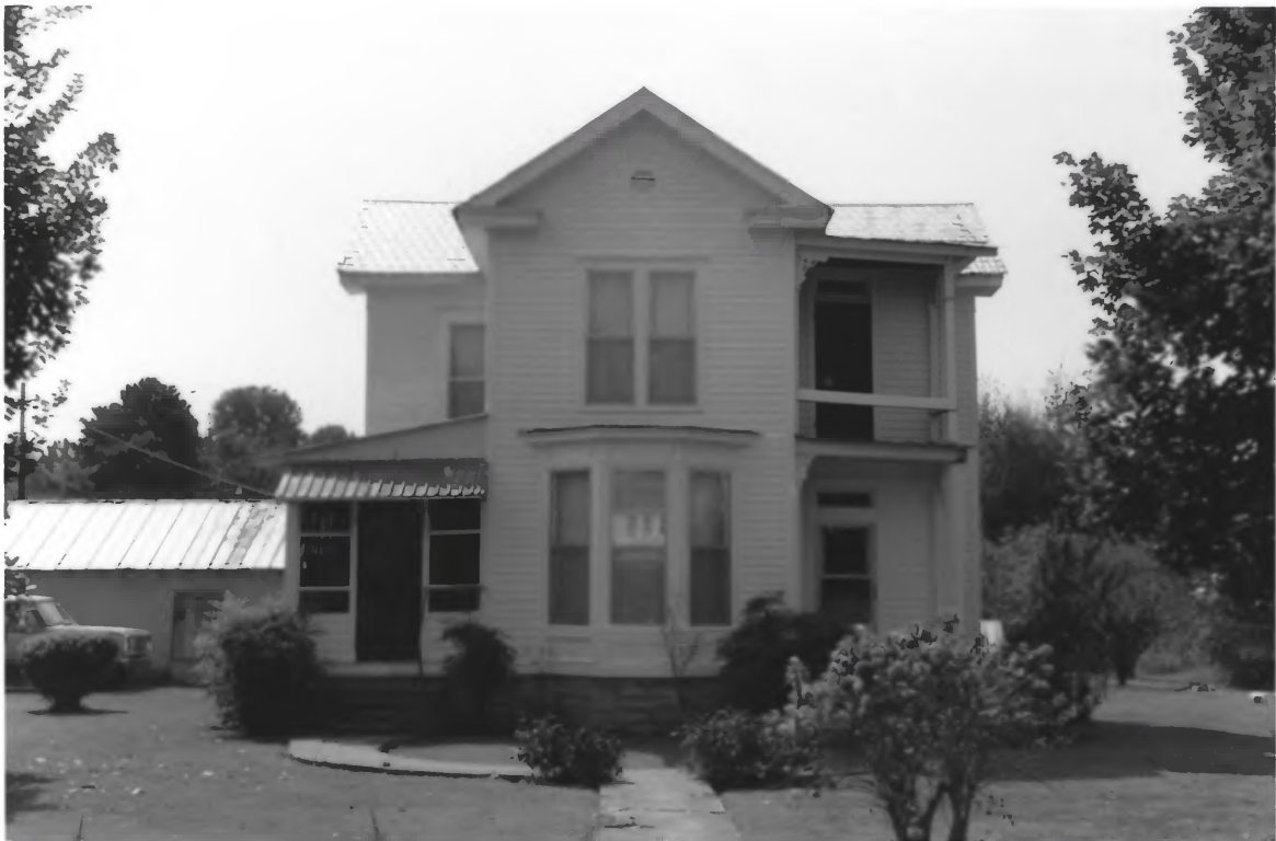
Water Street Historic District Clifton, Wayne Co., TN # 7 of 10
