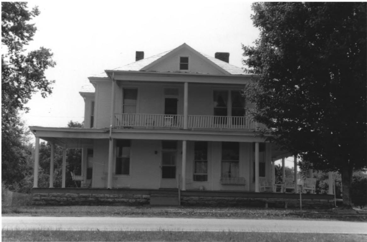
Water Street Historic District Clifton, Wayne Co., TN #1 of 10
