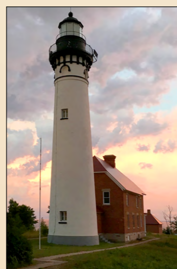
Powered now by solar energy, the 1874 Au Sable Light Station still warns mariners about the dangerous Au Sable reef.
