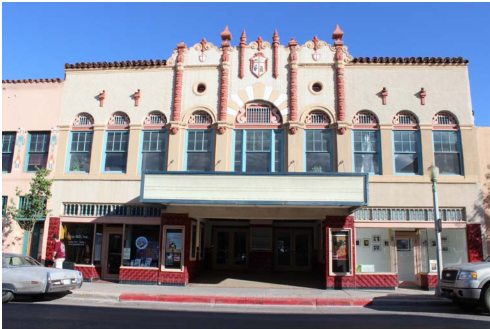
5 of 15. El Morro Theater, 205-207, West Coal Avenue, photographer facing southwest.
