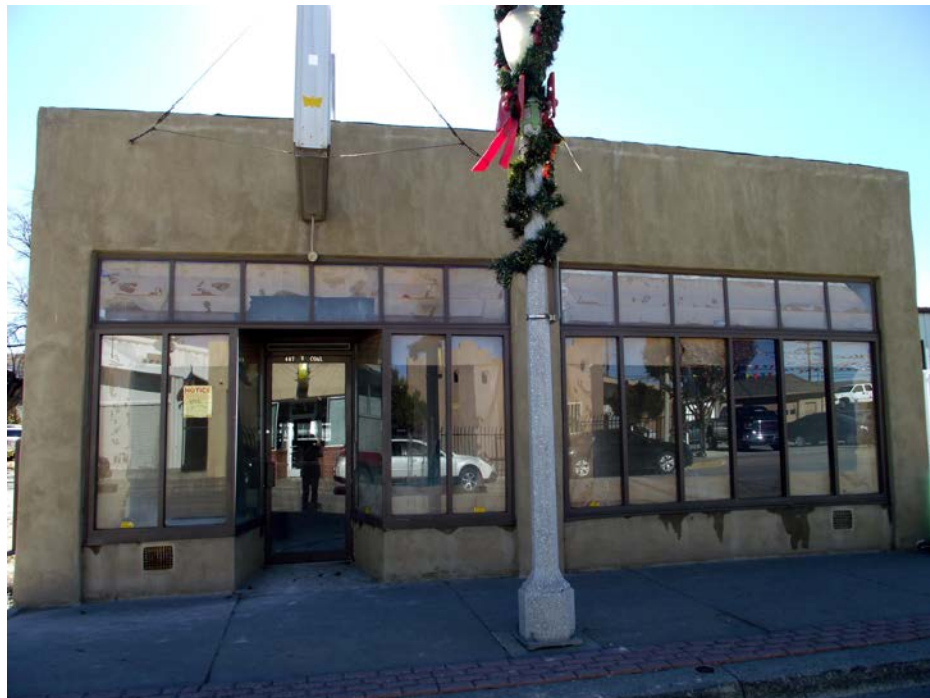
10 of 15. Commercial Building, 407 West Coal Avenue, photographer facing southeast.
