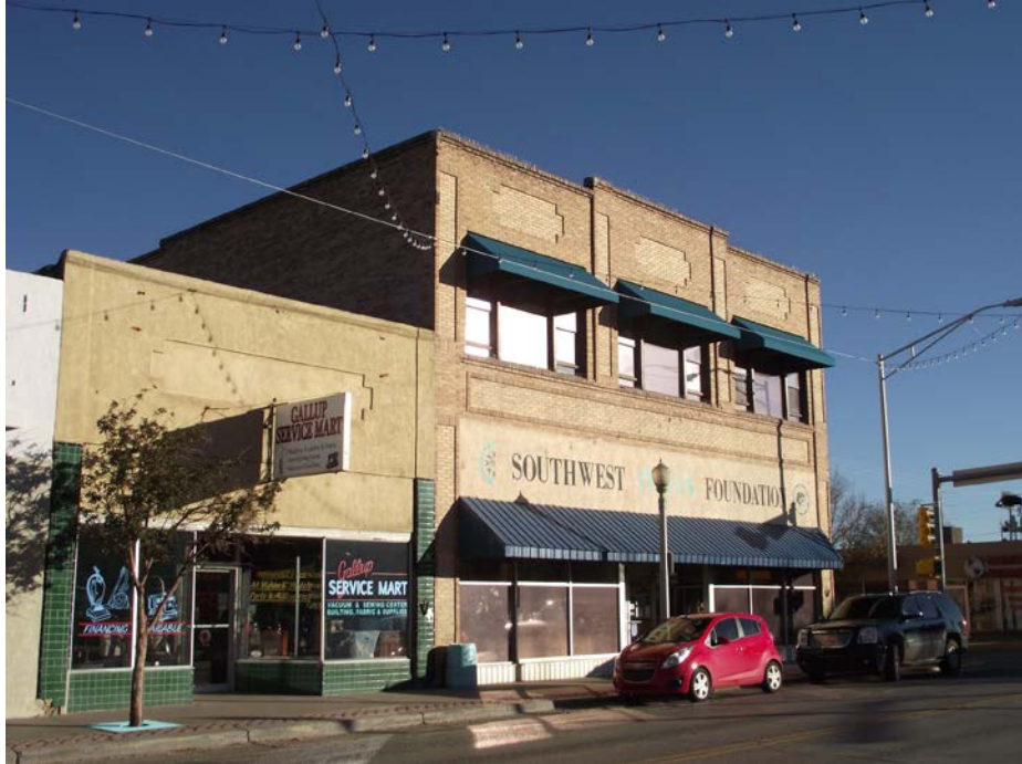
1 of 15. Montgomery Ward Building 100 and 104 West Coal Avenue, photographer facing northeast.
