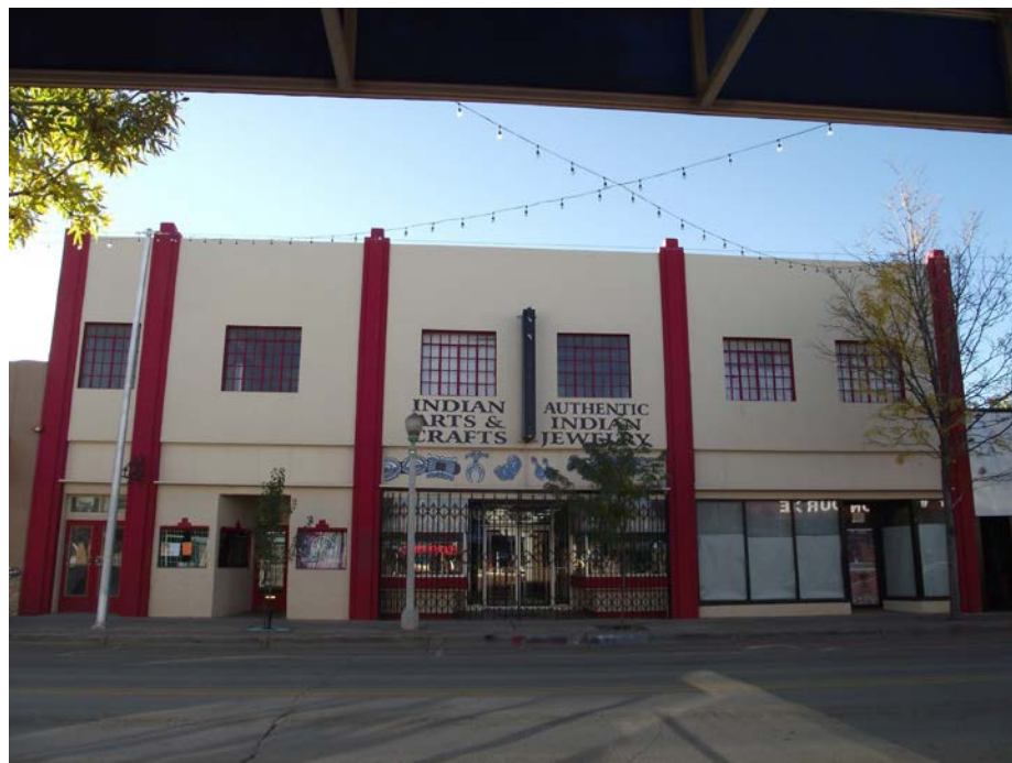
2 of 15. Allison Building, 115-119 West Coal Avenue, photographer facing south.
