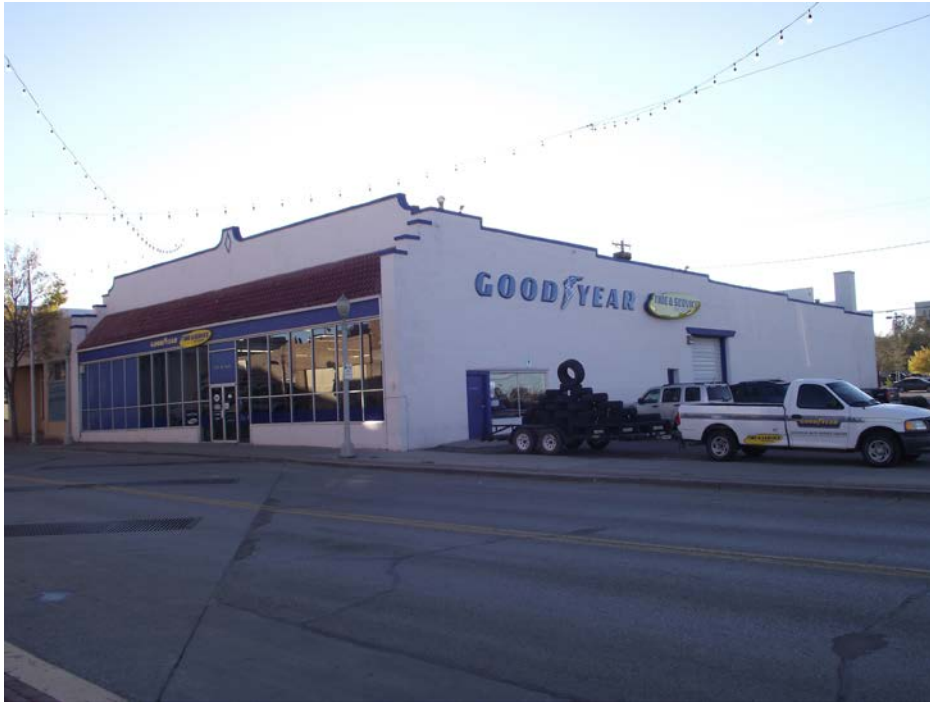
9 of 15. Rico Motors Company Building, 307 West Coal Avenue, photographer facing southeast.
