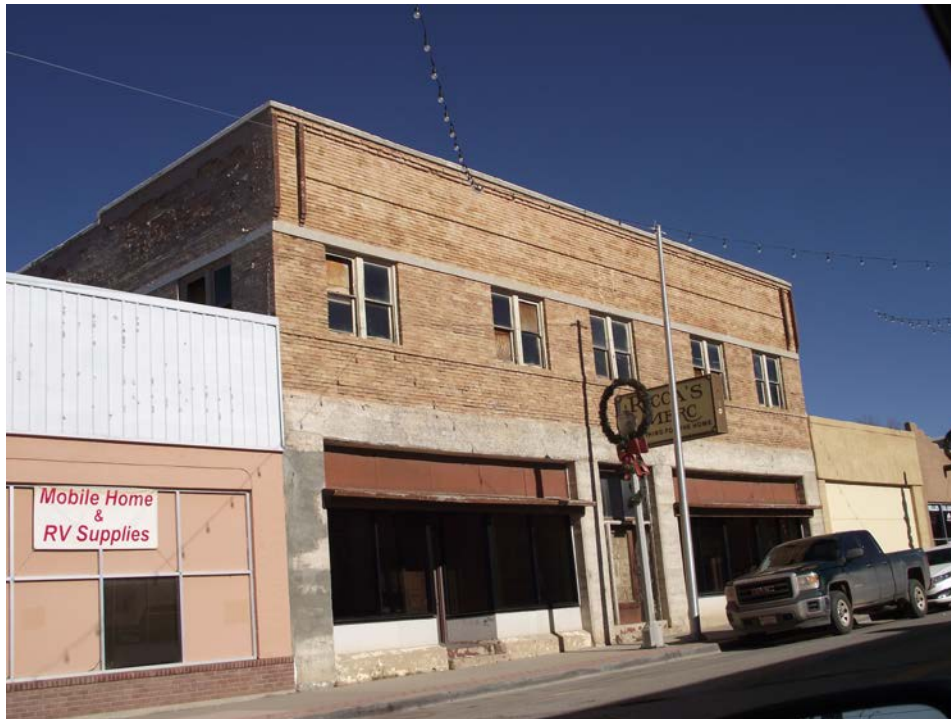
7 of 15. Grand Hotel (Ricca Mercantile), 304-306 West Coal Avenue, photographer facing northwest.
