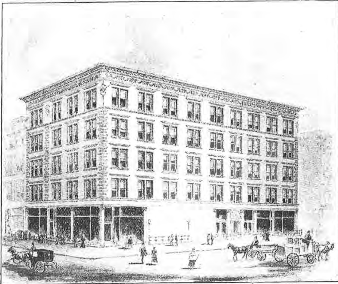
No. 24 JEFFERSON THE TAMA BUILDING.
