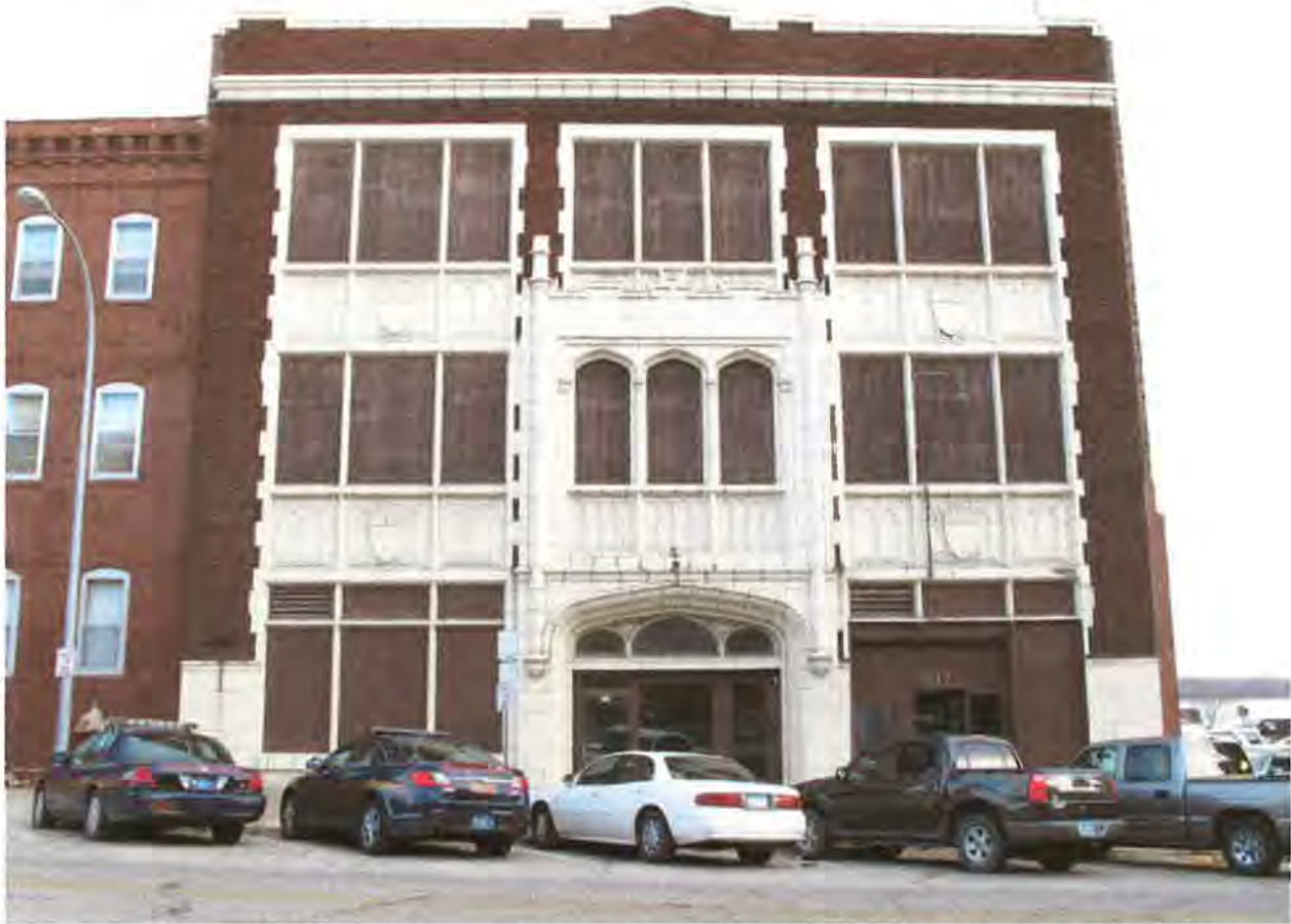
Figure 24. Current view of terra cotta on Remy Building (McCarley, November 15, 2012).
