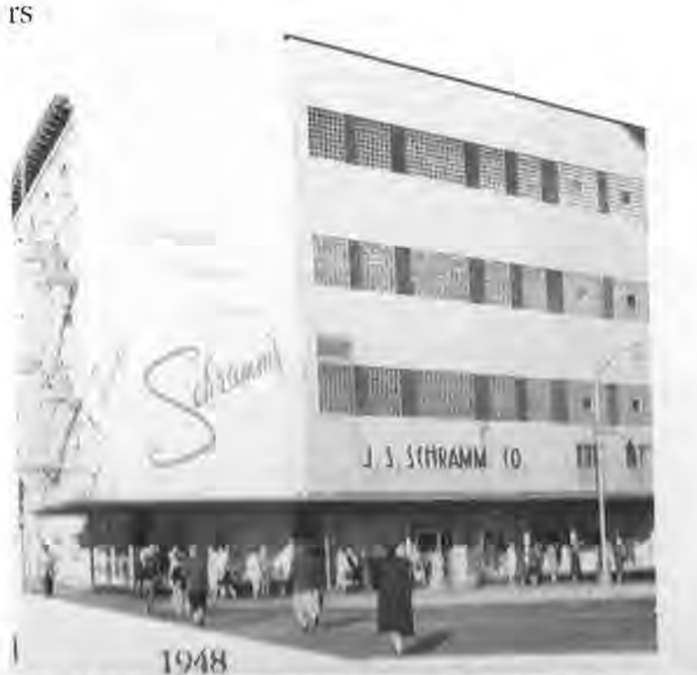
Figure 37. J.S. Schramm after completion of 1947 remodel (Mertens 1996: 99).
