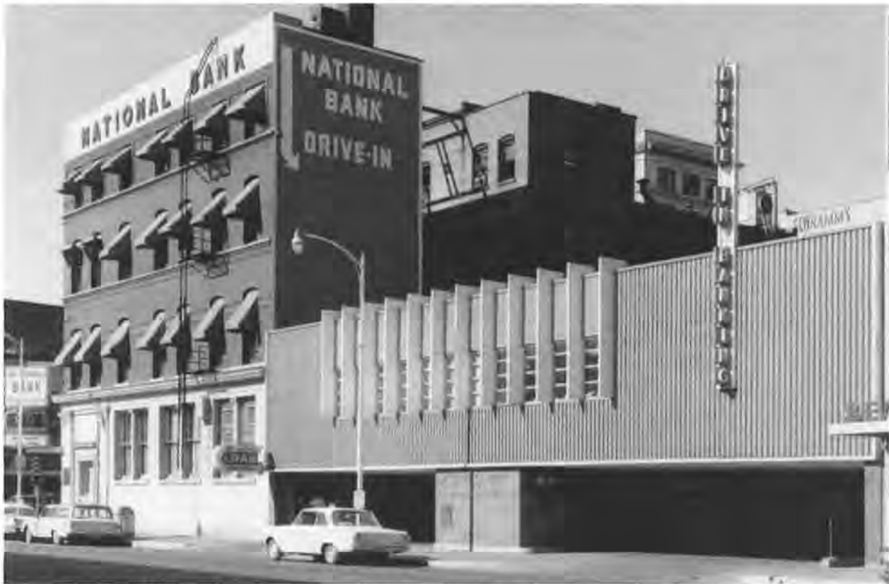
Figure 46. National Bank and new 1958 section in 1970s (Downtown Partners collection).
