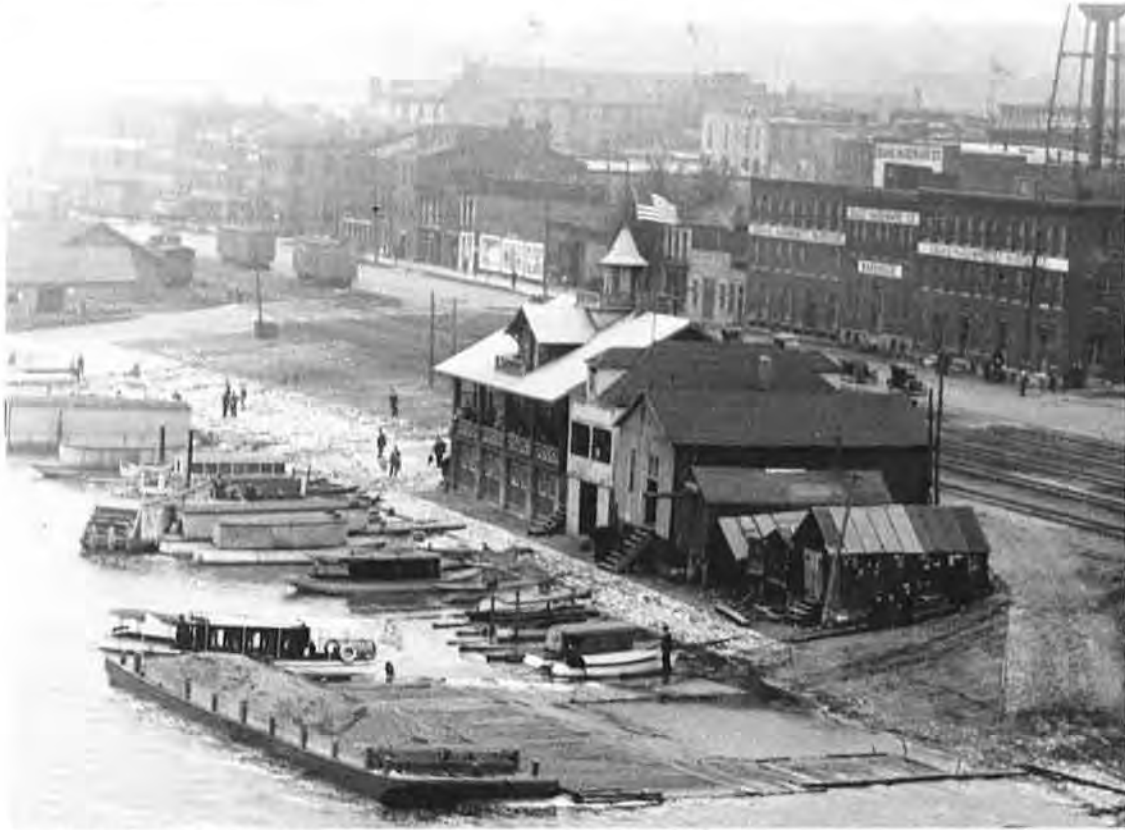
Figure 15. Buildings on levee and along 200-400 blocks of N. Front Street in 1910s (DMCHS collection).
