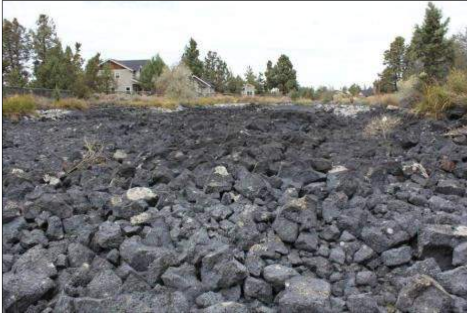
SEGMENT 4: At this location, the canal has two cut sides and a shallow, rocky bed. The loose rock was likely blasted. Because there is no embankment here in which to make use of it, the rock was left in the canal bed. Photographer looking north.
