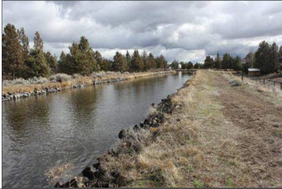
Segment 3: Segment is straight and deep with thick riprap on both sides. At-grade cut side on north side of canal. Sloping embankment and agricultural fencing on south side. Tax lots run to center of canal. Photographer looking east.
