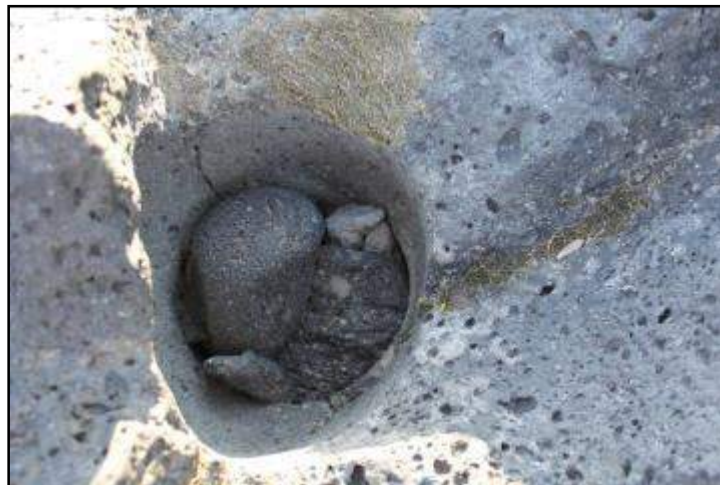
Photo of sediment and stones deposited in a drilled and blasted rock in the canal bed near the Old Deschutes Road Bridge in the Historic District. Many drilled and fractured rocks in the district represent the 1904 labor.
