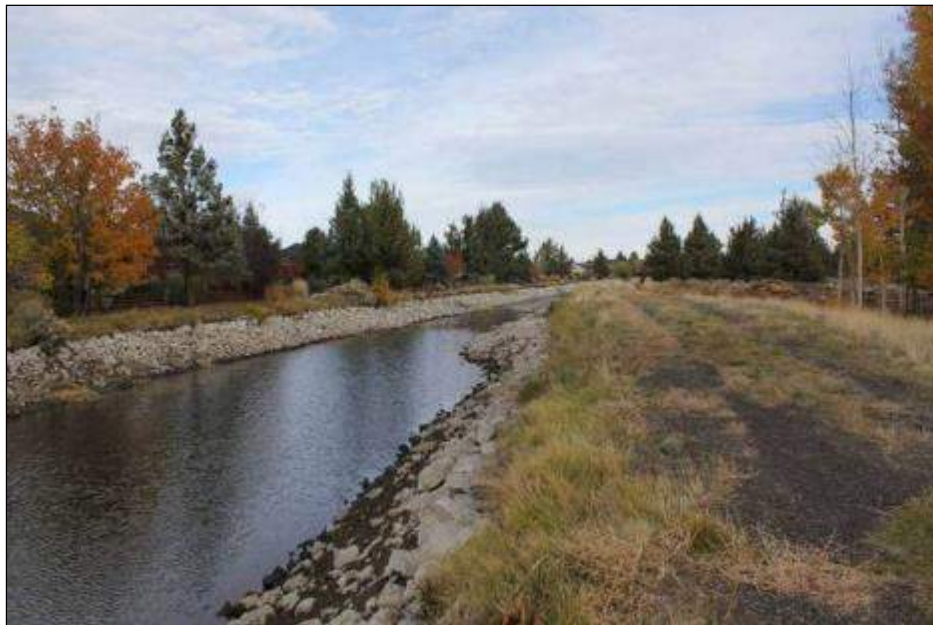
Segment 1: Canal bed with standing water, wide embankment on right. Photographer looking north.
