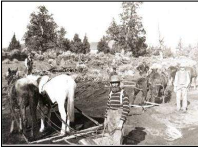
Using horse-drawn Fresno scrapers Photograph: DeschutesCounty Historical Society
