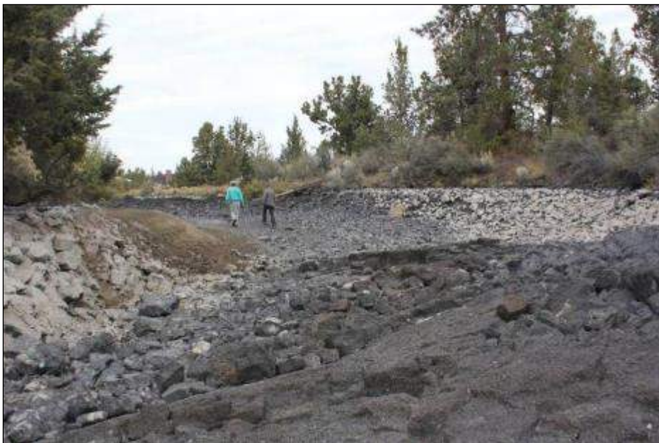
SEGMENT 4: Undulating bed, lava flows and loose rock, no berms. Photographer looking north.
