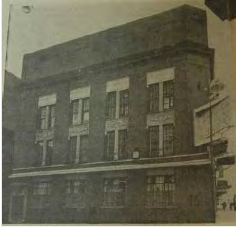
1962, pre-renovation. From Goloversic, “‘Simple’ Project At Lagonda Bank Is Completed As Major Renovation”
