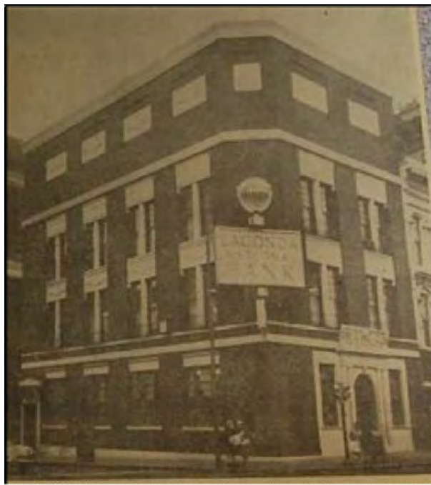
1963, post renovation. From Goloversic, “‘Simple’ Project At Lagonda Bank Is Completed As Major Renovation”
