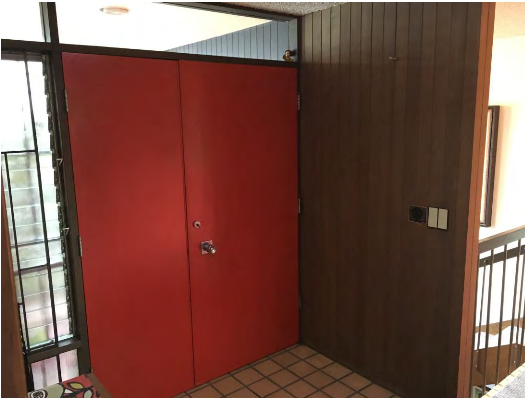
11 of 23 - Detail of main entry doors.
