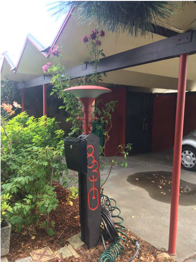
2 of 23 – Detail of entry light post and house number mail box.
