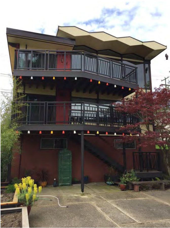
6 of 23 - Rear of house / East façade.
