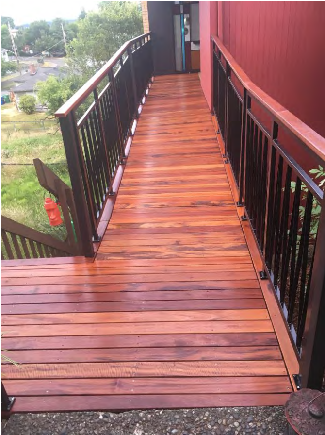
4 of 23 – Detail of entry bridge.
