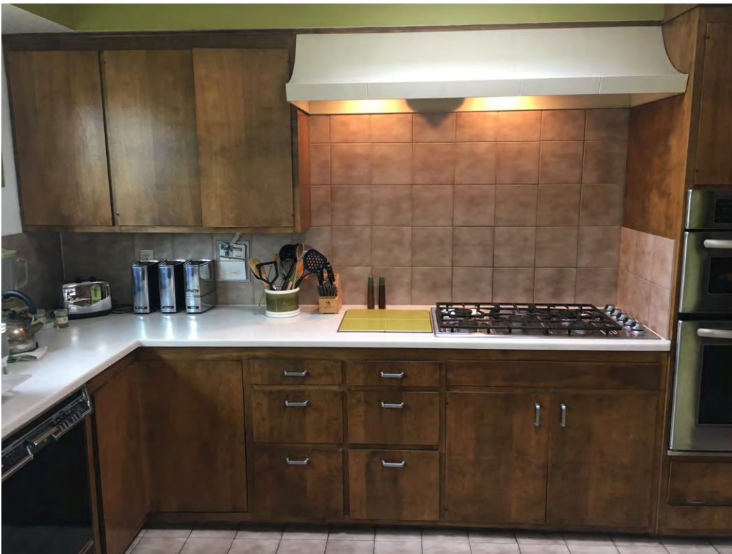
15 of 23 – Detail of kitchen cabinets and range area.
