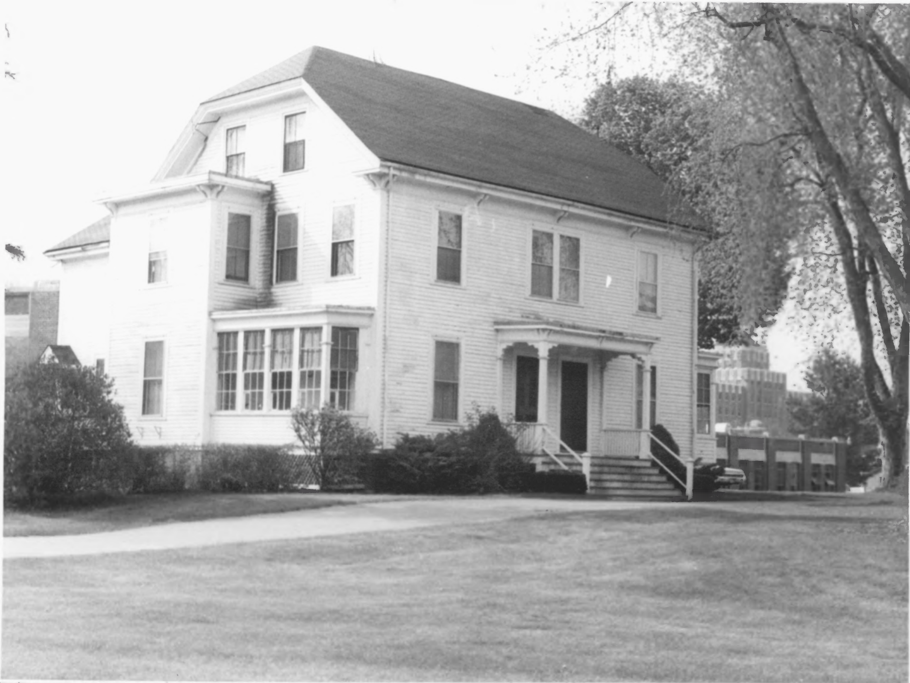
Engineer and Band Master's House (Building No. 68), National Home for Disabled Volunteer Soldiers, Togus, Maine. NPS Photo 1973
