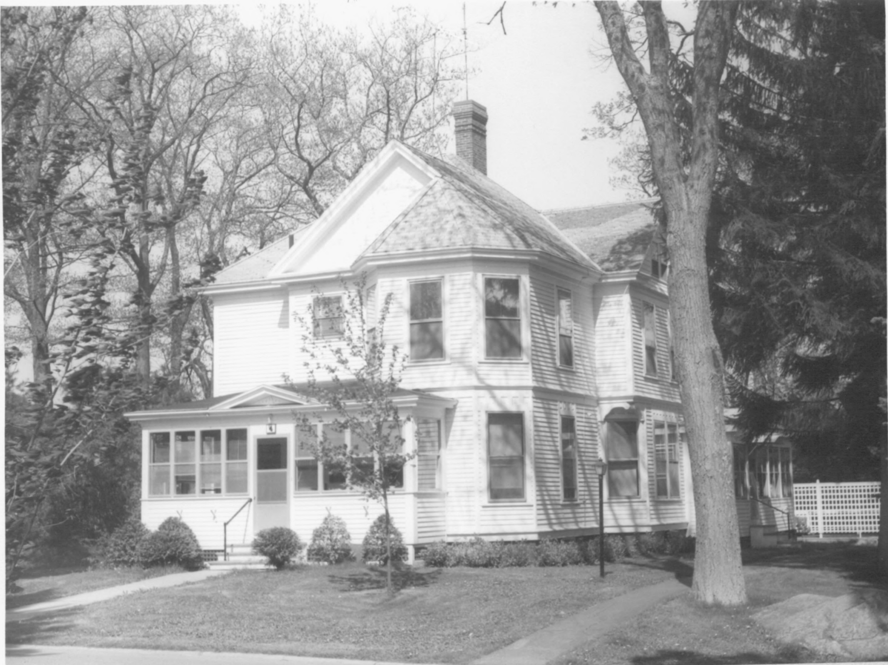
Commissary of Subsistences House ( Building No. 4), National Home for Disabled Volunteer Soldiers, Togus, Maine. NPS Photo 1973
