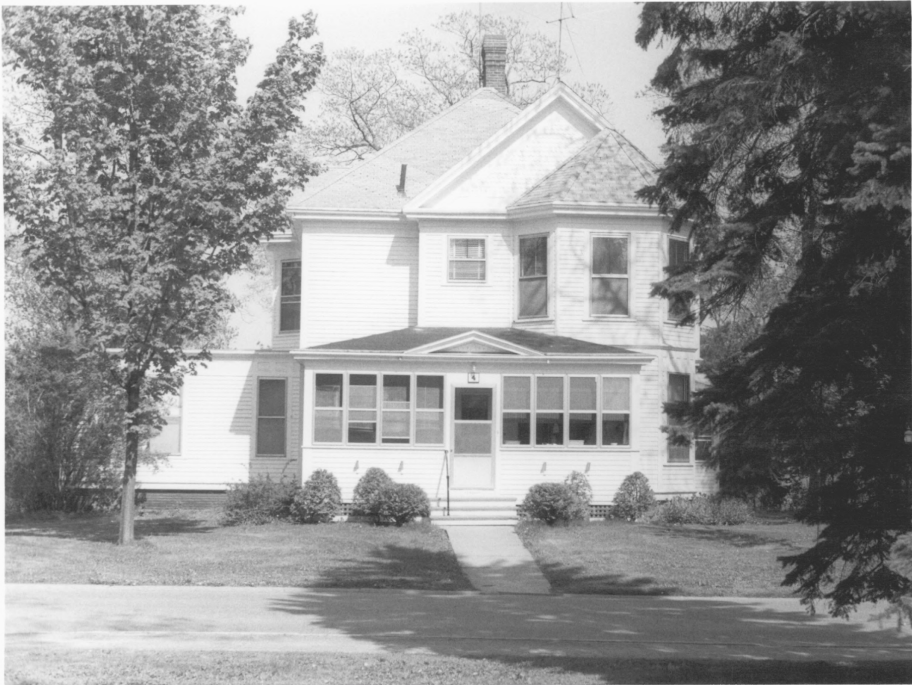
Commissary of Subsistences House (Building No. 4), National Home for Disabled Volunteer Soldiers, Togus, Maine. NPS Photo 1973
