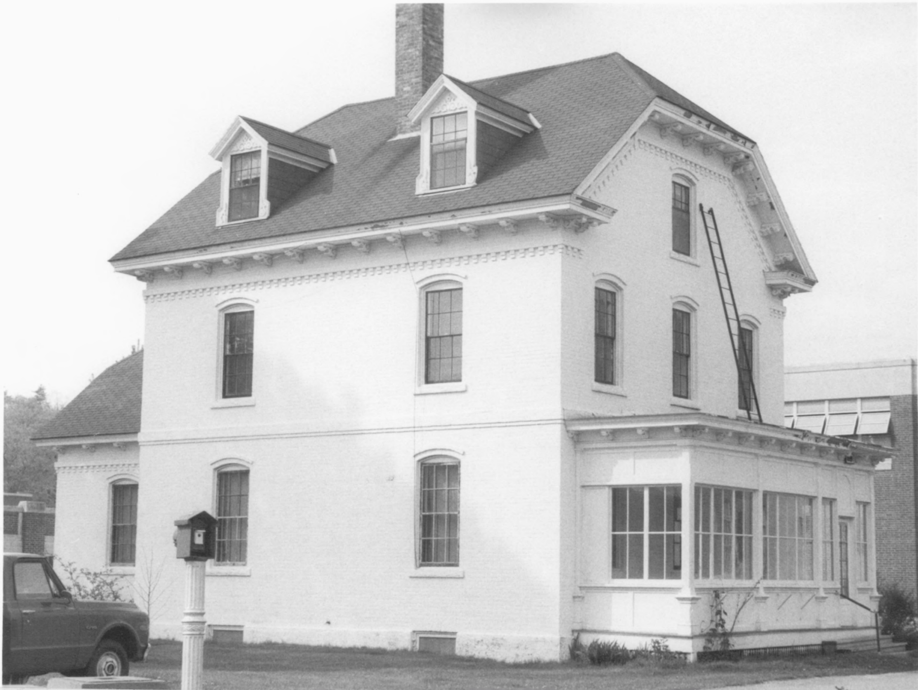
Surgeon's House (Building No. 69), National Home for Disabled Volunteer Soldiers, Togus, Maine.
