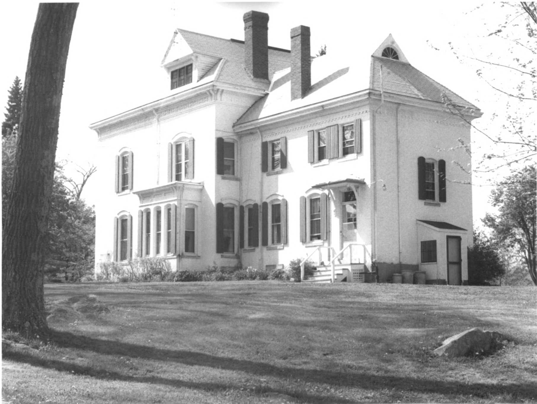
Treasurer's House (Building No. 3), National Home for Disabled Volunteer Soldiers, Togus Maine.
