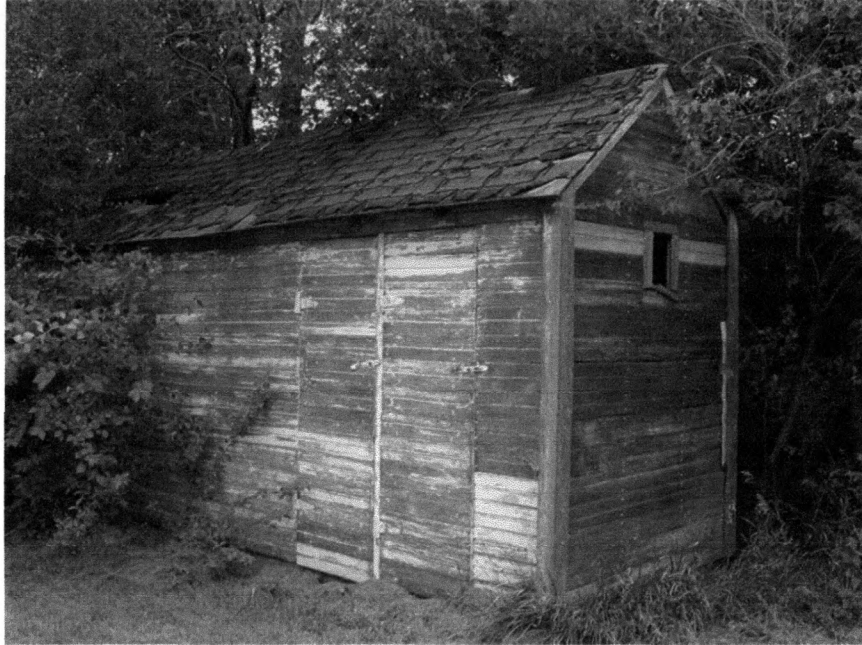
Figure 11 The outbuilding's two doors lead into the single-chamber privy on the right and a storage area on the left. Tallgrass Historians L.C.
