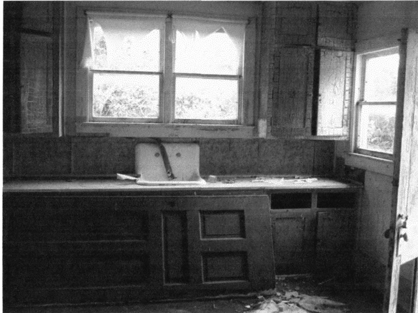
Figure 10 The kitchen, looking slightly northeast. Tallgrass Historians L.C.
