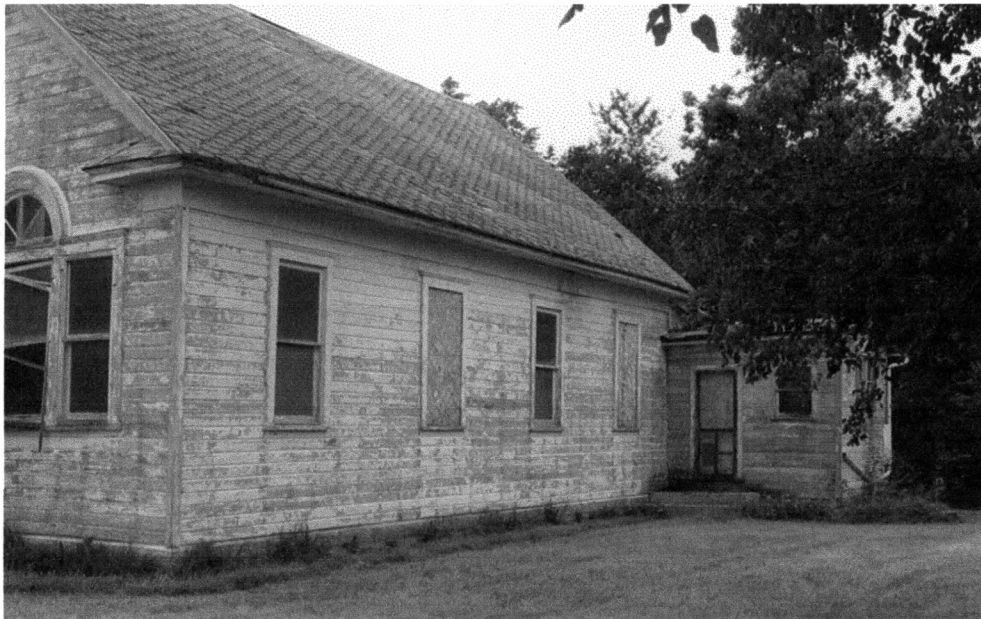
Figure 2 East side and rear kitchen wing. Tallgrass Historians L.C.
