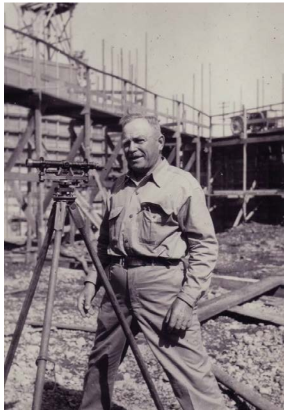
Einar Fieldstad during construction of St. Aloysius School in Spokane. Image courtesy of Tedd Fieldstad.
