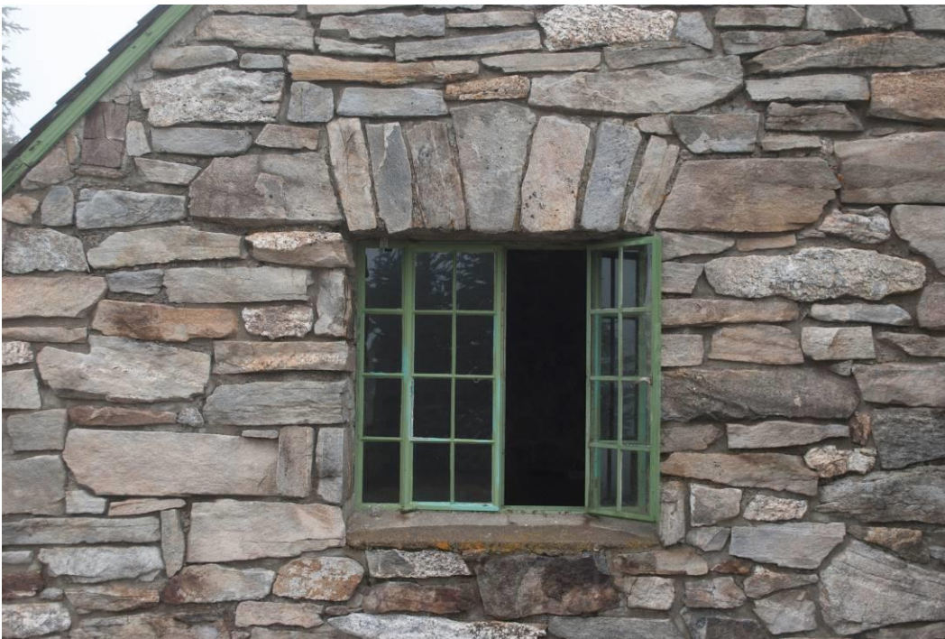
Photo 7: Detail view of typical window (south window at main floor shown).
