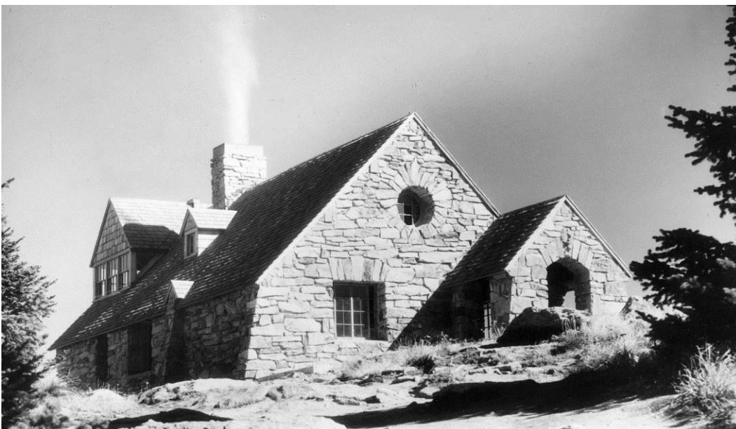
Vista House, view to northeast, 1937. Image courtesy of WSPRC.
