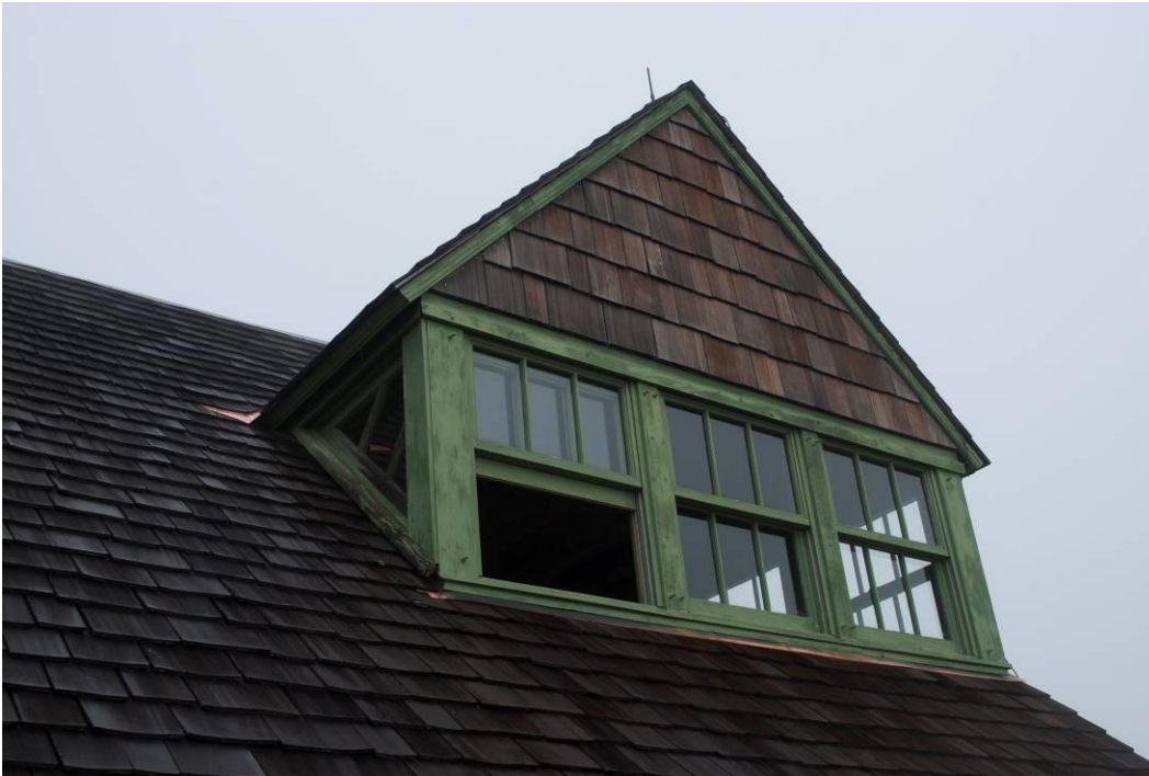
Photo 6: Detail view of fire lookout, east side.
