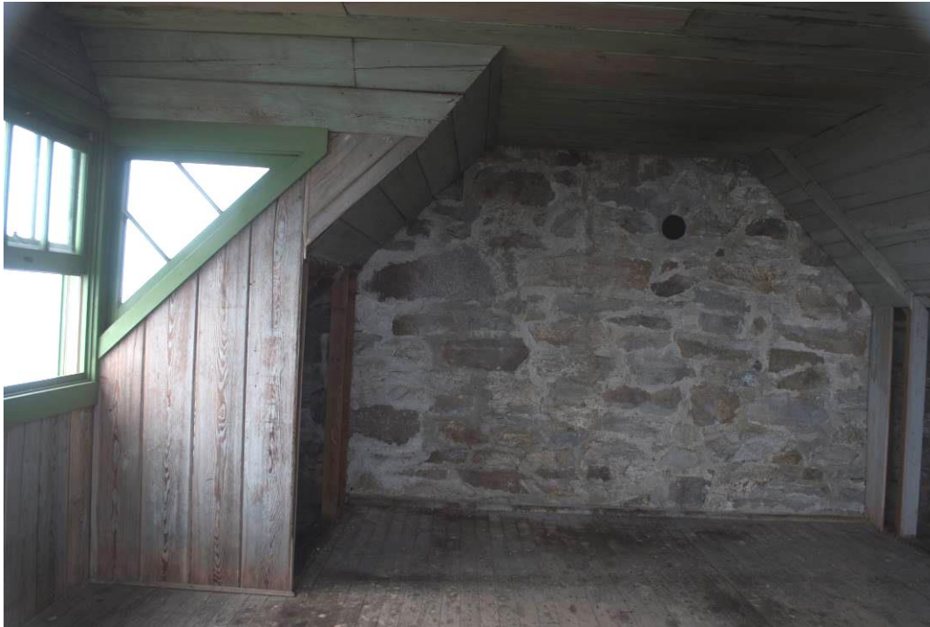
Photo 12: Interior view (to south) in fire lookout.
