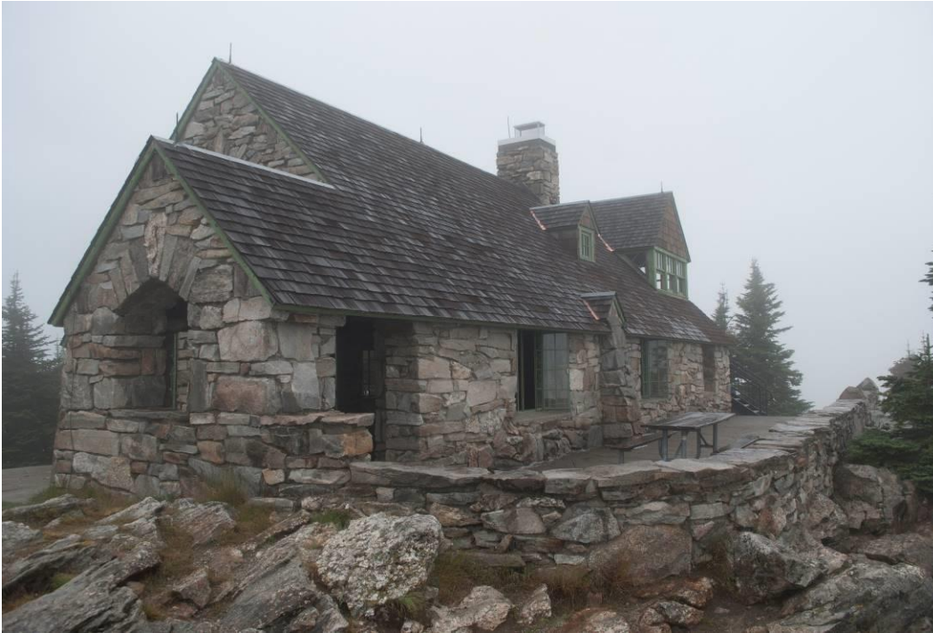
Photo 2: View to northwest.
