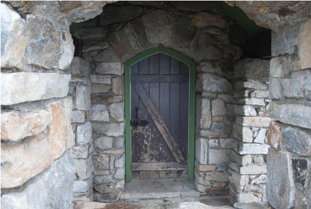
Photo 8: Detail view of front door (south end).
