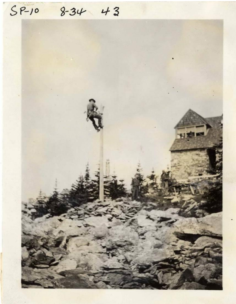
Vista House, northwest end visible. August 1934. WSPRC Image 78-SP10-43.
