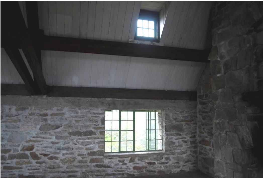
Photo 11: Detail view of interior windows at northwest corner of gathering room.
