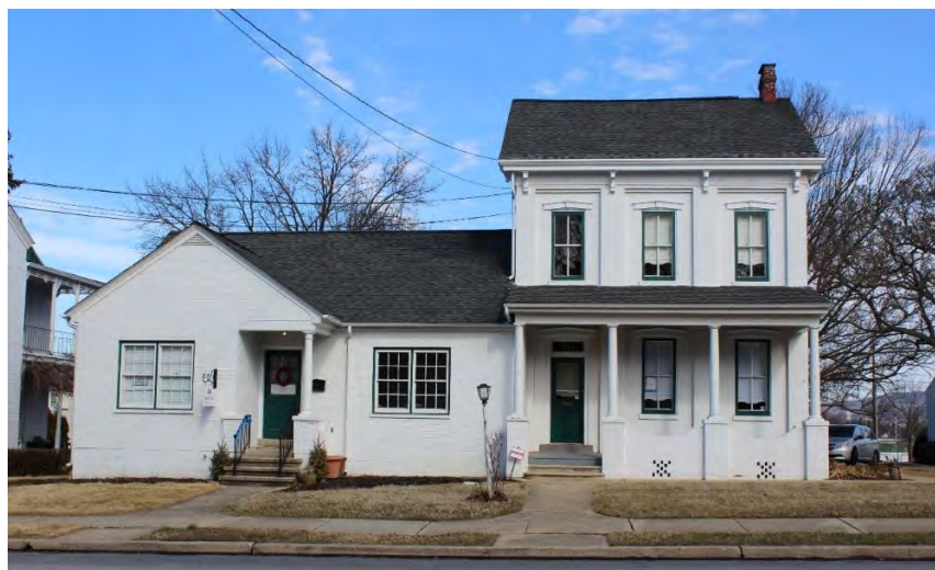
Photo 4: The Philadelphia Avenue-facing elevation, featuring the 1884 original home with the 1950 doctor's practice addition.
