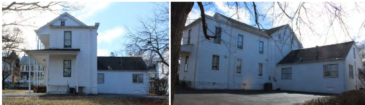
Photo 9 (left) and Photo 10: The north elevation includes the c.1900 addition, the upper gable end of the original service ell and the rear of the 1950 addition. The view looking southeast shows the relationship of the 1950 addition to the front of the original house.
