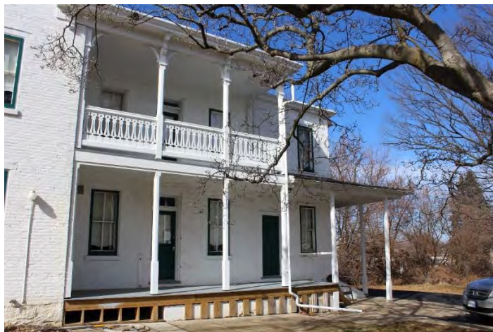
Photo 8: The two-story side porch was restored in 2017.
