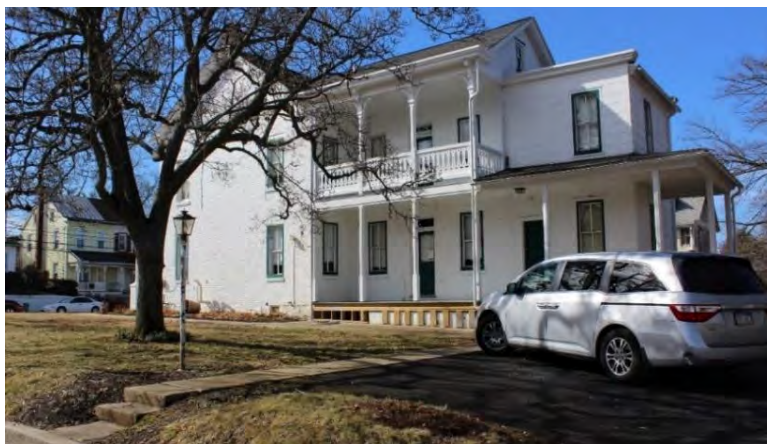
Photo 7: The east elevation includes the original house with the two-story c.1900 frame addition at the rear.
