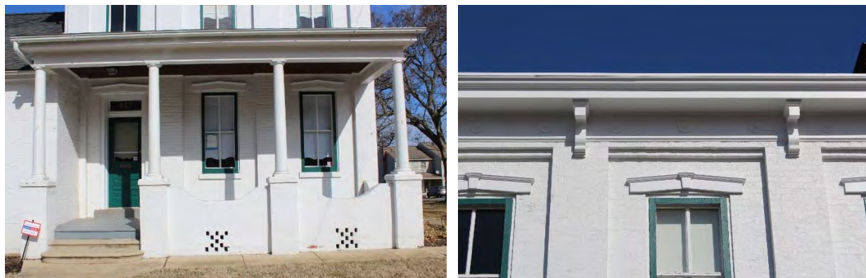
Photo 5 & 6: The front porch, 2-over-2 sash windows, front door and window hoods, and door frame are all original. The front door and transom glass date to the 2017 restoration, as do the cornice, brackets and frieze.
