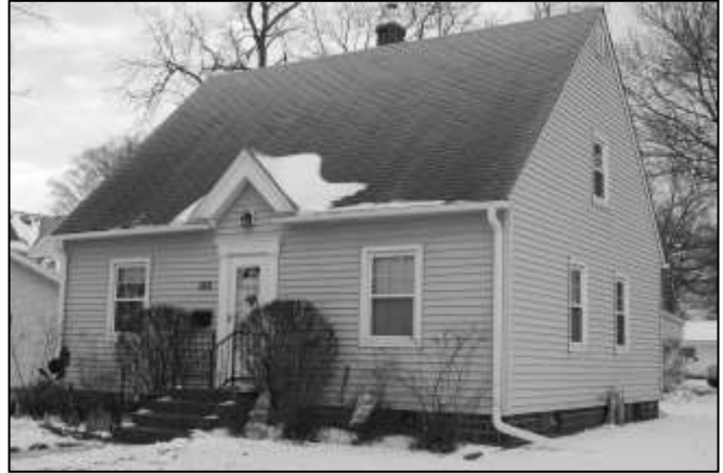
Wilbert and Blanche Oberheu House, 108 3 rd Ave SW, looking northwest (Svendsen Tyler, photographer, 2014)
