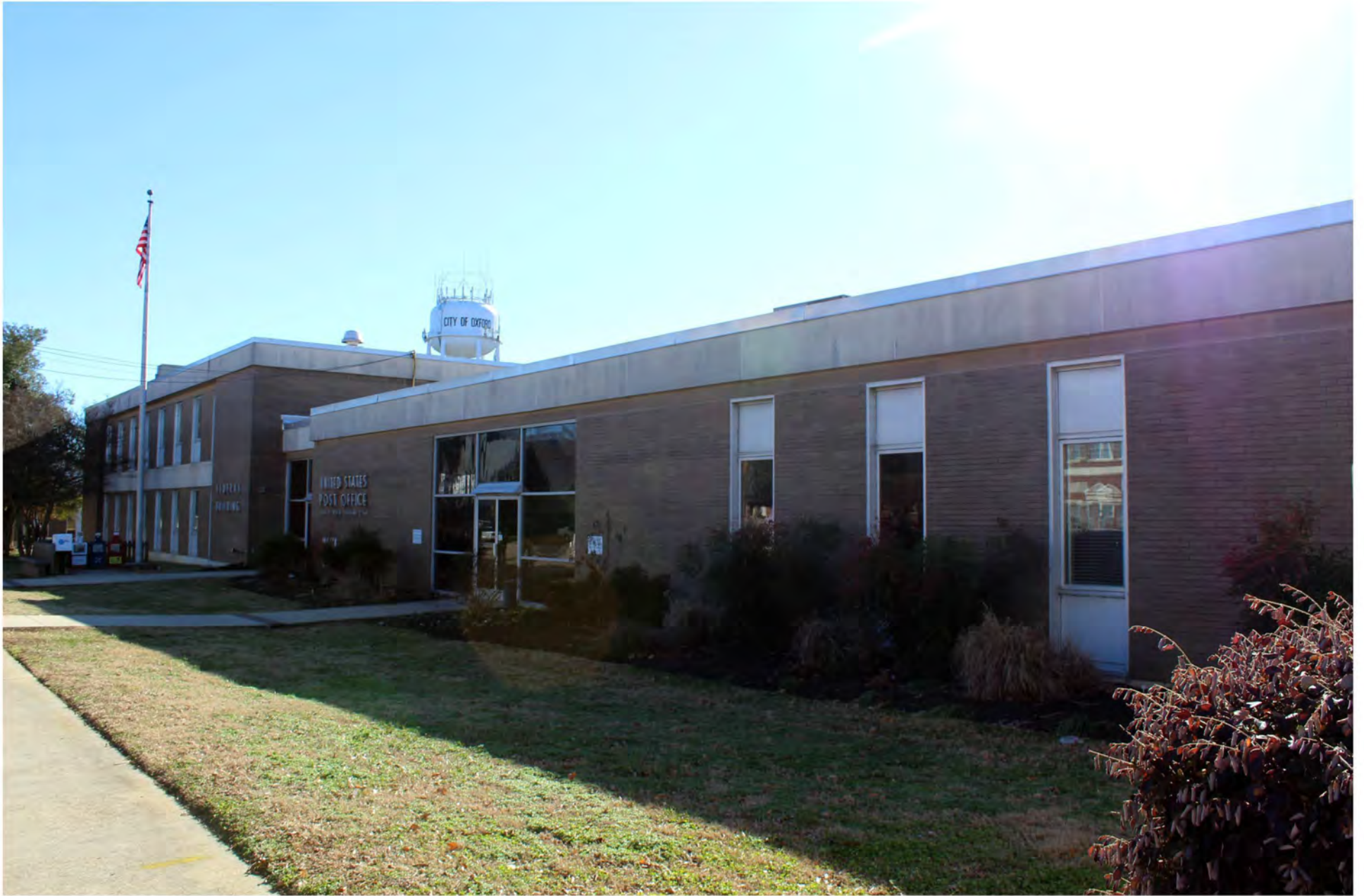
Photo 27 of 27: 144 Main Street, Oxford Historic District, facing southwest.
